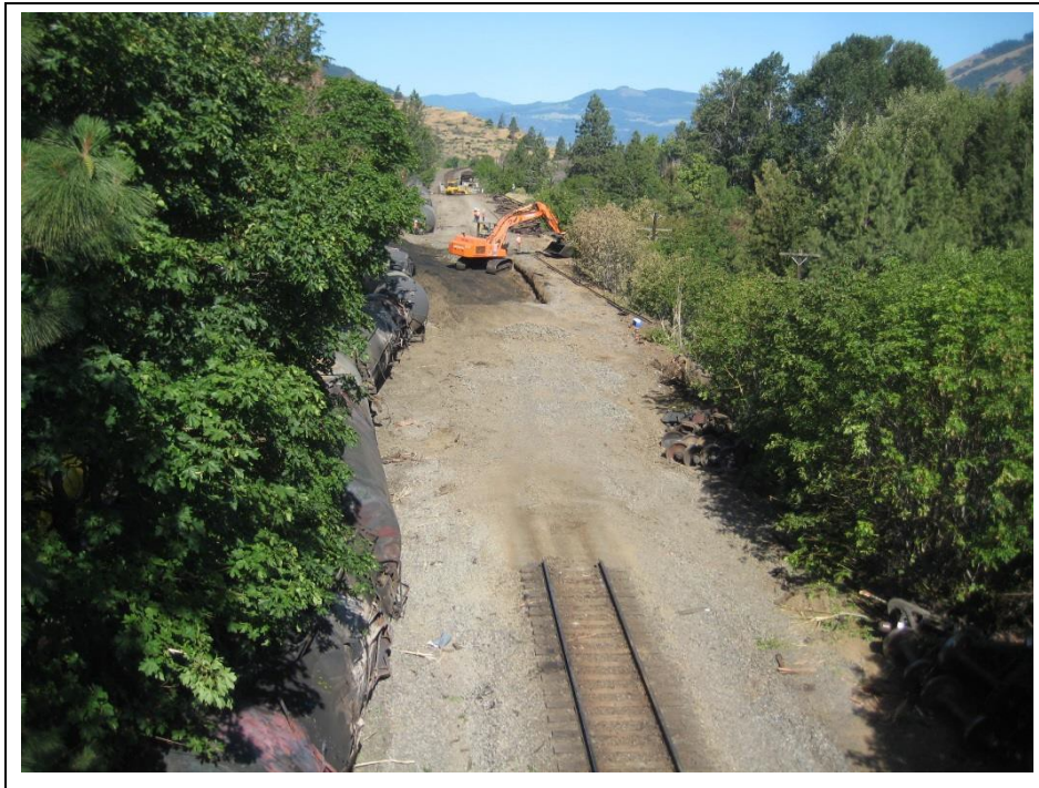
Photograph 7. Excavation and repair of UPRR line after train cars were moved off to the side. Photograph taken on June 5, 2016. Aspect: west.
