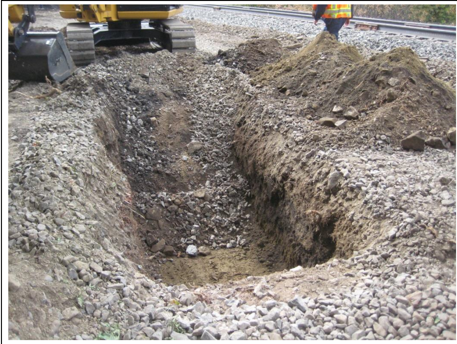
Photograph 3. Initial potholing at eastern end of excavation area conducted on June 9, 2016. Native soils were visible at the base of excavation. Aspect: west.
