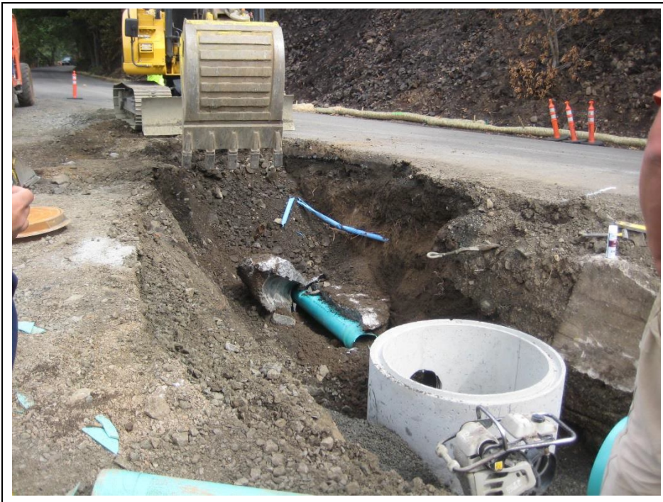
Photograph 10. Overview of open excavation, replacement of sewer line, and installation of new manway. Aspect: southwest.
