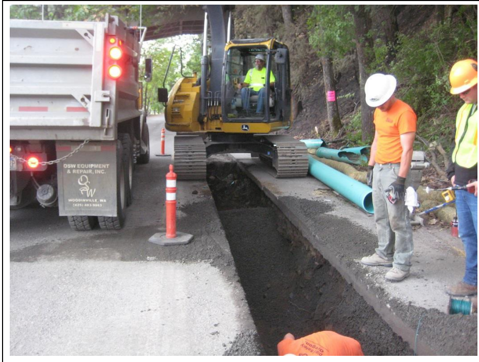
Photograph 11. Overview of trenching within Rock Creek Road to replace the sewer line to the WWTP. Aspect: east.
