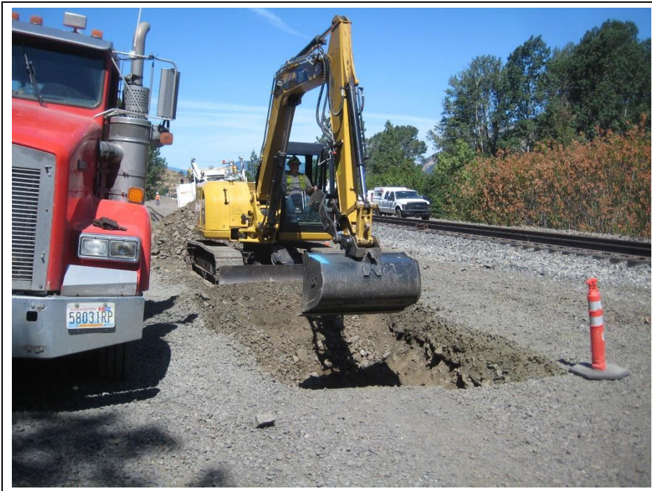
Photograph 5. Confirmatory sampling during initial remediation indicated that additional excavation was needed to remove contamination in a small area within the remediation footprint. Follow-up excavation was conducted on June 22, 2016. Aspect: west.
