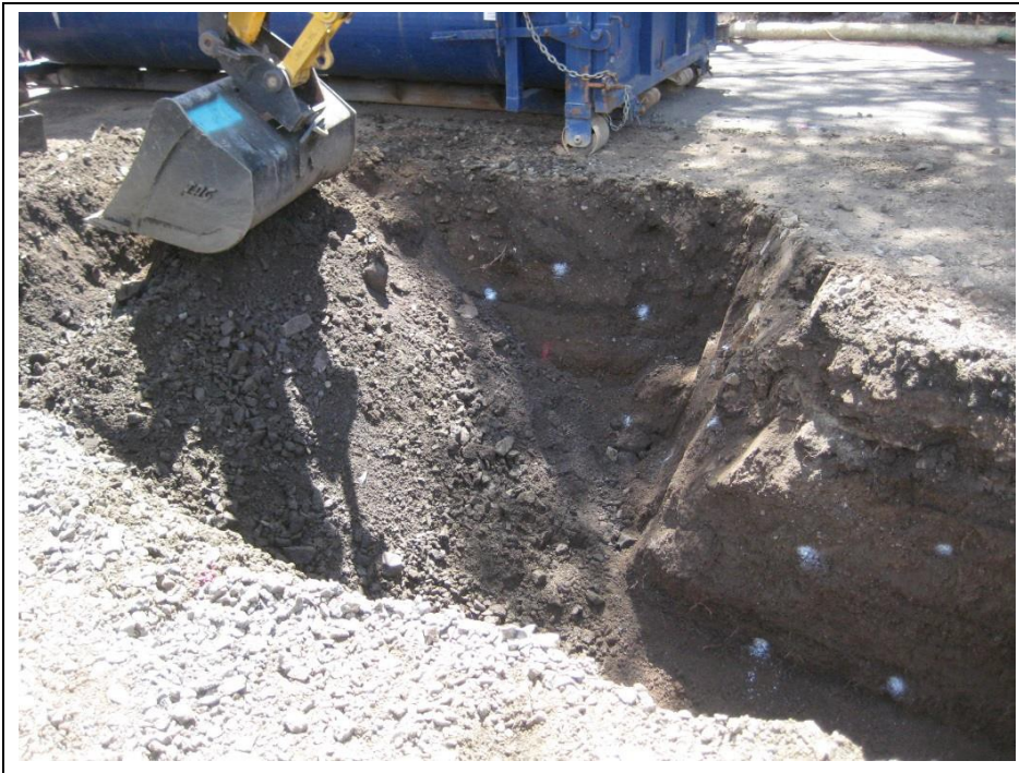
Photograph 9. Overview of open excavation. White dots were used to indicate areas where no further contamination was observed within the excavation. Aspect: south.
