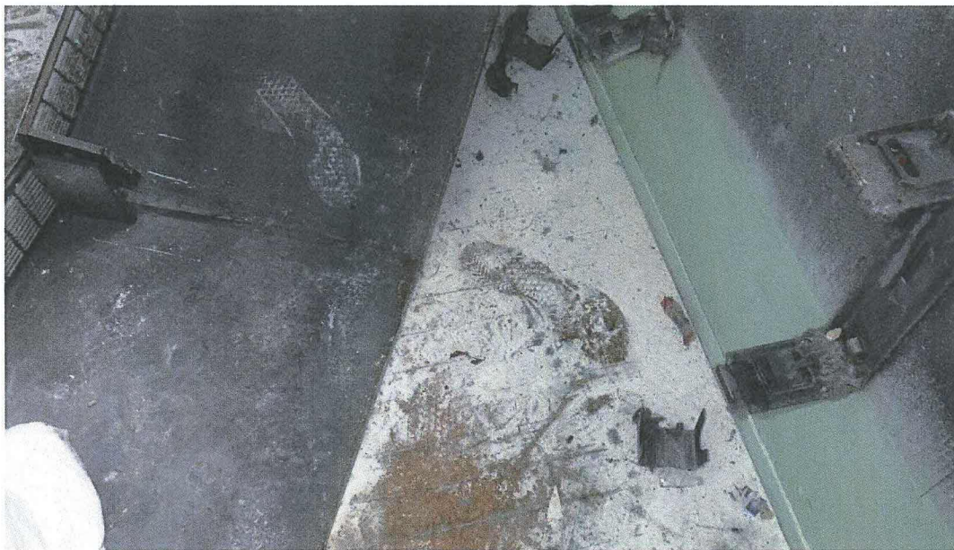
Photo 7: Friable asbestos on floor
