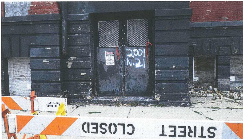
Photo 2: Warning sign posted on entrance; bricks crumbling from façade onto sidewalk
