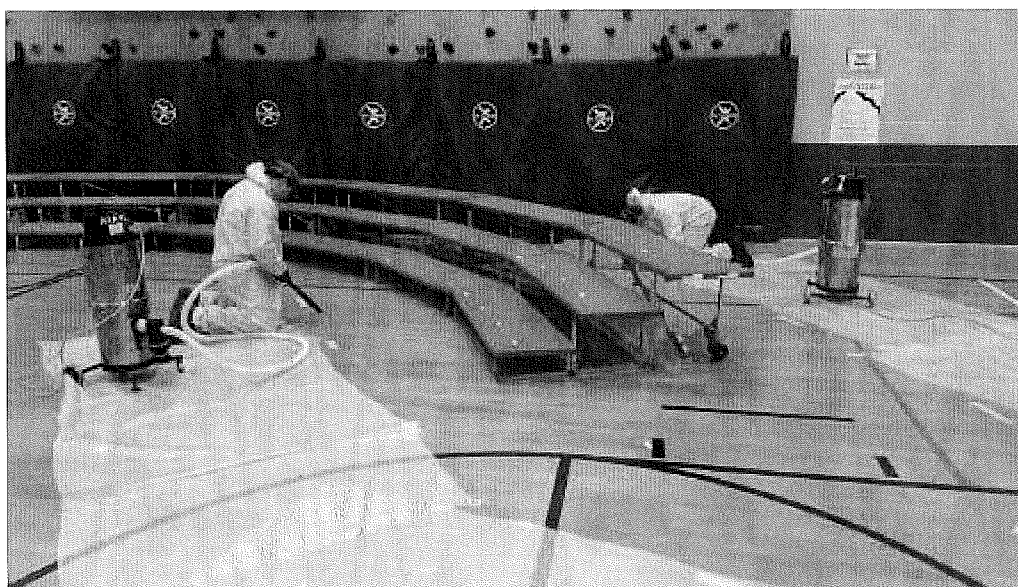
Photo 4: NSEC vacuuming mercury from Lincoln Elementary gymnasium floor
