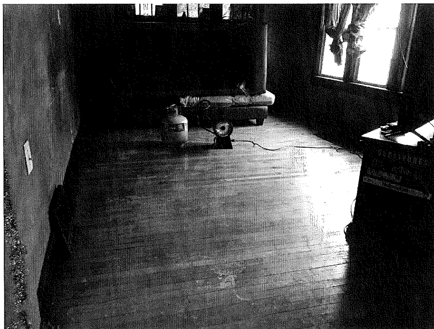
Photo 8: Heating after vacuuming and treatment with mercury decontamination solution
