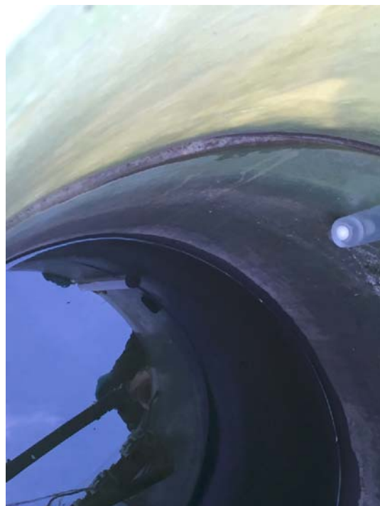
Photo No. IMG_3136; Taken on 12/09/15 at 14:01 hours by START-JW. Facing Down. Close-up of the shifted sump casing.
