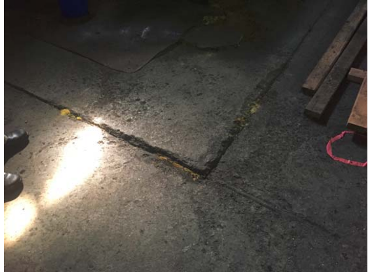
Photo No. IMG_3472; Taken on 05/19/16 at 9:53 hours by START-JW. Facing Down. Potential Cr+6 seeping from the ground through the concrete floor near the chrome plating pit.
