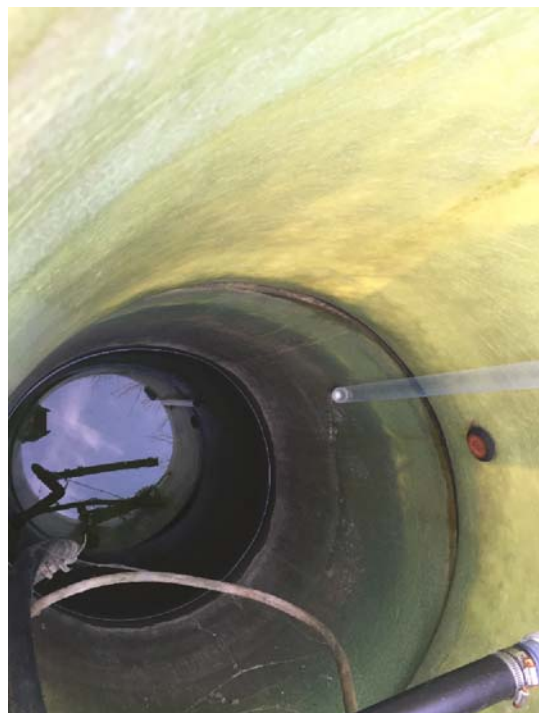
Photo No. IMG_3135; Taken on 12/09/15 at 14:00 hours by START-JW. Facing Down. Inside the Primary Sump Location. In the upper portion of the photo (near the bailer) there is evidence the sump casing has shifted at some point.
