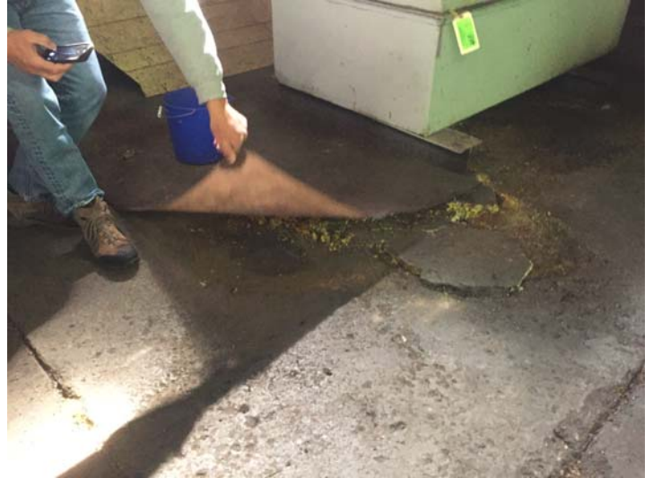
Photo No. IMG_3476; Taken on 05/19/16 at 9:58 hours by START-JW. Facing Down. Potential Cr+6 seeping from the ground through the concrete floor near the chrome plating pit.
