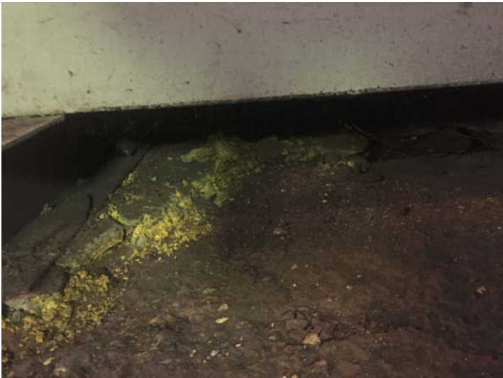
Photo No. IMG_3477; Taken on 05/19/16 at 9:58 hours by START-JW. Facing NA. Under a free-standing dipping pit, potential Cr+6 coming through the concrete.
