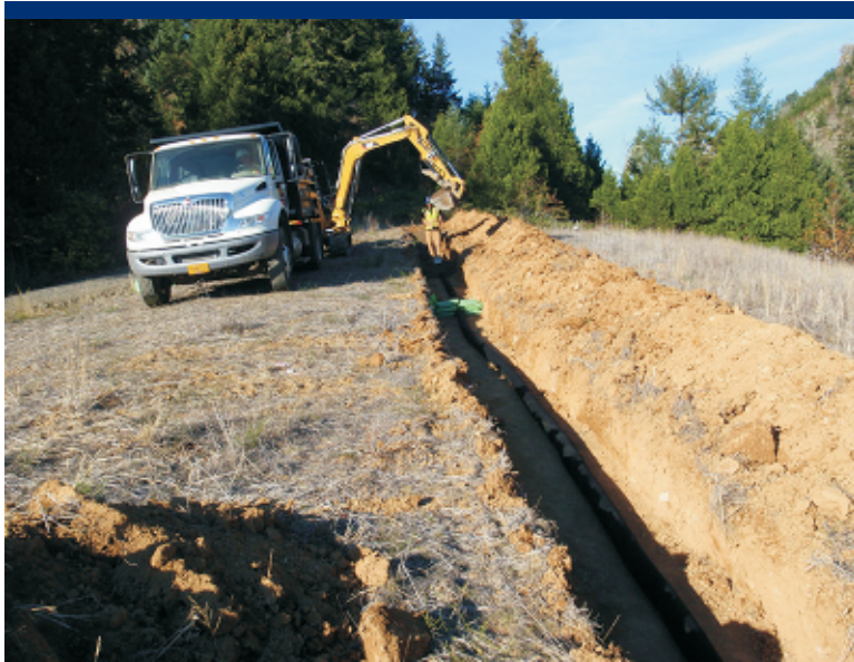
Photo 14 Installing lateral drain.
