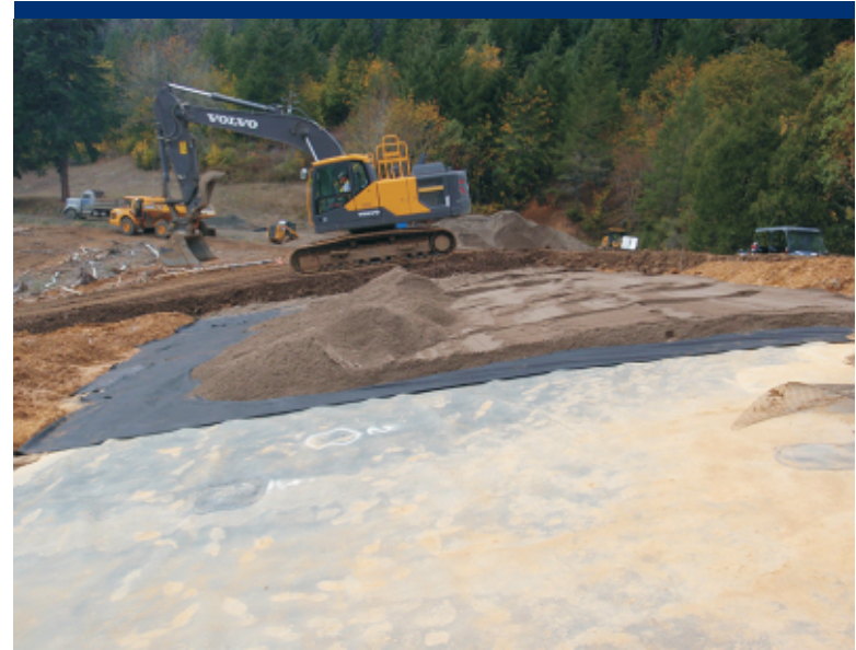
Photo 7 Placing sand layer on exposed LLDPE.
