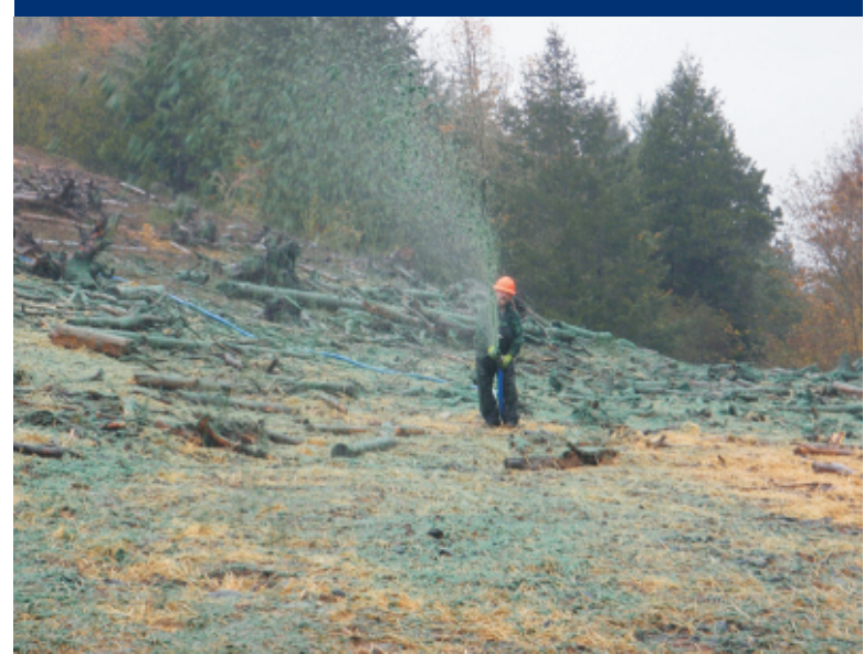
Photo 31 Hydraulic mulch and seed application.
