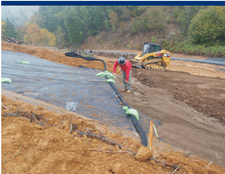
Photo 16 Installing lateral drain across area of exposed LLDPE.
