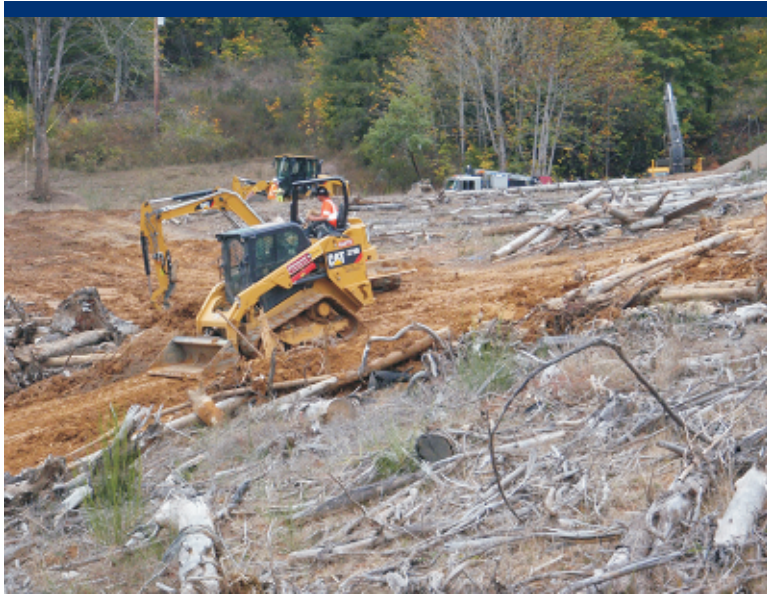
Photo 6 Installing drain trenches.
