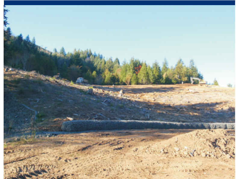
Photo 11 Southwestern end of gabion wall.
