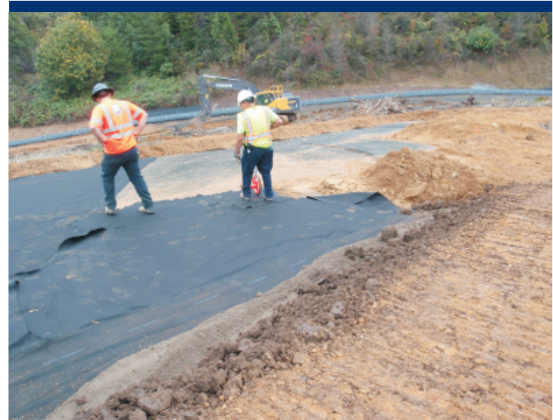
Photo 15 Placing geotextile.
