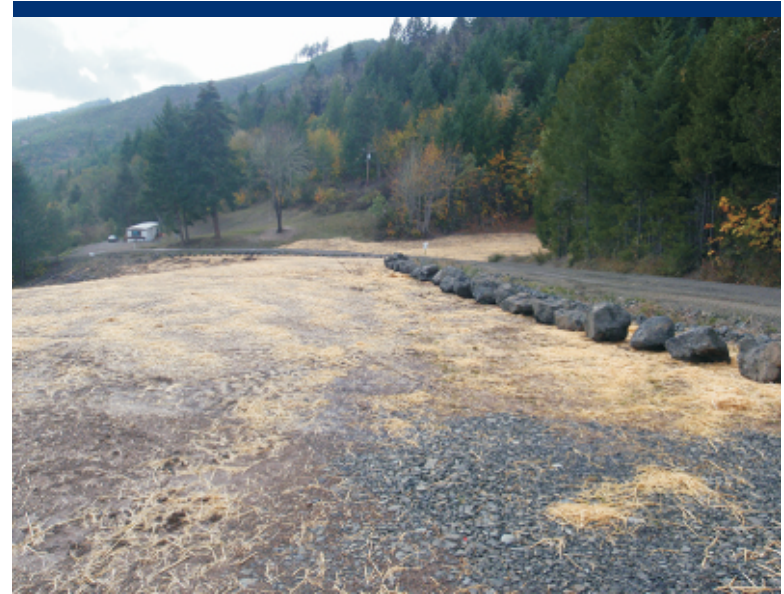
Photo 23 Boulder row on top of repository.
