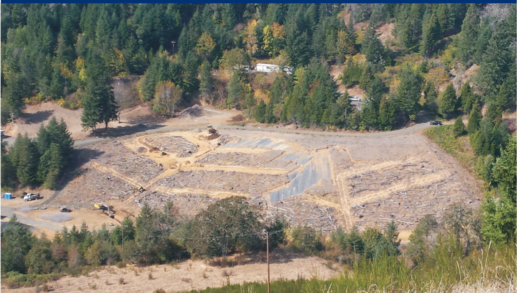
Photo 1 View of repository, showing areas cleared for subsurface drain installation.
