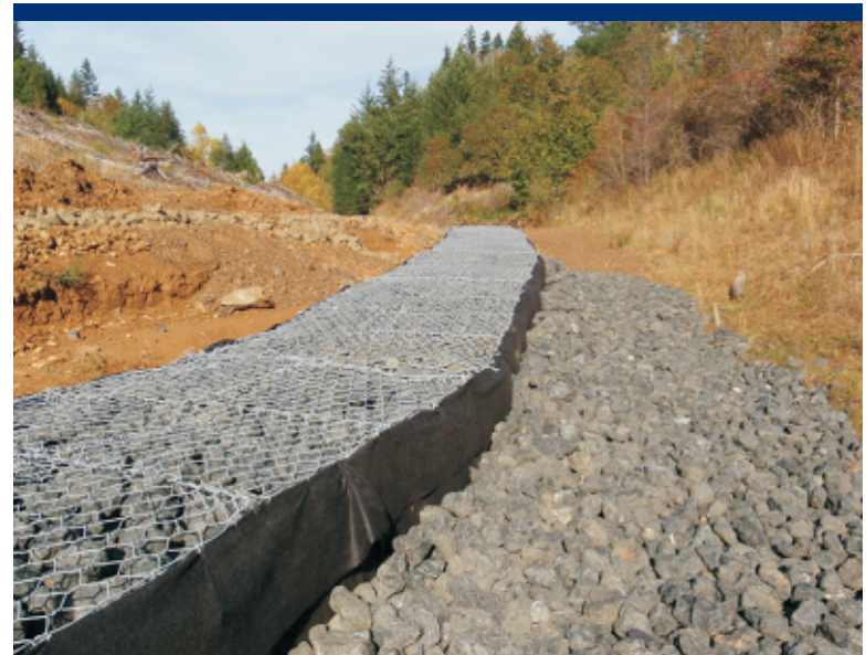
Photo 5 Gabion installation.
