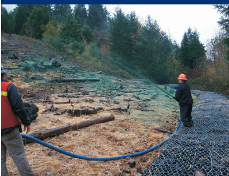
Photo 30 Hydraulic mulch and seed application.
