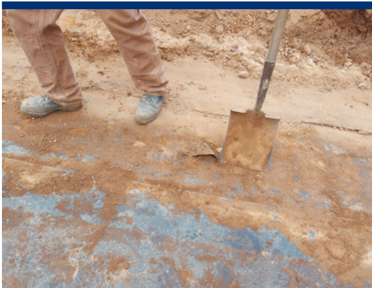
Photo 12 Tear in LLDPE, prior to repair.
