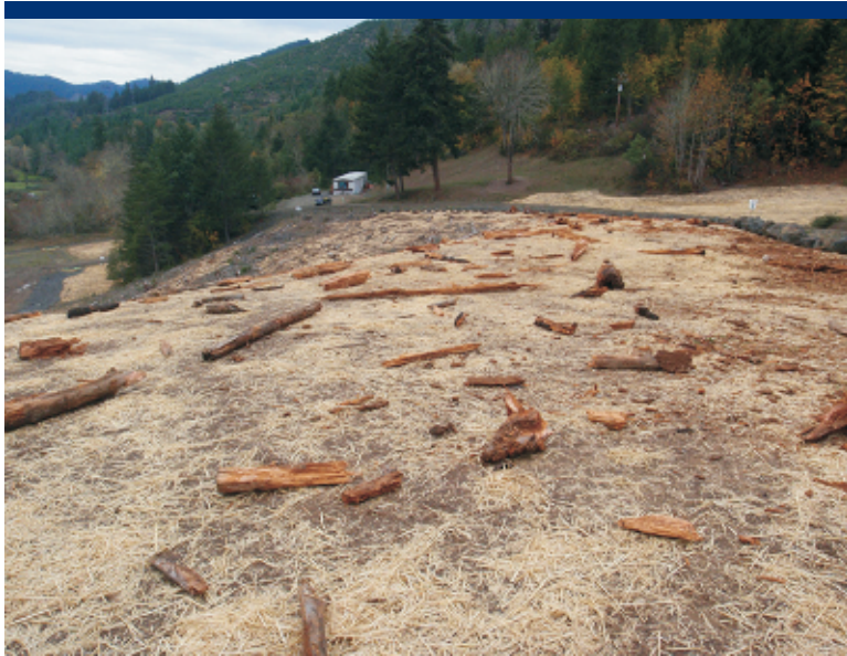
Photo 26 Upper slope of repository, after spreading straw and slash.
