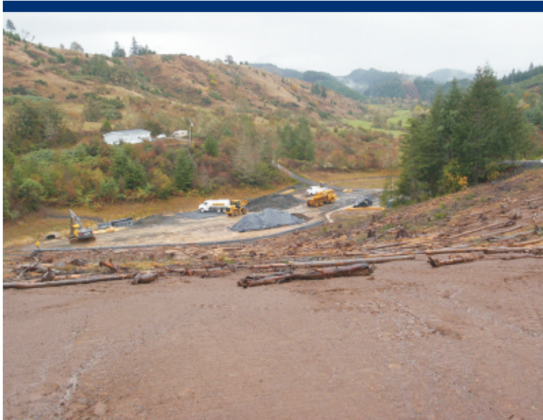
Photo 22 Restored cover soil on upper slope of repository.
