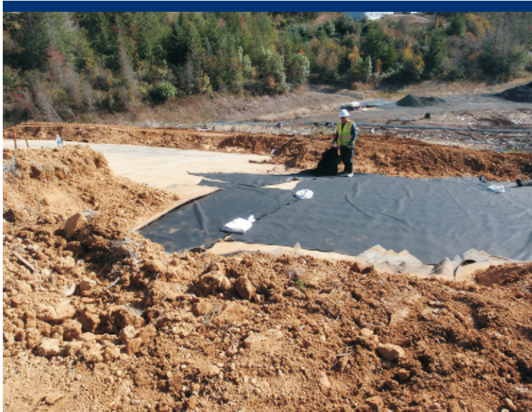
Photo 10 Geotextile placement.
