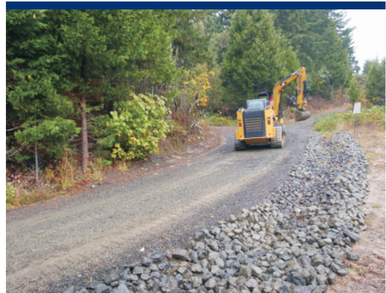
Photo 21 Restoring rock-lined run-on control ditch.
