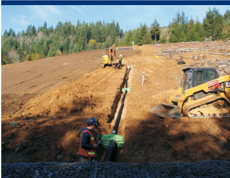
Photo 18 Completing lower end of down-drain.
