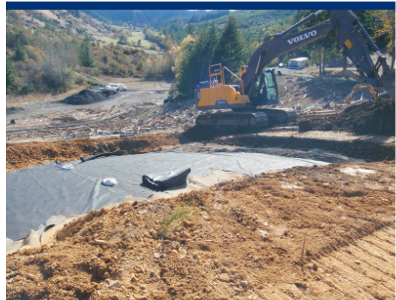
Photo 9 Placing sand layer on LLDPE.
