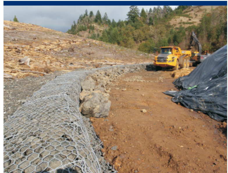
Photo 25 Placing riprap boulders below southwestern end of gabion wall.
