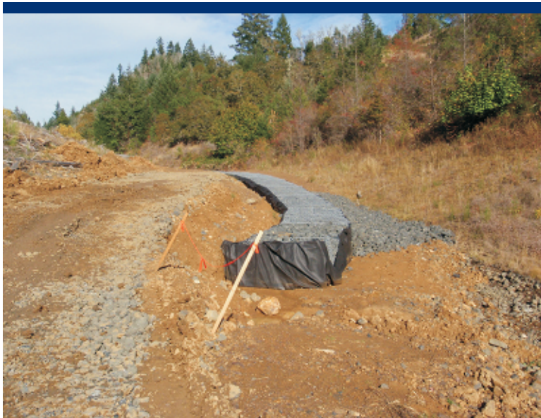
Photo 4 Gabion installation.
