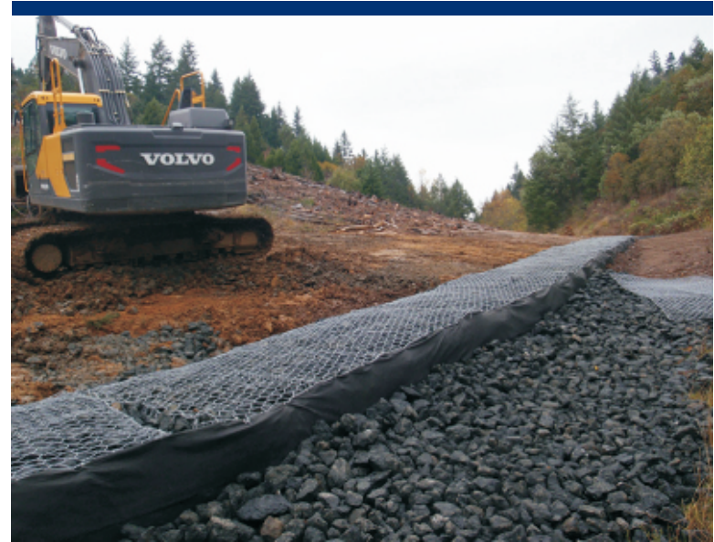
Photo 19 Backfilling behind gabions.
