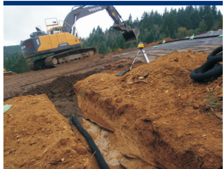
Photo 17 Lateral drain installation.
