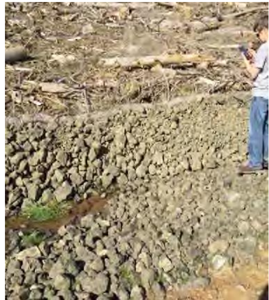
Photo 2-2: Toe drain seep below the southeast face of the repository
