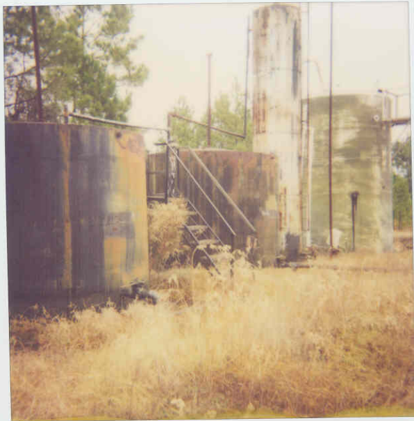
Quality Petroleum, Inc. (Q008) Hoffman ETAL #001 Production Facility Sec. 4, T21N, R16W CPI (2152) Caddo (009) 12-5-02
