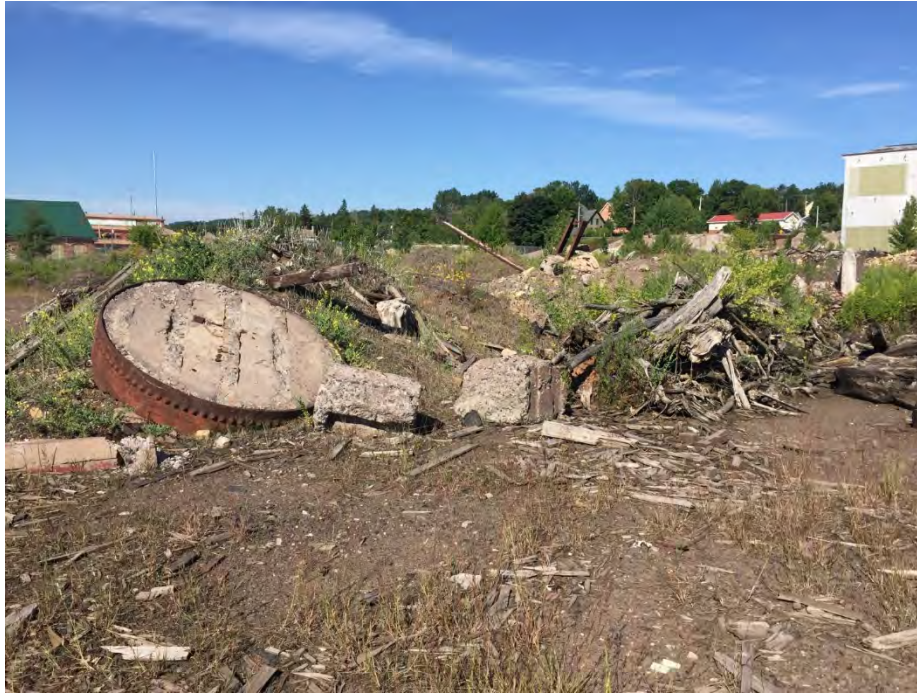
Photograph 17: WP-17 containing concrete pieces, wood, bricks, slag, and metal mixed with soil. The material appears older in nature. Photograph by J. Chrestensen, July 20, 2016.
