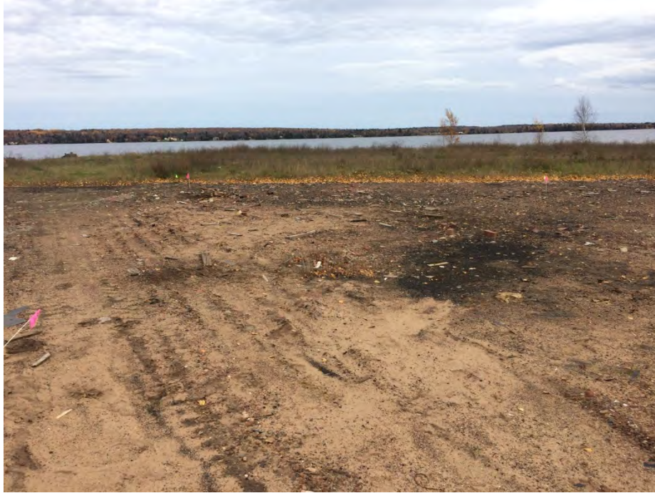
Photograph 35: WP-48 residual, primarily fine to medium grained sand with some wood and metal debris, and deteriorated corrugated cardboard. Photograph by MDEQ, October 23, 2017.
