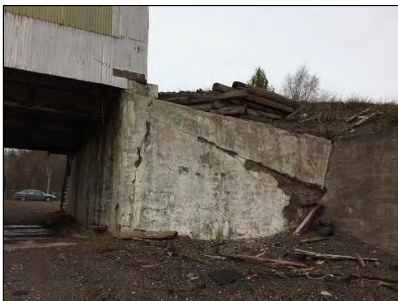
Photo 3: View of fallen roofing material near the northeast corner of the Mineral Building on the lake side. Photo taken: November 28, 2017.
