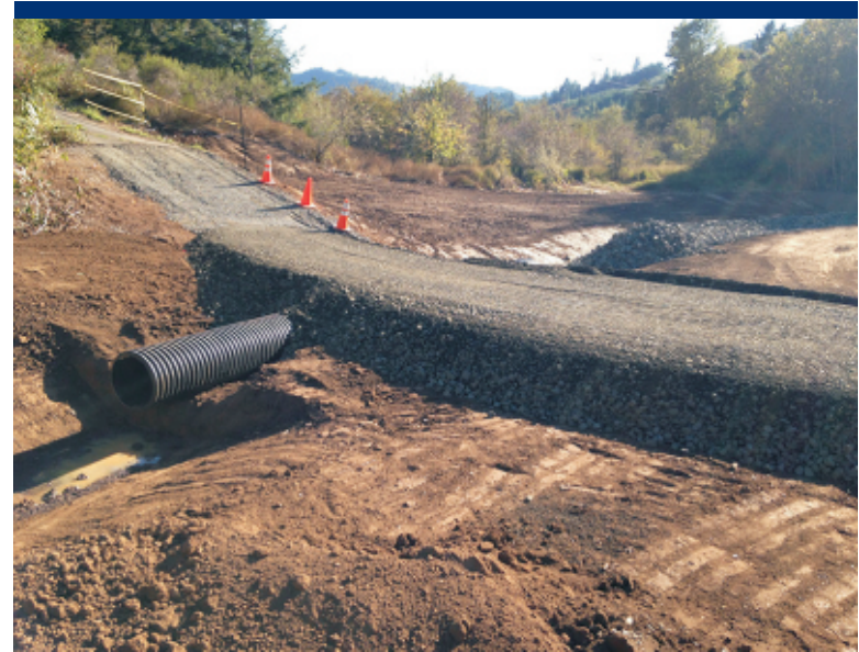
Photo 40 New 24 inch culvert installed between Area 1 and Area 2 leading to Residence 3.
