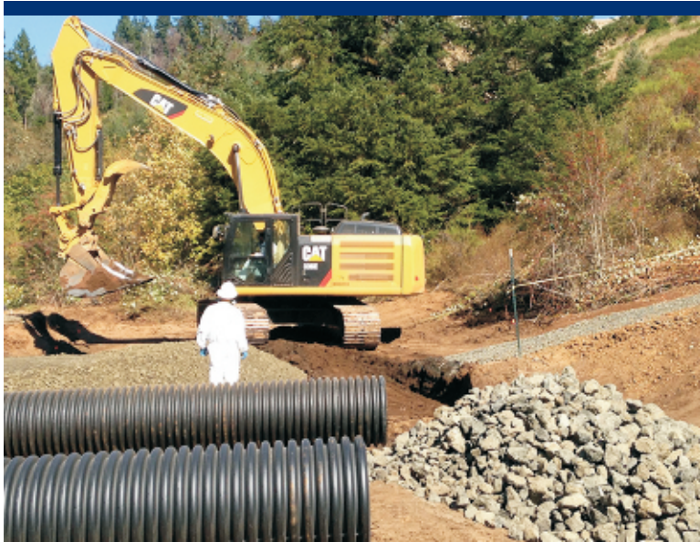
Photo 39 Replacing a culvert leading to Residence 3 from Area 2.
