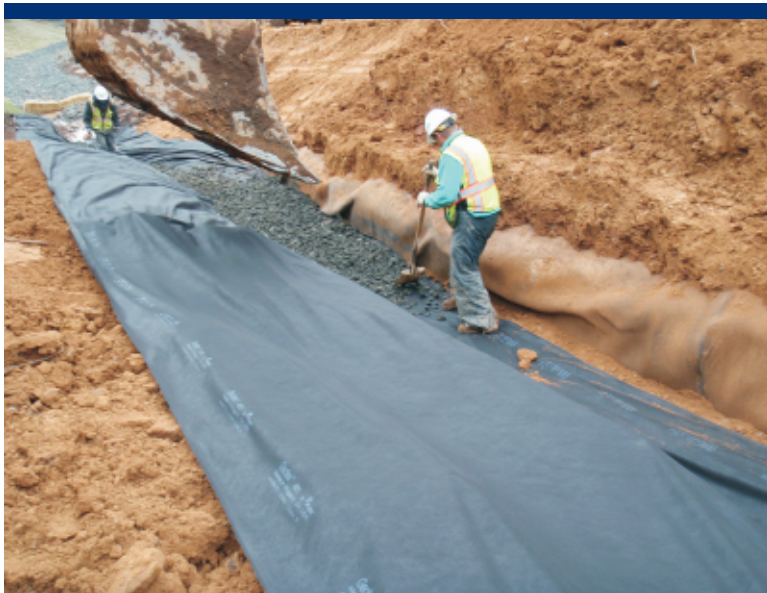
Photo 60 Installation of toe drain at the foot of the repository.
