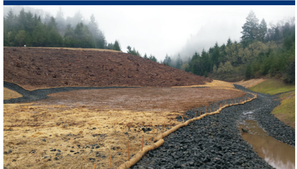
Photo 71 View of Area 1 with the finished repository in the background and multiple armored drainage channels.
