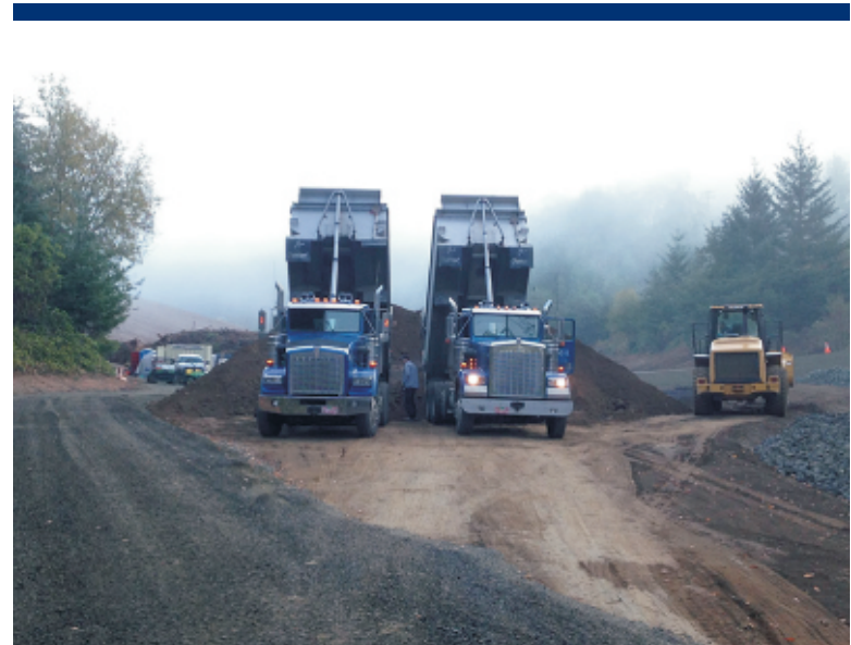
Photo 57 Staging clean backfill in Area 2.
