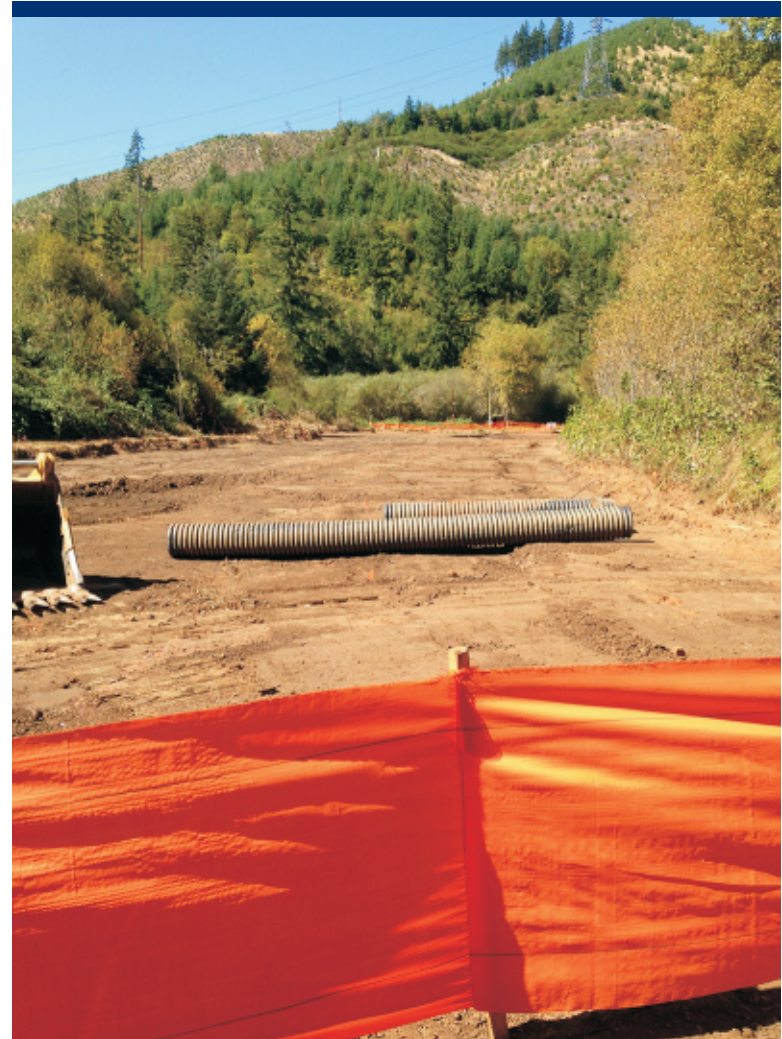
Photo 43 Excavation in Area 4 prior to installation of culverts.
