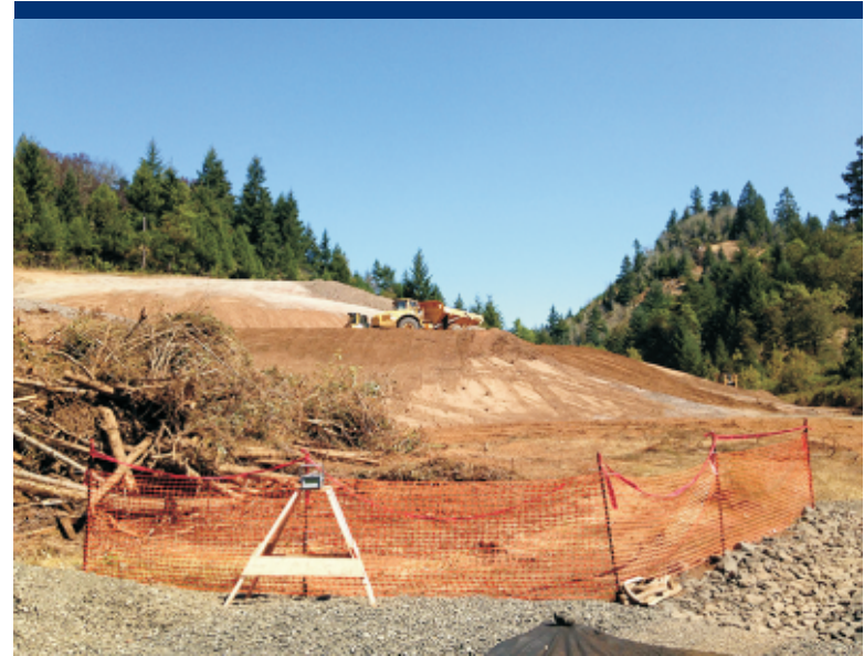
Photo 30 Repository construction with DataRam 4000 particulate monitor in the foreground.
