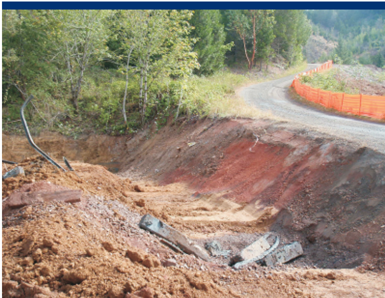
Photo 23 Exposed sidewall containing red calcine in the former Mill Site.
