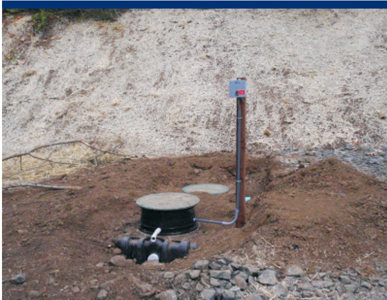
Photo 62 Installed septic tank at Residence 6.
