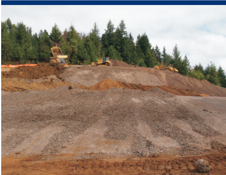
Photo 29 Construction of the repository with excavated mine waste material from the former Mill Site.
