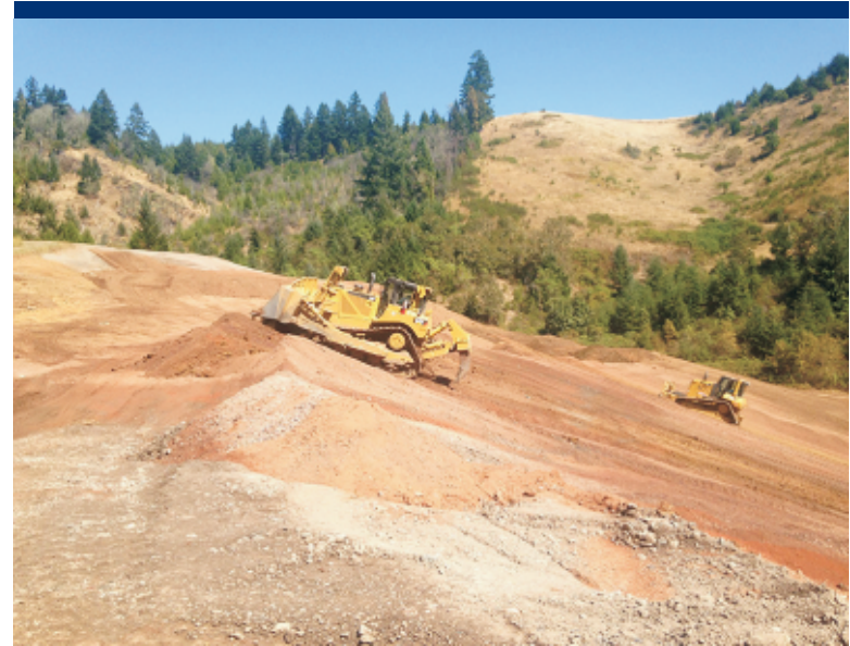
Photo 45 Grading and shaping the repository with heavy equipment.
