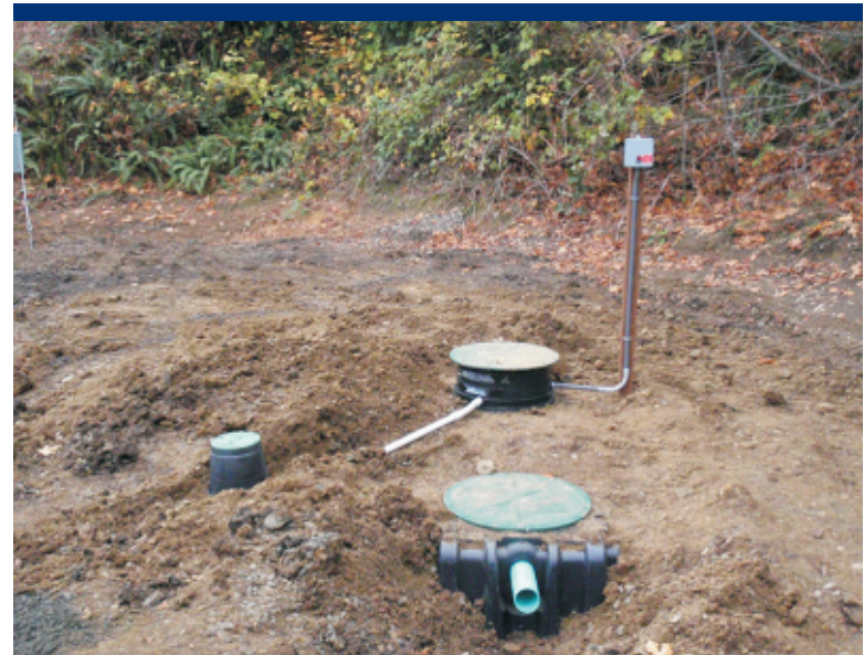
Photo 61 Installed septic tank at Residence 1.
