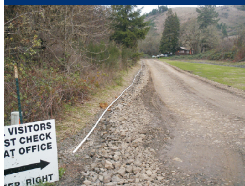
Photo 59 Road leading past Area 4 with water line temporarily exposed along the north side of the road.
