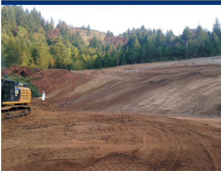
Photo 44 Expanding the repository to the west to accommodate increased volume of excavated material.
