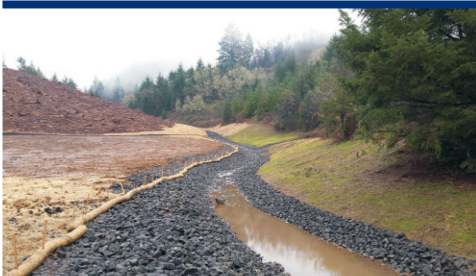
Photo 70 Armored channel leading past Area 1 and the repository.
