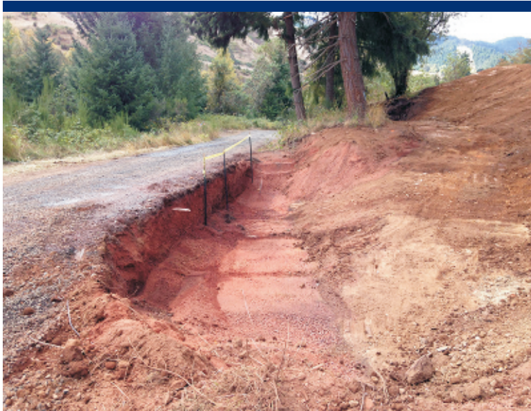
Photo 50 Excavation of mine-waste material at Residence 2 along the upper road.
