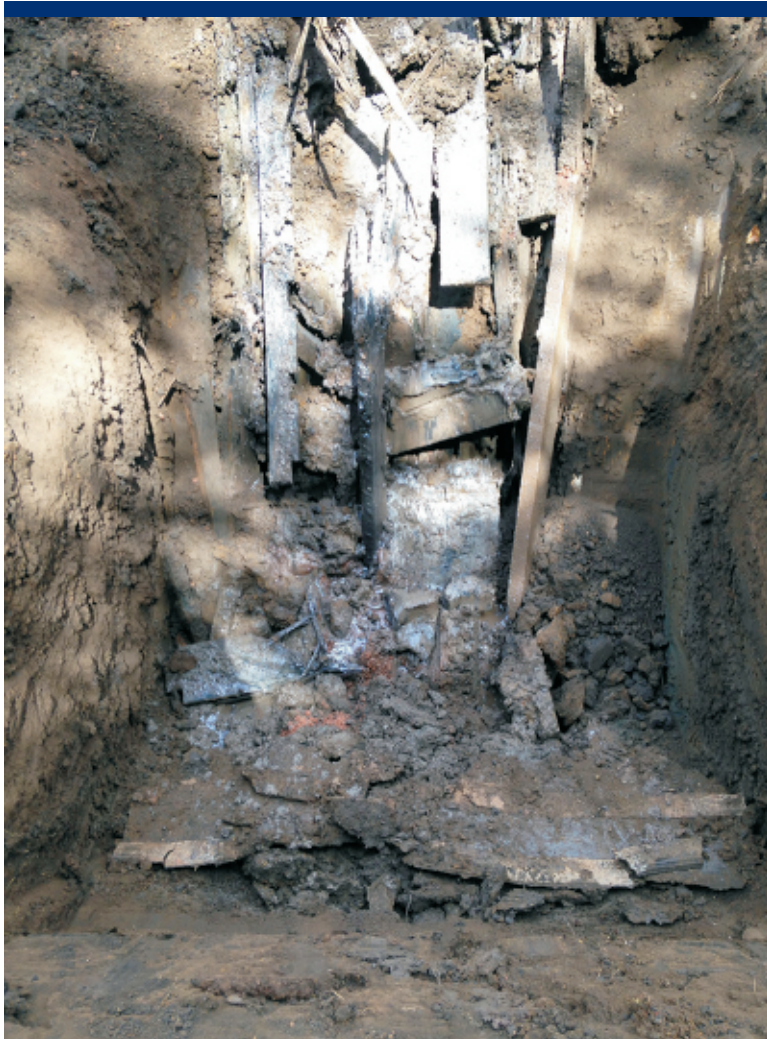
Photo 36 Excavated mine feature in Area 2 to a depth of 8 feet bgs.
