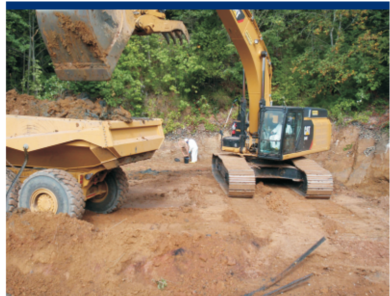
Photo 24 Excavation of the former Mill Site; a section containing free mercury was marked with orange spray paint.
