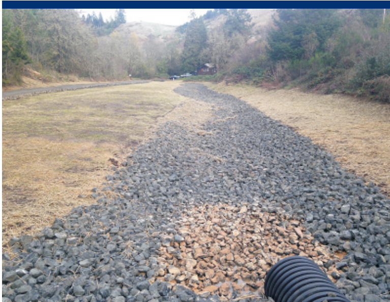
Photo 58 Armored channel and culvert in Area 4.
