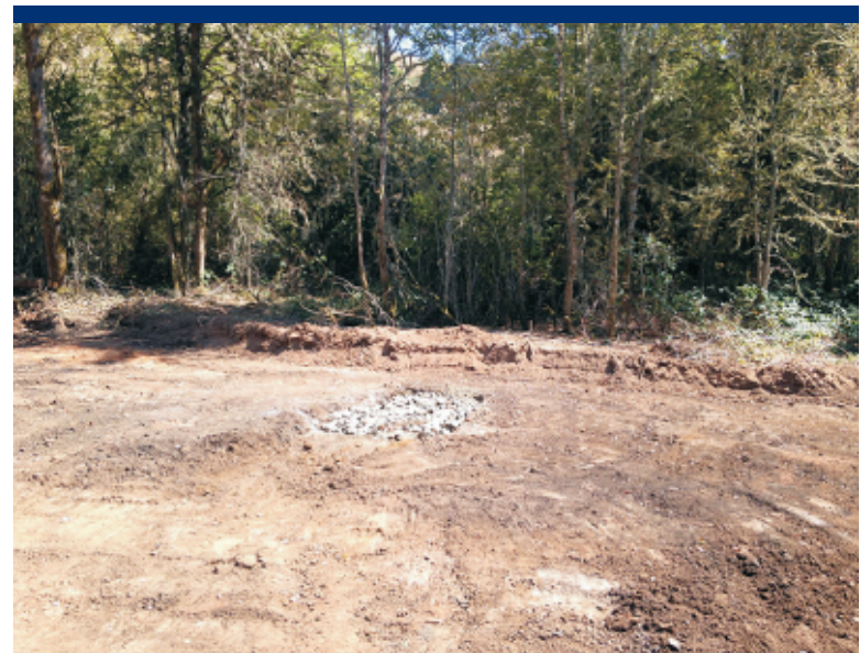
Photo 38 Mine feature backfilled with 4- to 8-inch rock.
