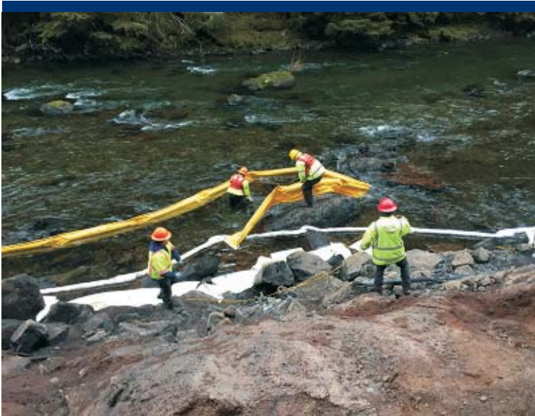
Photo 9 NWFF Environmental installing hard boom on North Santiam River.
