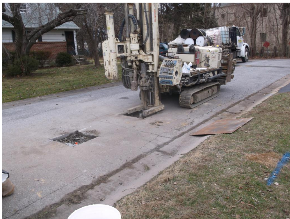
PHOTOGRAPH 4: GEOPROBE rig constructing MW-22 Shallow.
