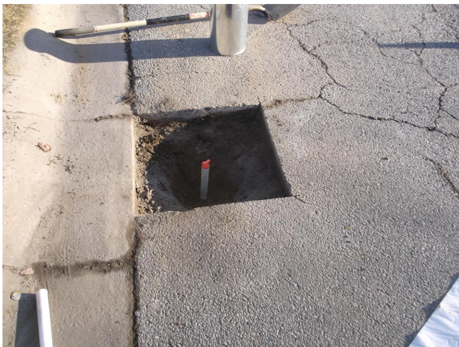
PHOTOGRAPH 1: Monitoring well (MW)-23 before the installation of the well box.
