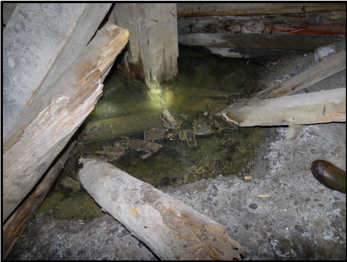
Photo 31: Collapsed Timbers at Bachelor Shaft Nelson Tunnel landing
