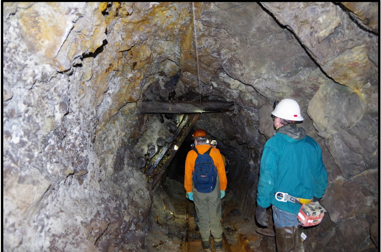
Photo 56: Area of clay gouge in left rib near 47+10
