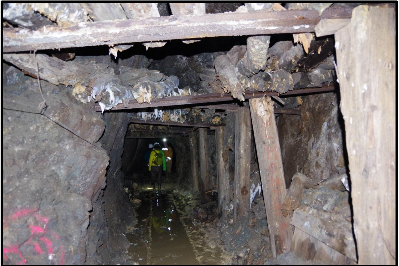
Photo 51: Raise with steel rail, wood posts, and rotten cribbing near 44+00
