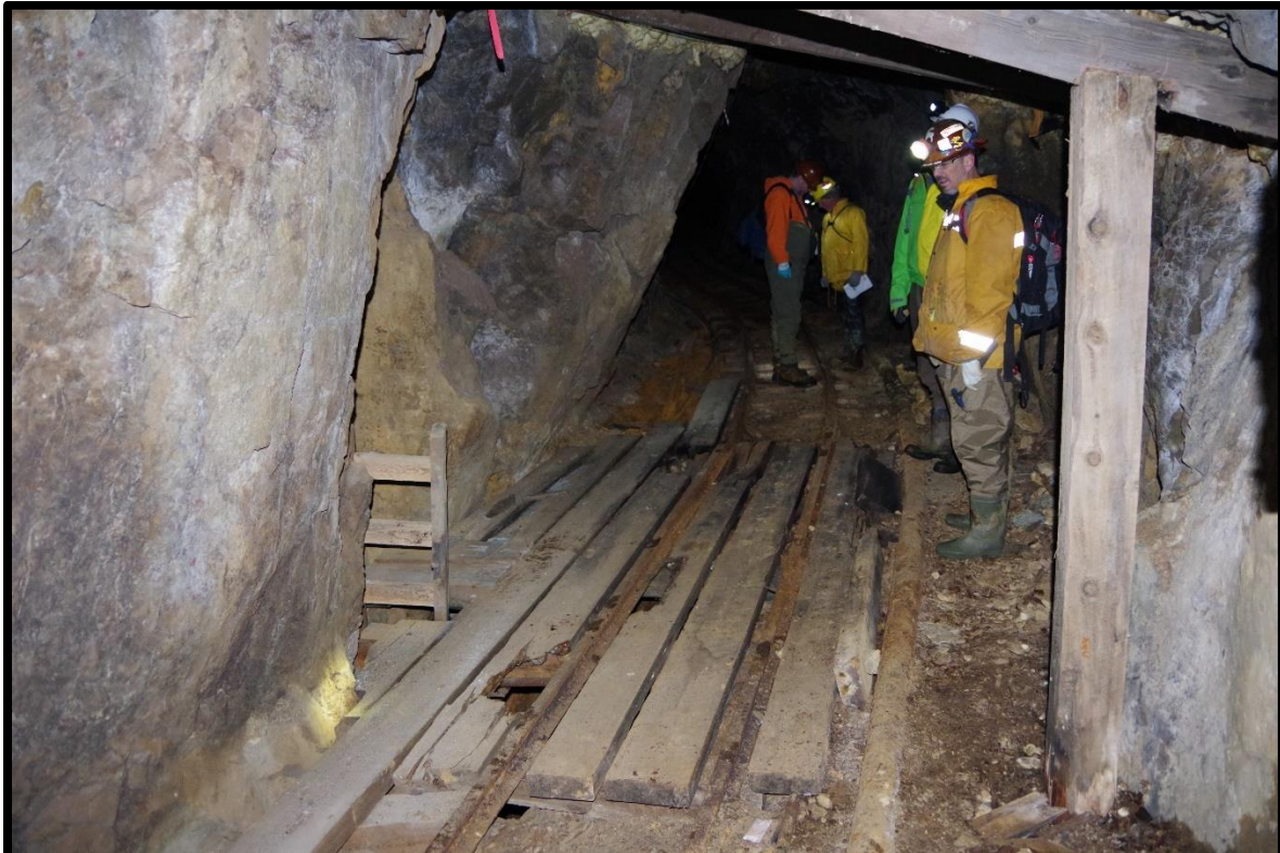
Photo 16: Overview of Daylight Winze; Note decayed wood cover
