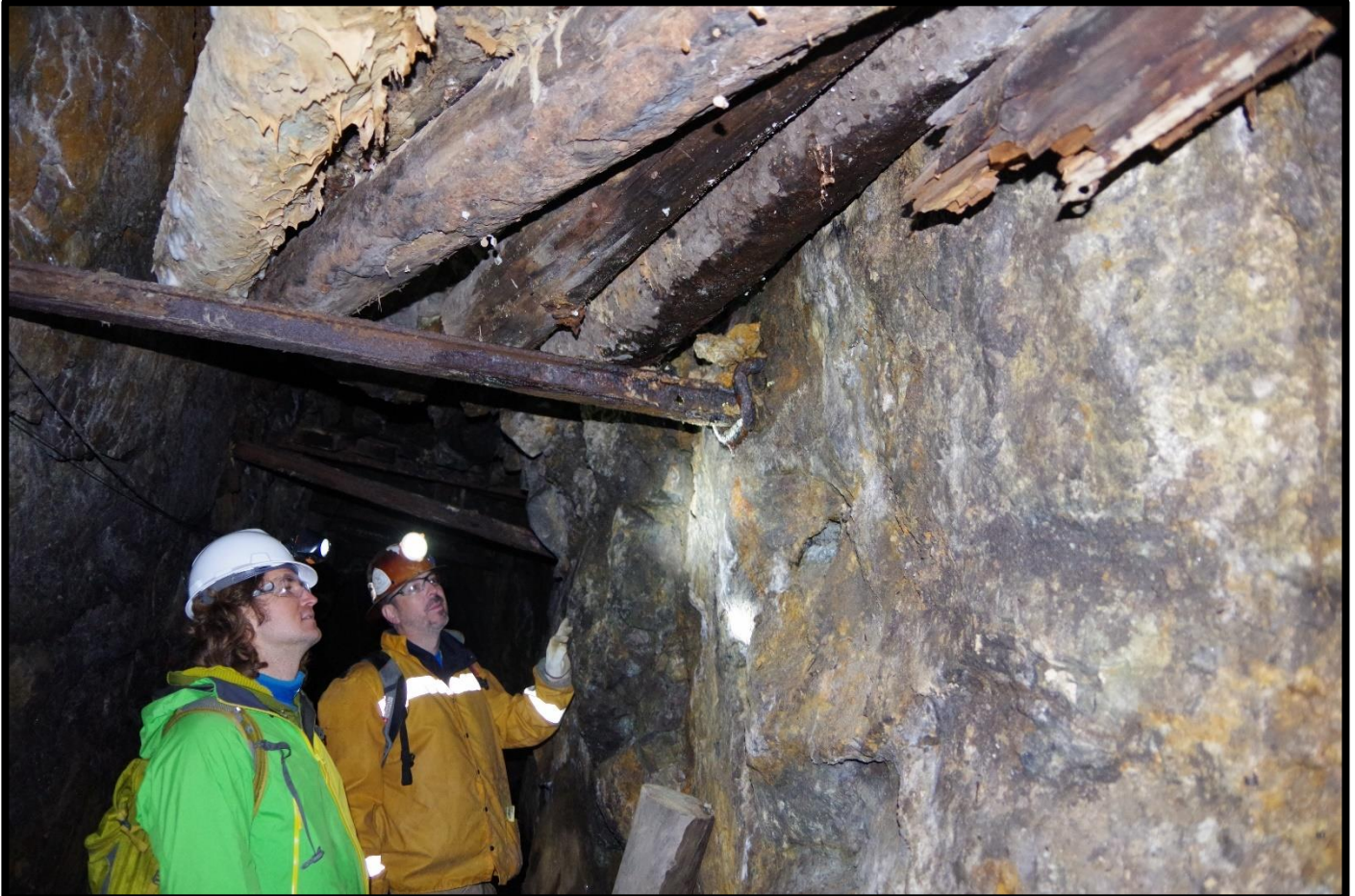
Photo 43: Steel rail stulls and rotten wood lagging near 37+50
