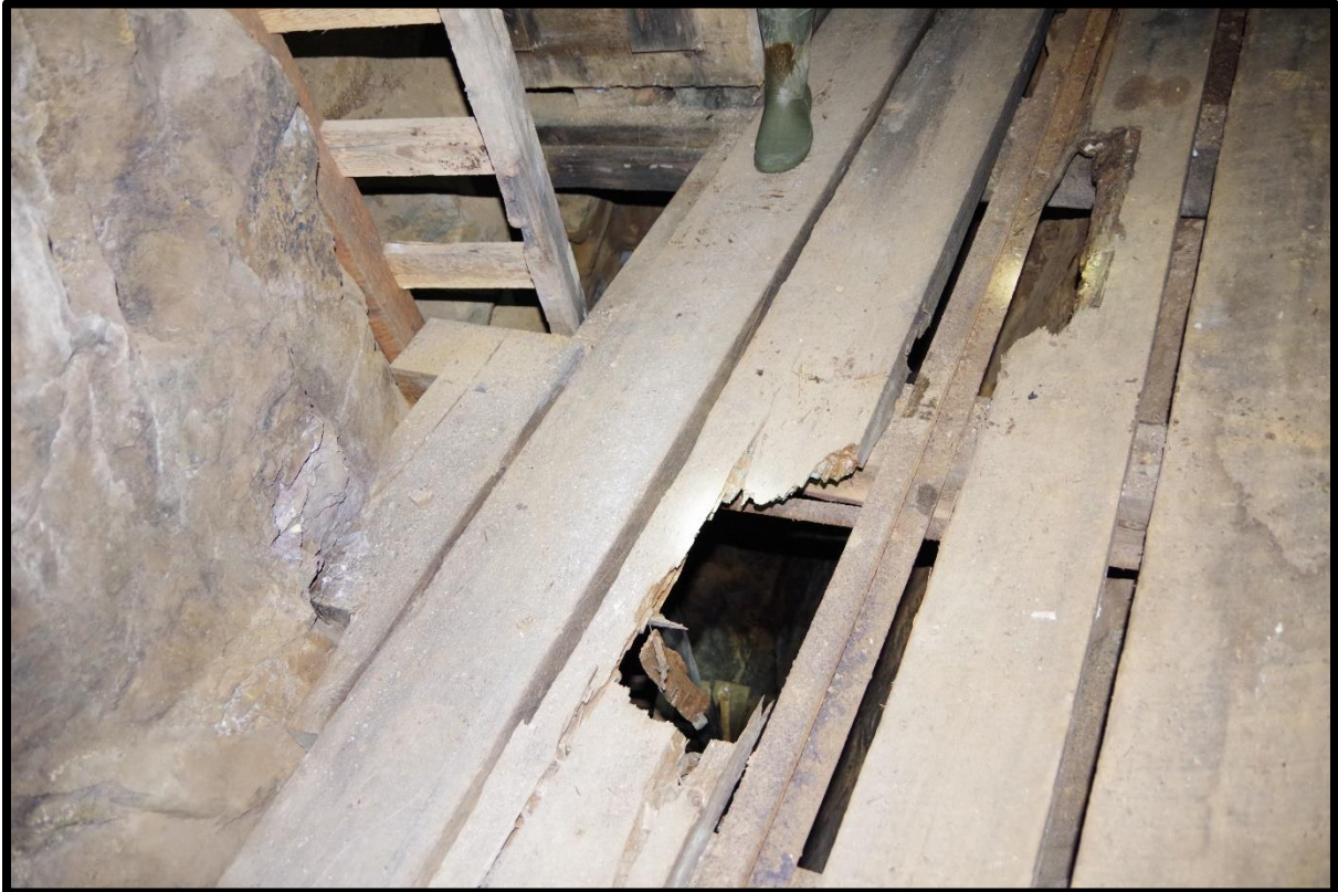
Photo 17: Daylight Winze with rotten wood cover
