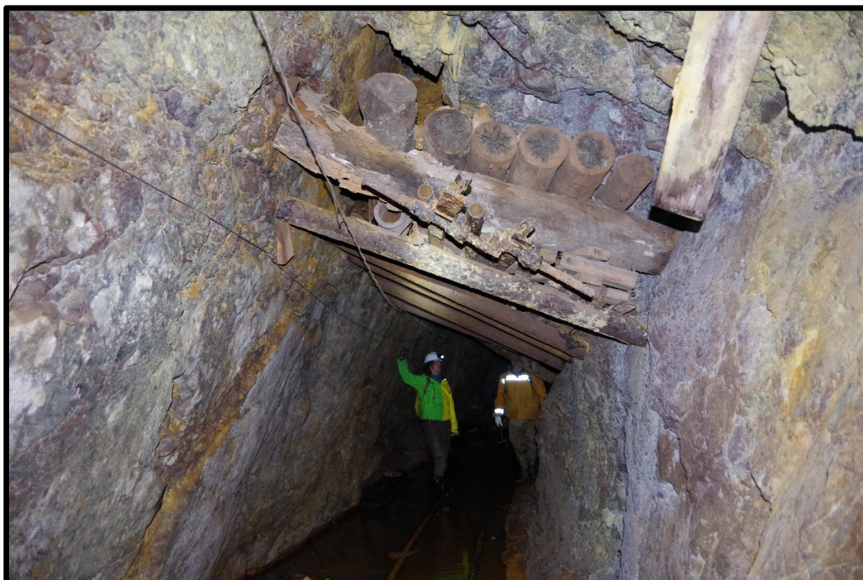
Photo 39: Steel pipe stulls near 32+20; Note pipe cribbing
