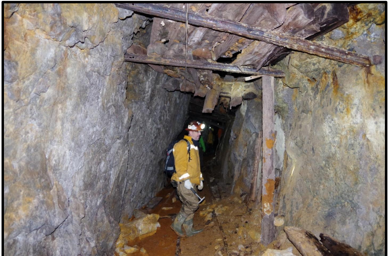
Photo 36: Steel rail stulls with rotten timber lagging 30+50
