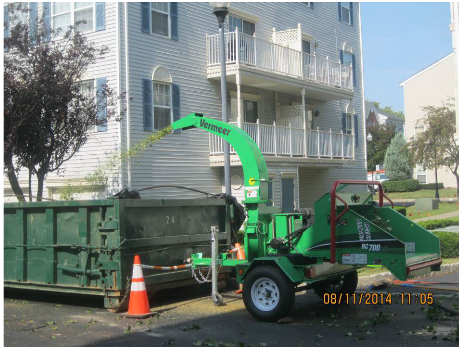
Photograph 7: Tree branches and shrubs were mulched using a wood chipper; the debris was placed directly into roll-off containers.
