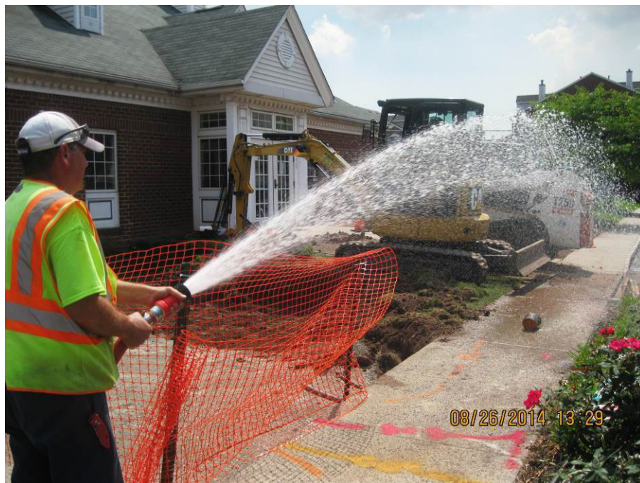
Photograph 2: During the excavation of on-site AOCs, particulate levels were suppressed by wetting the excavation area with water.
