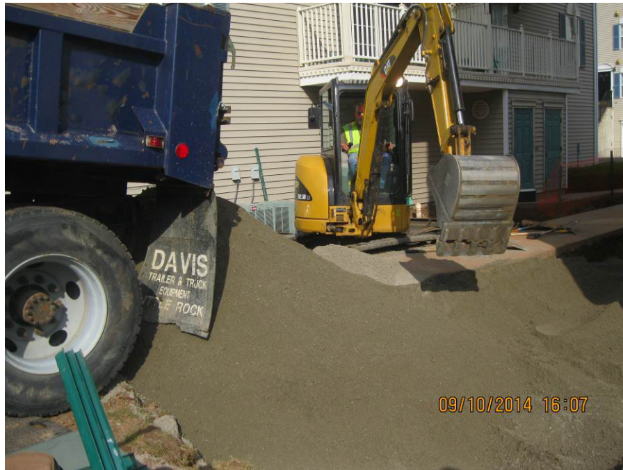
Photograph 13: Each excavated AOC was backfilled with pre-analyzed clean fill (quarry dust) to 12-inches bgs. A vibrating compactor was used to compact the clean fill.
