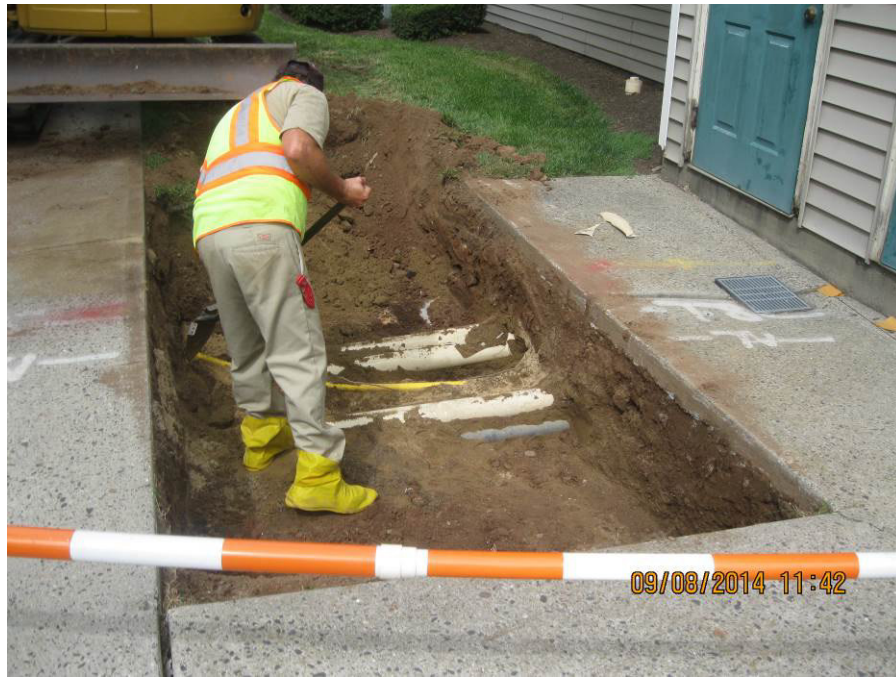
Photograph 5: Hand digging around underground utilities.
