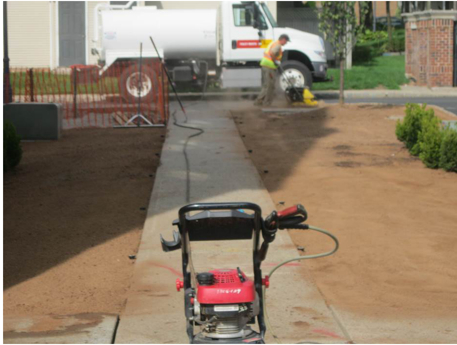
Photograph 15: The crew compacting backfill materials. Particulate exceedance spikes were sometimes observed on the air monitors during backfill operations. Although lead contaminant migration was not a concern the established engineering controls were implemented as a corrective action.
