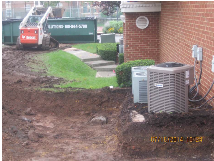
Photograph 8: A skid-steer loader was used to transport and deposit excavated soils directly into polyethylene-lined mobile roll-off containers which were staged close to the work area at each AOC. Soils around A/C units were not excavated to avoid service disruption. Using an XRF analyzer, soil screening around A/C units and surface utility boxes was conducted to document the concentration of lead in the soils.
