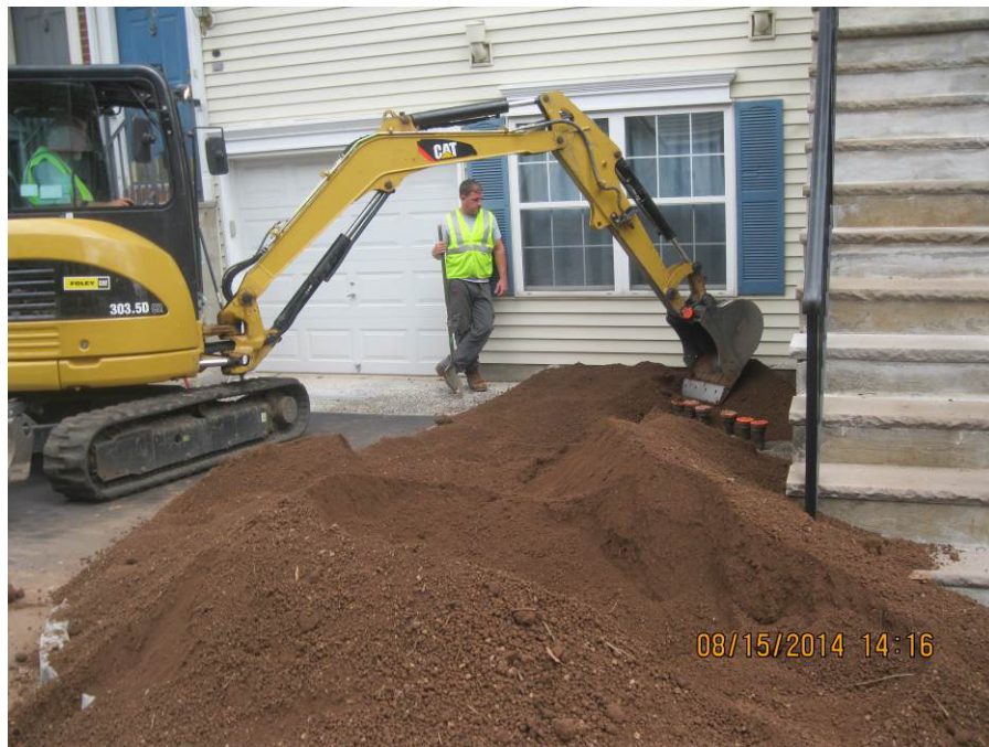
Photograph 14: 12-inches of pre-analyzed topsoil was placed on top of the clean fill and compacted to bring the ground level to its pre-existing surface elevation while ensuring that the original landscape was maintained.
