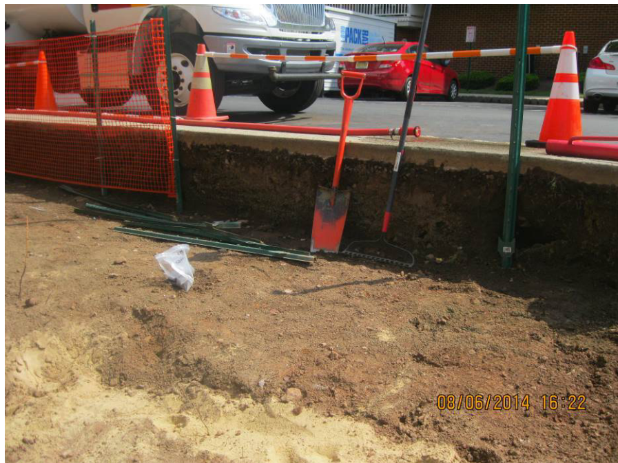
Photograph 4: The majority of on-site AOCs were excavated to a target depth of 2-feet bgs. Some locations could not be excavated due to their proximity to permanent structures, including sidewalks and utility pads.
