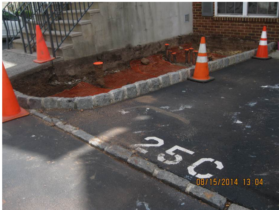
Photograph 12: Prior to backfilling each AOC, orange safety fence was installed on the excavation floor as a warning barrier demarcating where the concentration of lead in soils was above the EPA RSL of 400 mg/kg for residential soils.
