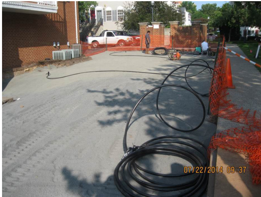
Photograph 9: The landscaping contractor installed and replaced sprinkler lines as part of Site restoration. The sprinkler lines at each AOC were tested after installation.
