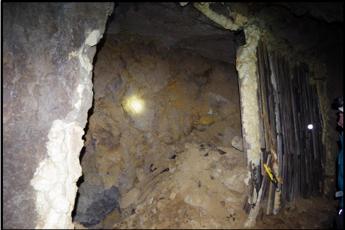
Photo 13: Close up of collapsed raise from Nelson Tunnel
