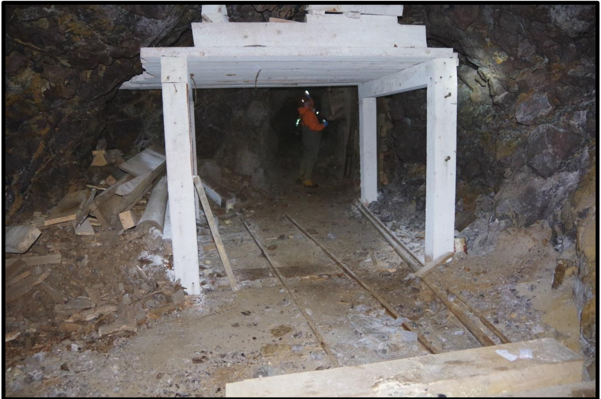
Photo 21: Moldy canopy in McClure Cross Cut
