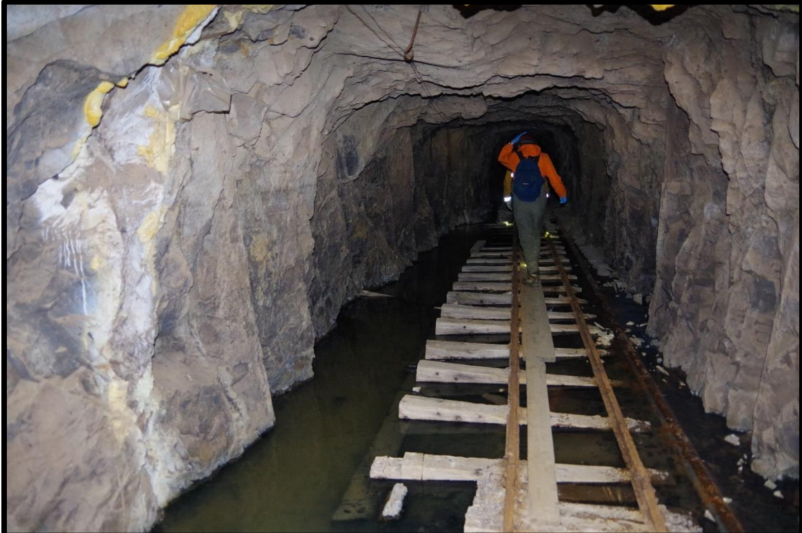
Photo 7: Floating rail ties and poor drainage near 1+00
