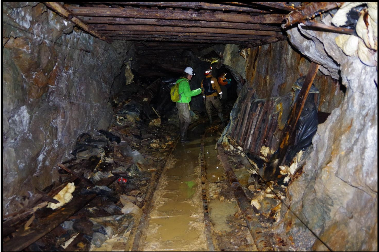
Photo 46: Abandoned heading near 41+00; Drift moves into foot wall
