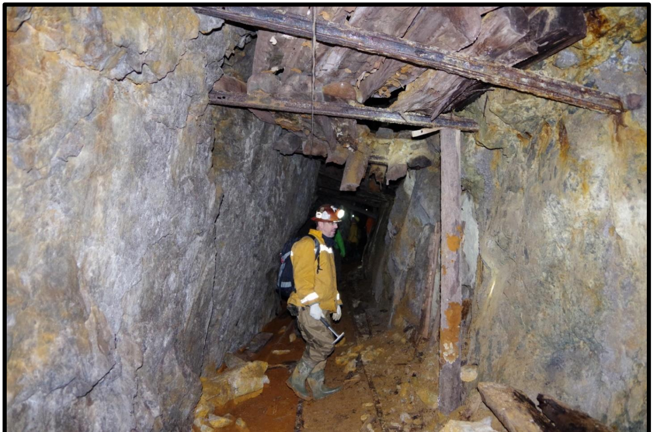
Photo 36: Steel rail stulls with rotten timber lagging 30+50
