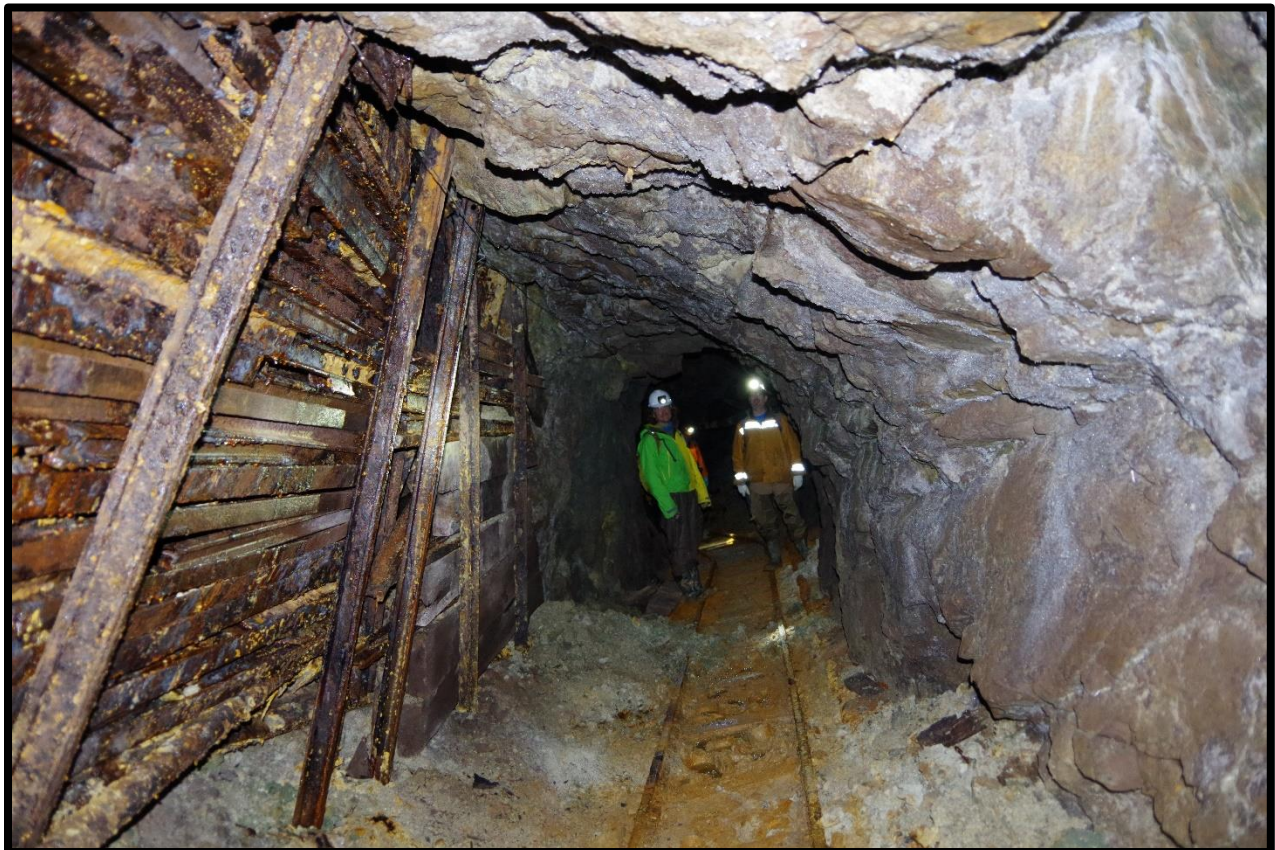
Photo 57: Area of clay gouge in left rib near 47+10; Note heavy steel rail lagging
