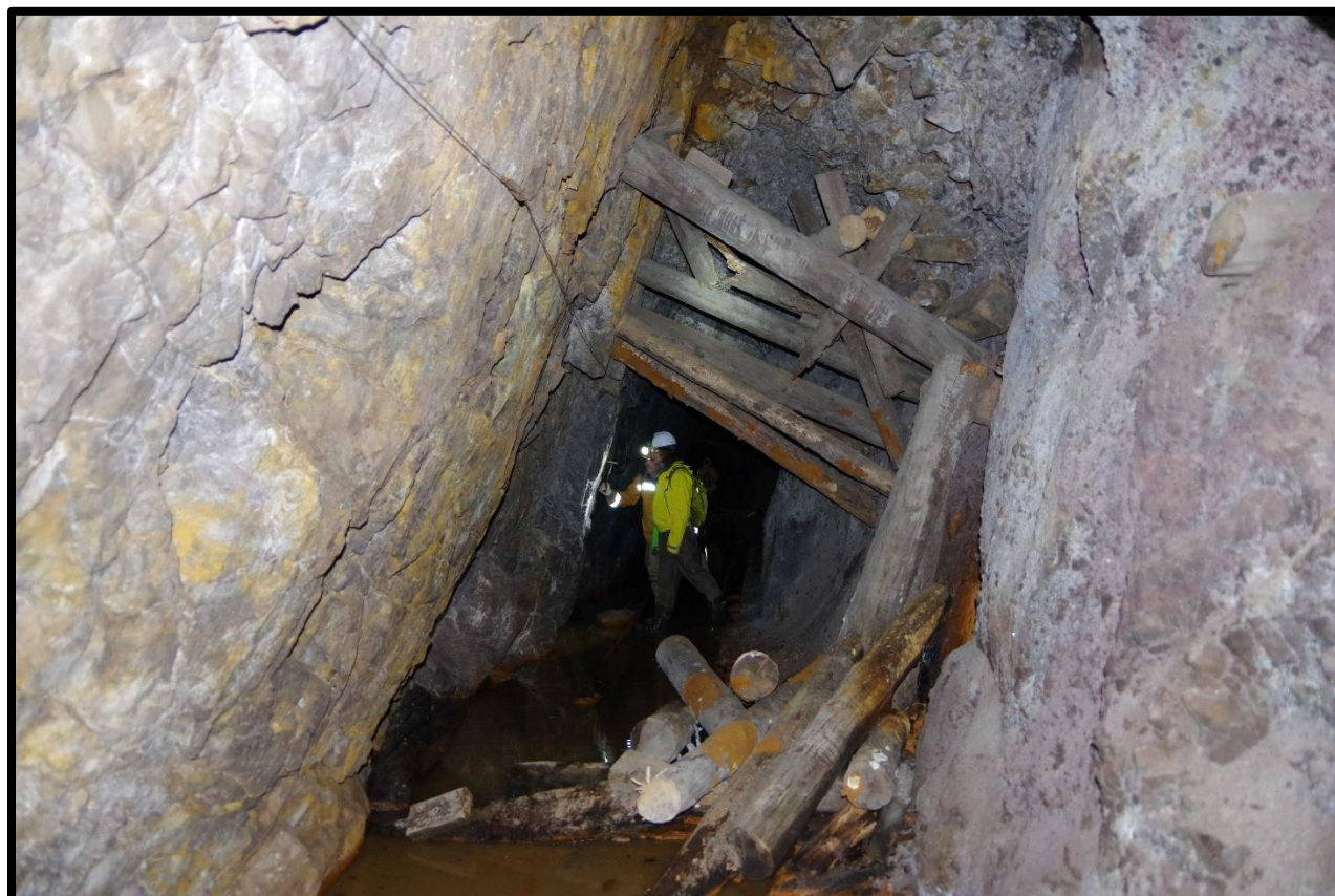
Photo 40: Failed timber stulls near 32+80
