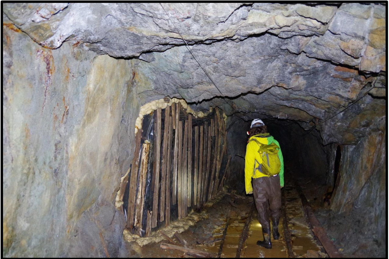
Photo 47: Sealed opening in left rib near 41+50; Loose debris is behind it
