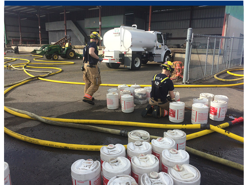
Photo 18 Portland Fire crew prepping Light Water™ ATC Plus™ for inline injection with firefighting stream.
