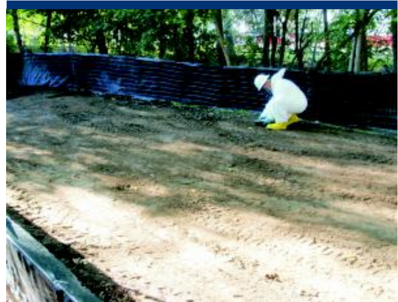
Photo 18 START collects soil composite sample following excavation of contaminated fill at 256 2nd Street.
