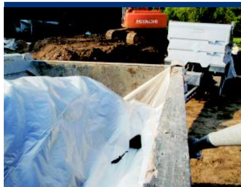
Photo 16 Contaminated material is covered with plastic in truck and pup beds.
