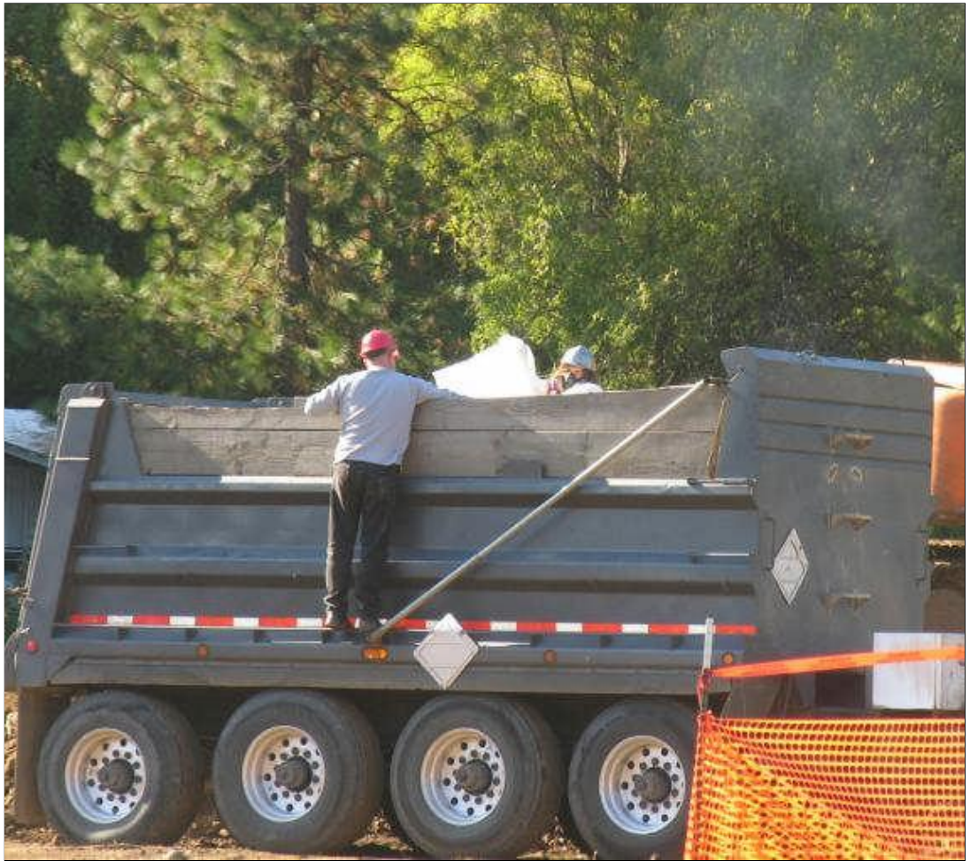
A truck driver and excavation site worker double cover the semi trailer before it heads out to deliver the load to a landfill between Medical Lake and Spokane, WA.
