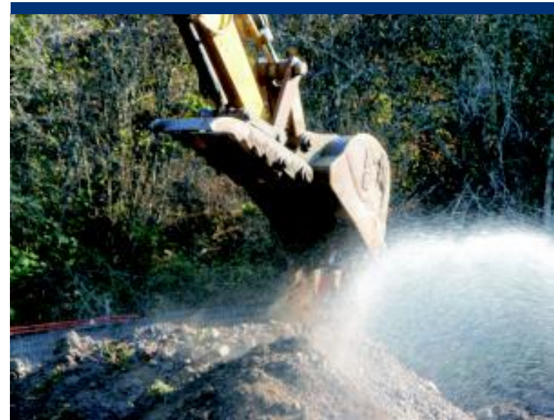
Photo 8 Dust suppression during excavation of contaminated fill.
