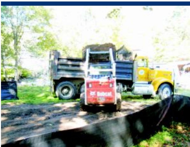
Photo 15 Loading truck with contaminated fill at 256 2nd Street.
