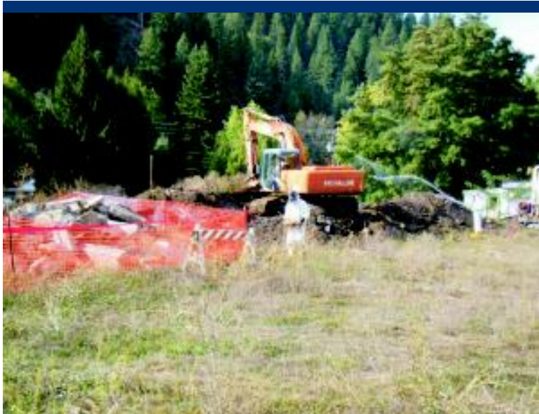
Photo 9 ERRS prepares contaminated fill stockpile at 14228 Highway 12 and recovers ACP.
