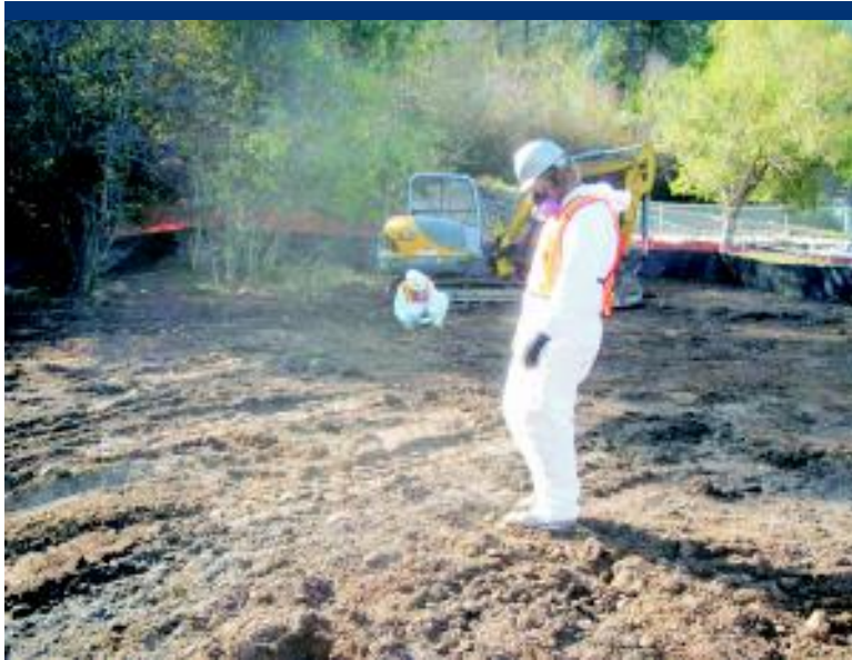
Photo 17 START collects soil composite sample following excavation of contaminated fill at 12586 Hartford Avenue.
