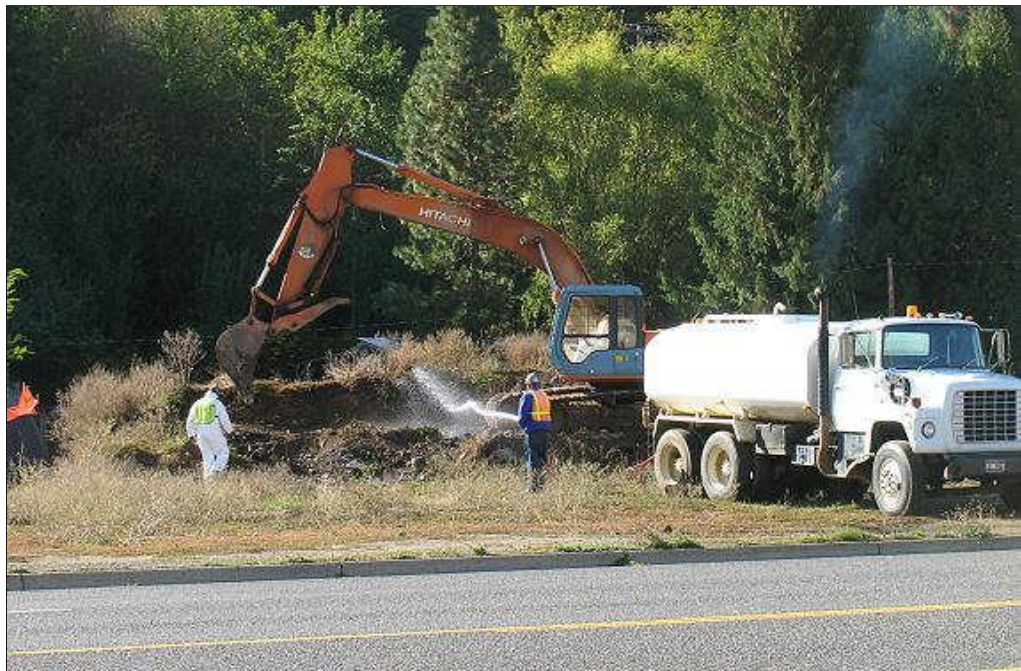
Crews are working on this site along U.S. Highway 12 to remove fill that is contaminated with asbestos fibers.
