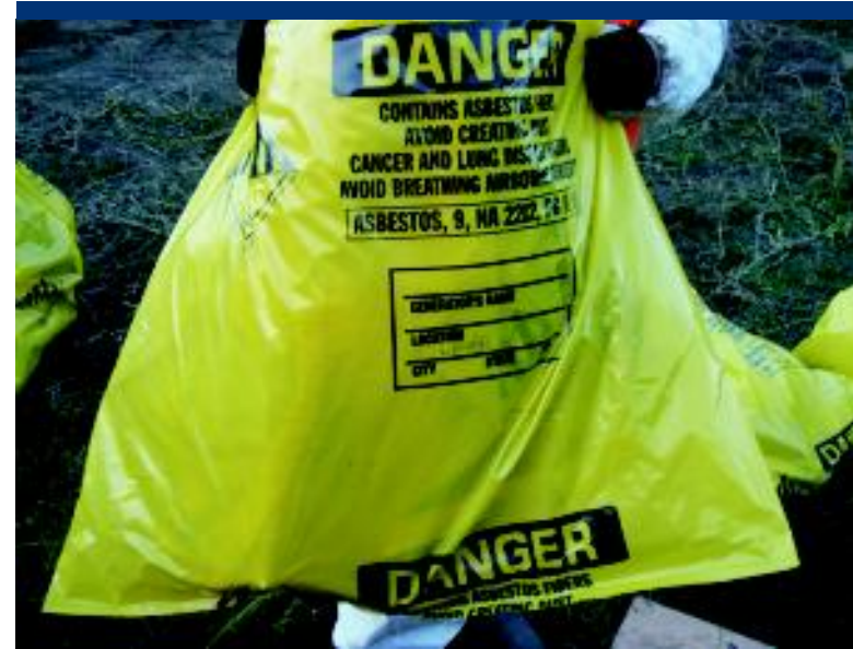
Photo 22 ACP in asbestos waste disposal bags for off-site disposal.
