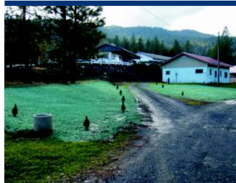
Photo 26 Hydroseed over top soil backfill at 131 122nd Street.
