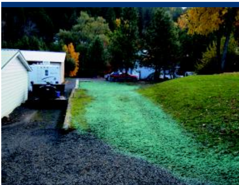
Photo 27 Hydroseed over top soil backfill at 12252 Indio Avenue.
