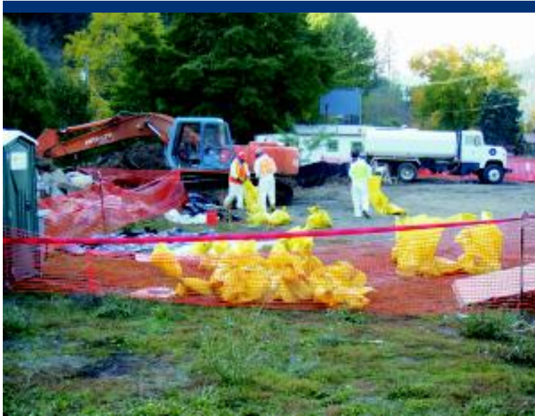
Photo 21 ERRS places recovered ACP into asbestos waste disposal bags.
