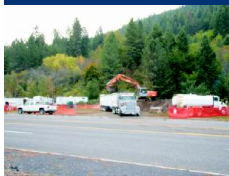
Photo 10 Overview of 14228 Highway 12 staging location; ERRS loads contaminated material into truck and pup.
