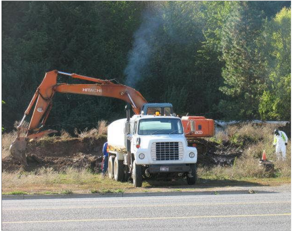
Photos: Second--Signs are posted to warn people about the hazard. Third--Works wear special protective gear. Fourth--Water is sprayed on the area to suppress dust that may carry the fibers as they are excavated.
