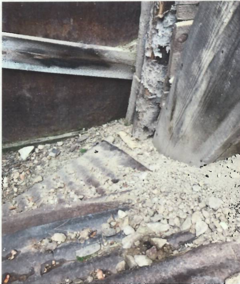
Entrance to magazine with degraded dynamite stick at base of wood post
