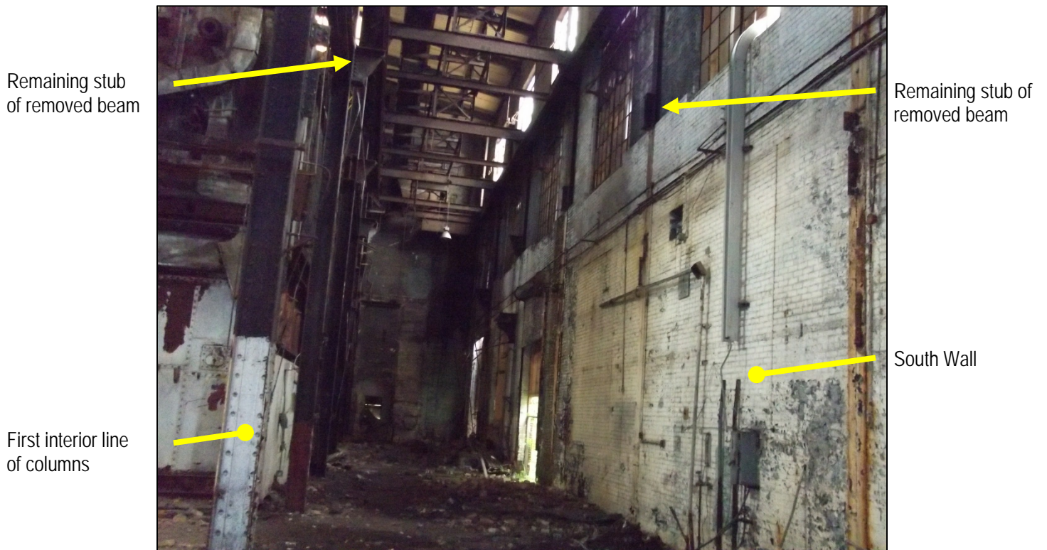
Photo 4: Removed beams in south building wall to first interior line of columns
