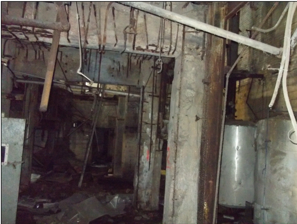
Photo 2: Exposed steel in beams and columns supporting the first floor.
