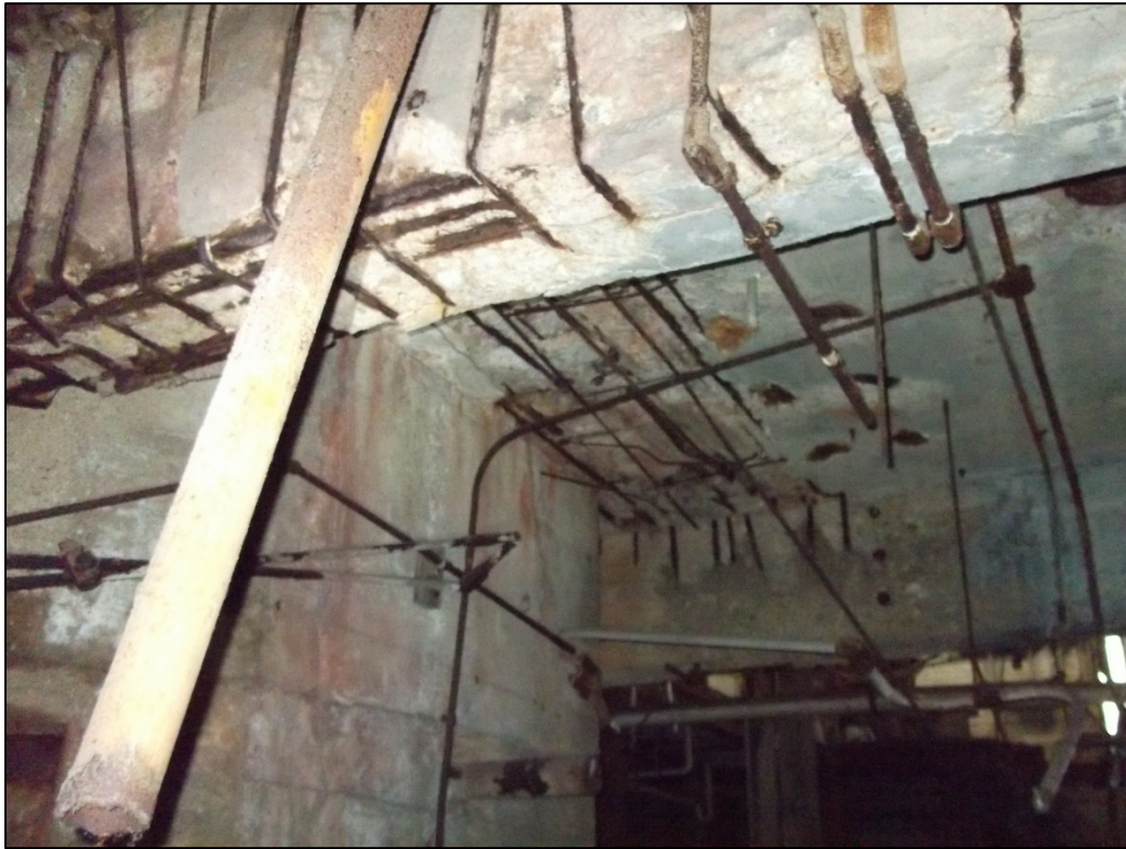
Photo 3: Exposed steel in beams and slab supporting the first floor.
