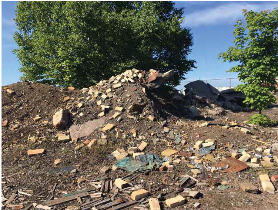
Photograph 2: WP-02 containing fire brick, metal, wood, concrete, and old appearing debris mixed with soil. Photograph by J. Chrestensen, July 20, 2016.
