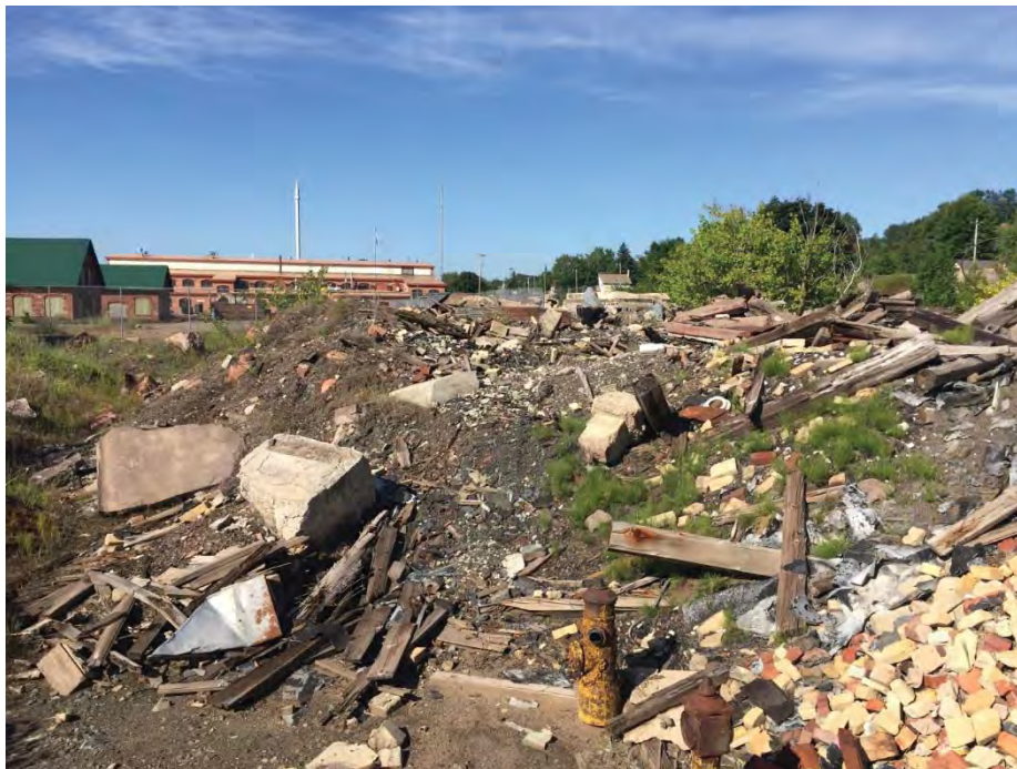
Photograph 28: WP-28 containing concrete, wood, metal, soil, fire brick, and transite pieces. The material appears older in nature. Photograph by J. Chrestensen, July 20, 2016.
