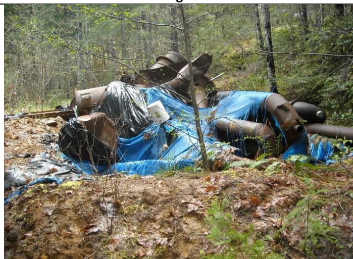
Metal Debris in non-Engineered Repository, Note Torn Visqueen Liner
