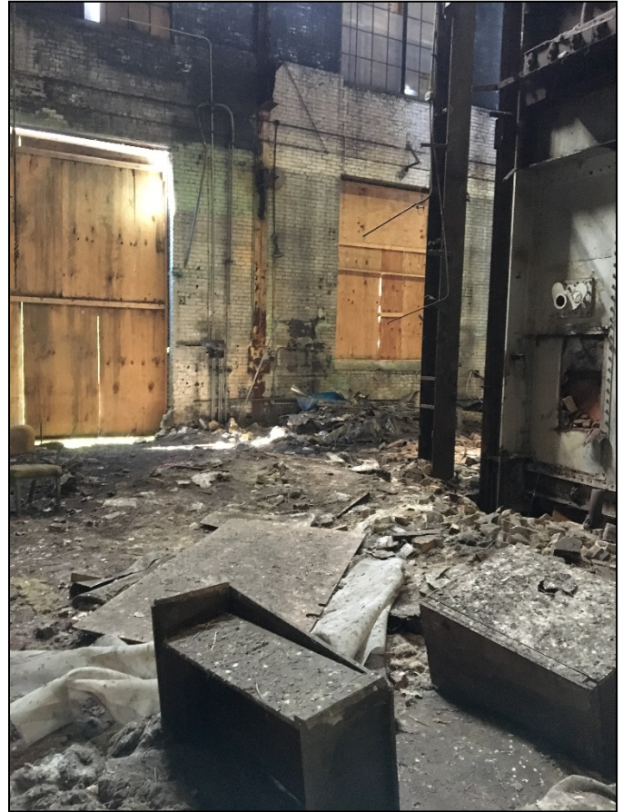
Loose asbestos is strewn about the inside of the building.
