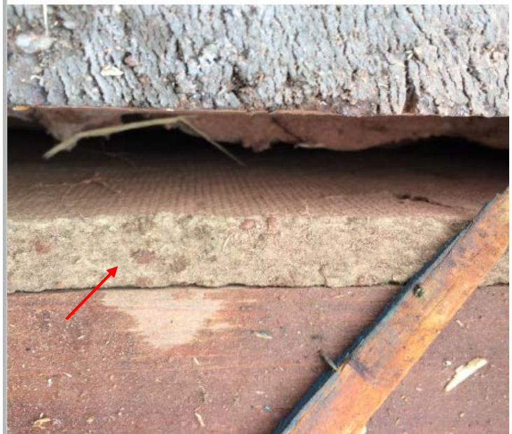
Sill Materials - copper flashing with fiber and adhesive
