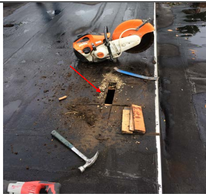
Roofing Materials- rubber, tar, and particle board material
