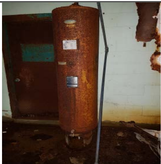
Air dryer inside chemical make-up room of basement
