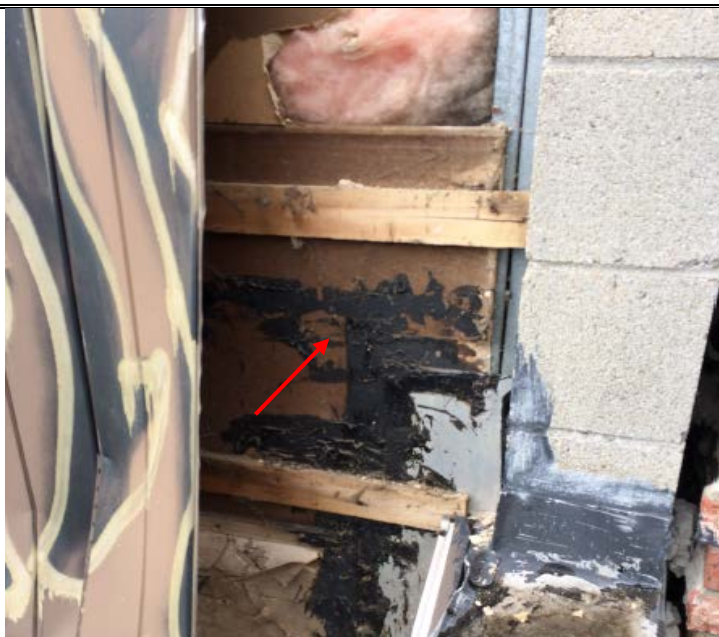
Sill Materials - fiber and adhesive
