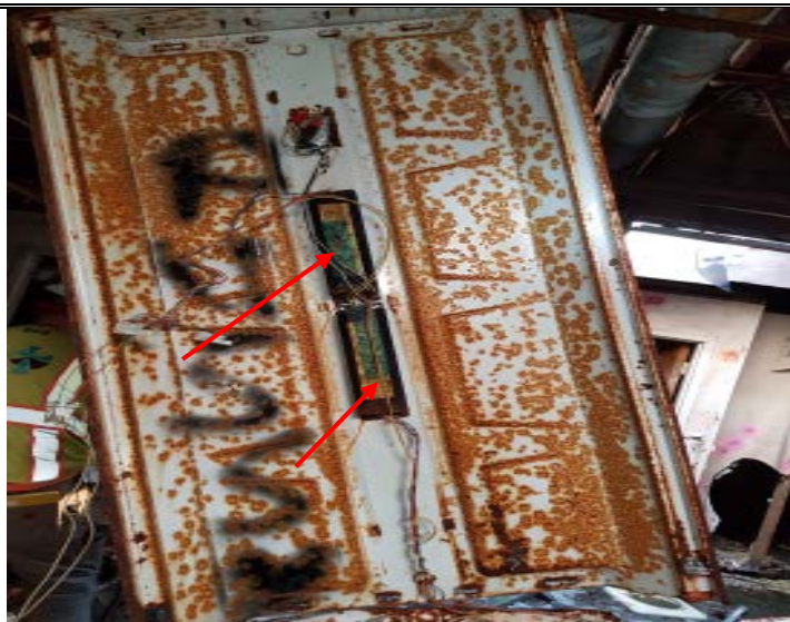
Ballasts attached with Fluorescent tube fixtures Location: throughout building Type: Universal waste.
