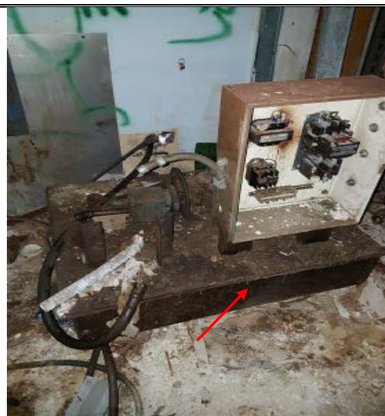
Pump having hydraulic Oil in trash room of ground floor Volume of oil: 25 gallons (worst case scenario)
