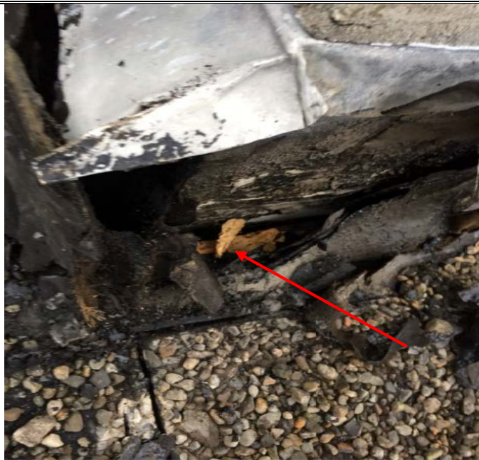
Interior Roof Edge Flashing Materials - tar material with wood, concrete, metal, and shingles
