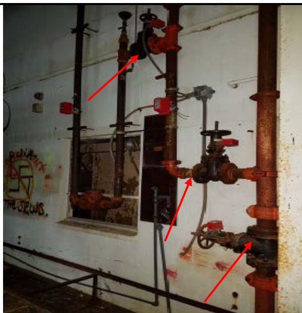
Gaskets between Flanges Total number of gaskets: 5
