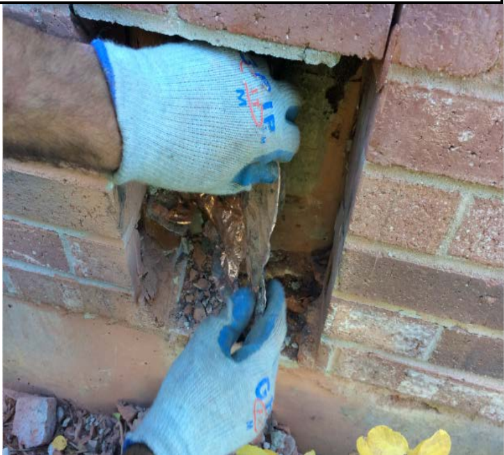
Block Wall Materials - loose insulation from block wall bay
