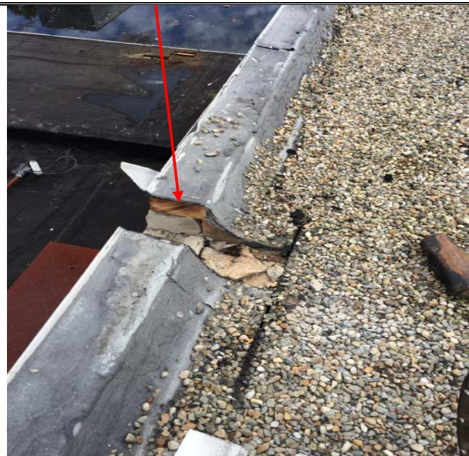
Equipment Flashing Materials - rubber, black tar material
