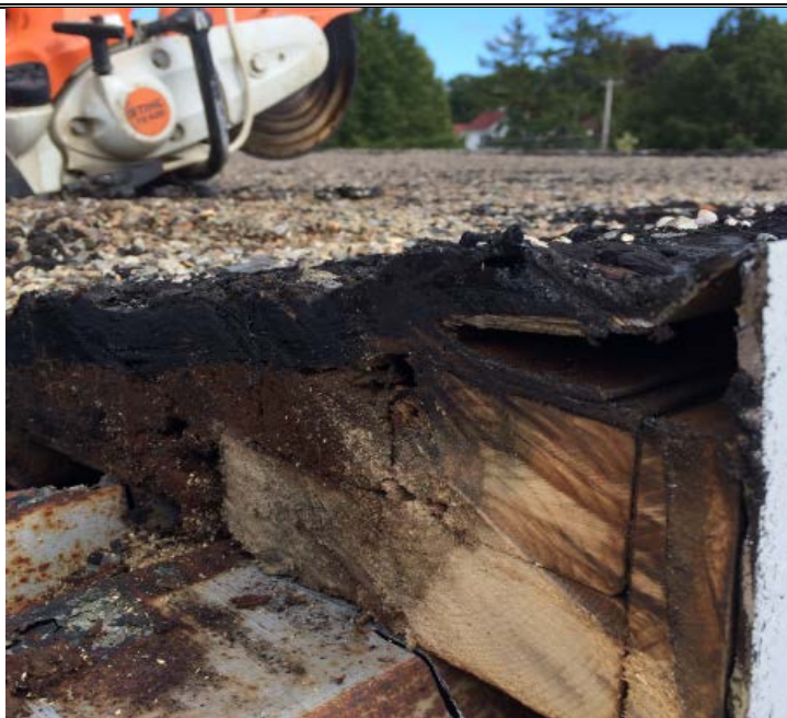
Roofing Materials- rubber, with tar, shingle, and particle board material
