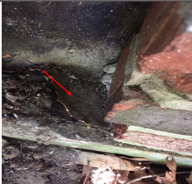
Block Wall Materials - loose insulation from block wall bay
