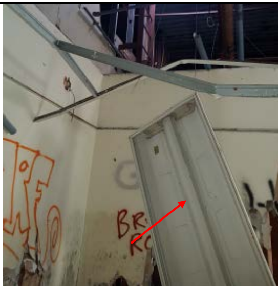
Fluorescent tube with fixtures Location: throughout building, about 50% tubes are broken Type: Universal waste.
