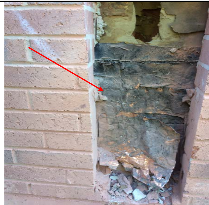
Block Wall Materials - loose insulation from block wall bay
