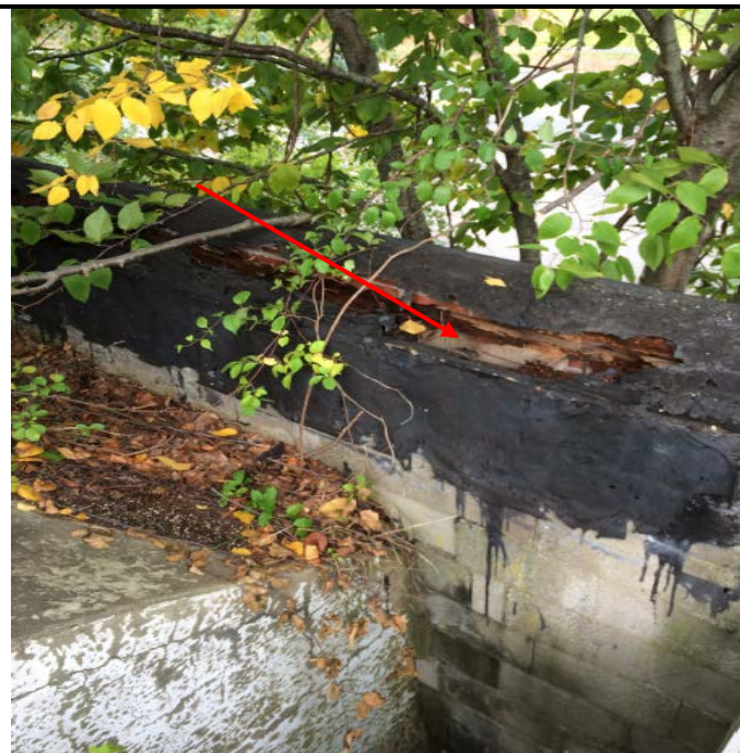
Wall Materials - tar material with shingles and drywall
