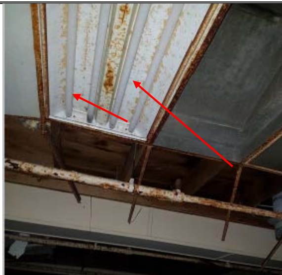
Fluorescent tube with fixtures Location: throughout building Type: Universal waste.
