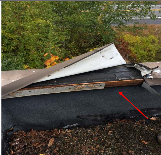
Roofing "Cap" Materials- rubber, tar with stone , and particle board material
