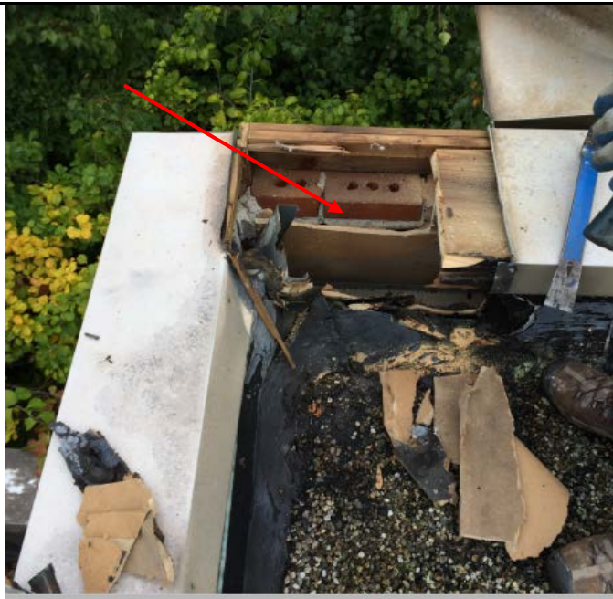
Interior Roof Edge Flashing Materials - tar material with shingles, drywall, and fibers
