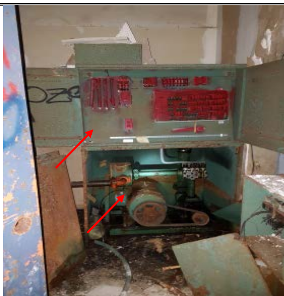
Elevator reservoir having hydraulic Oil in trash room of ground floor Volume of oil: 40 gallons (worst case scenario)
