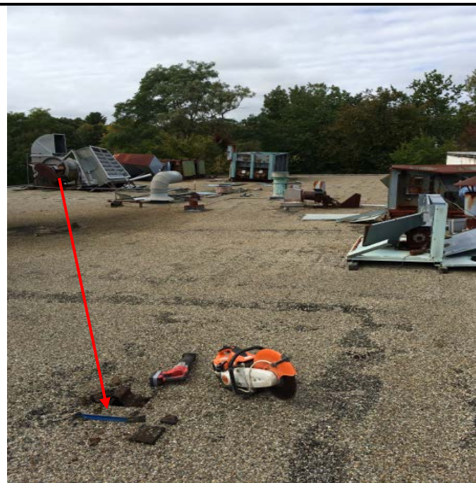
Roof Edge Flashing Materials - tar material with wood, concrete, metal, and shingles
