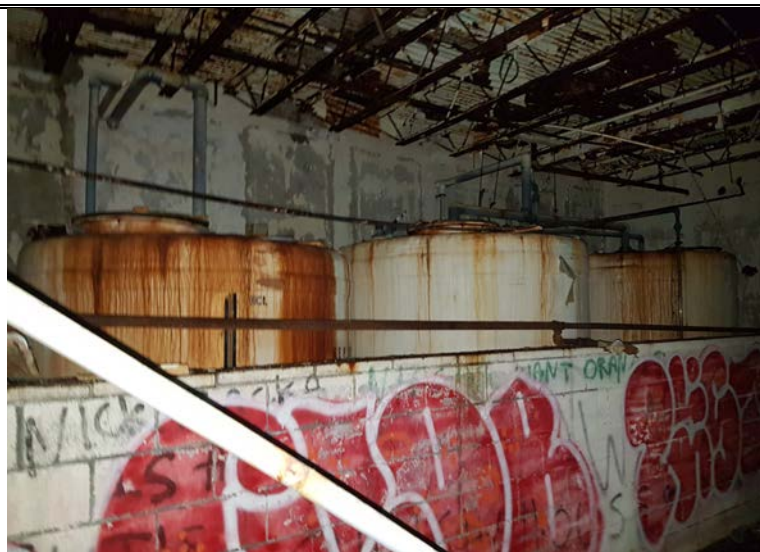
Three Poly tank with 1 inch of conc. acid pH of 1 at ground floor of new building (Location #7). Each Tank Volume ~ 7500 gallons Volume of acid~ 150 gallons (worse case)
