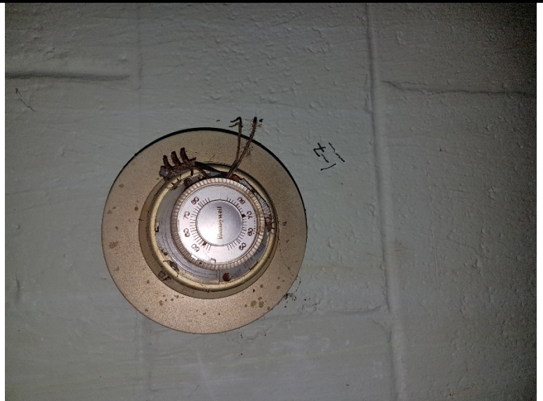
Wall mounted Mercury Thermostat
