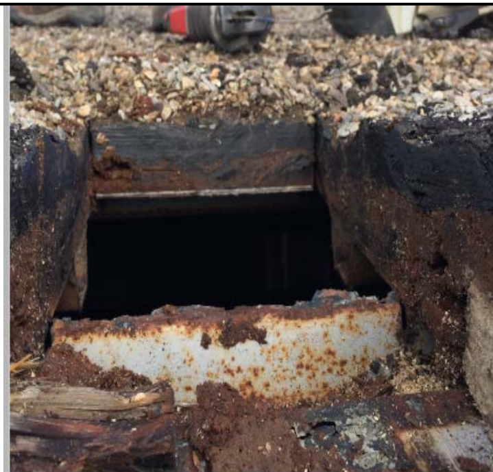
Roofing Materials- rubber, tar with stone , and particle board material
