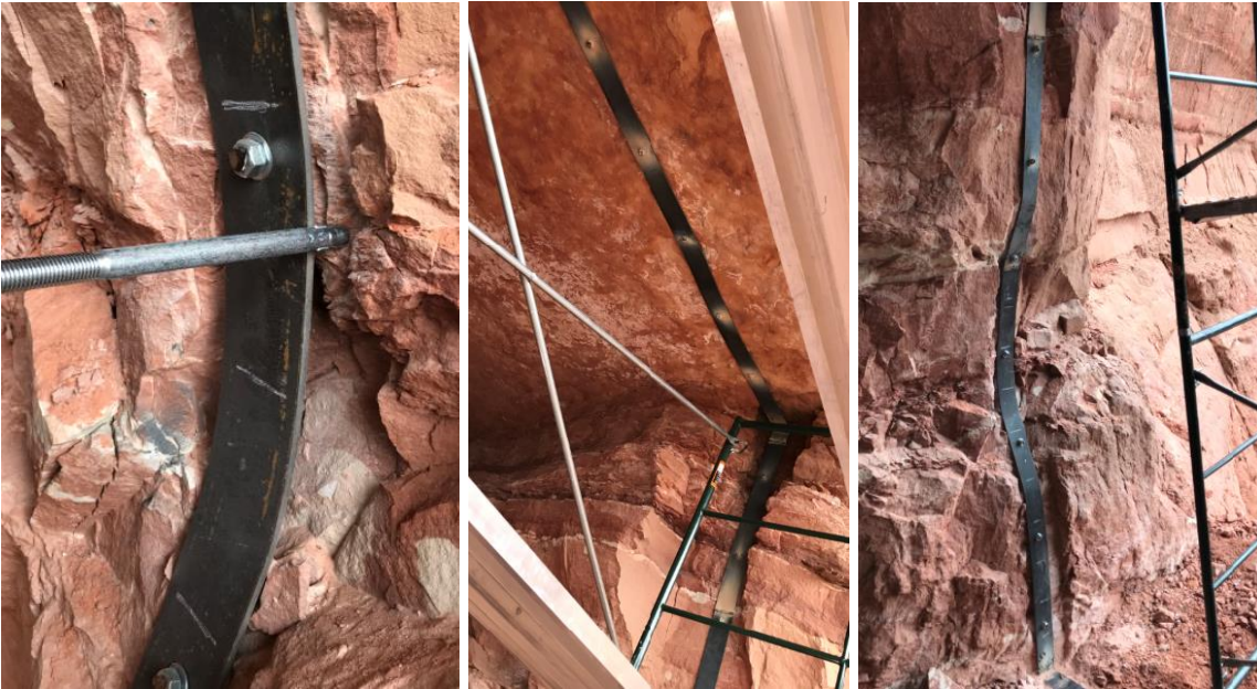
Anchor bolts (size: 5/8 – 11 x 12) installed into bed rock.
