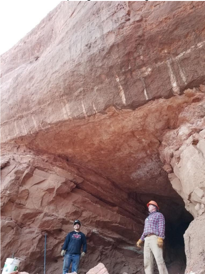
Natural rock drip edge shown, might not need drip panel.
