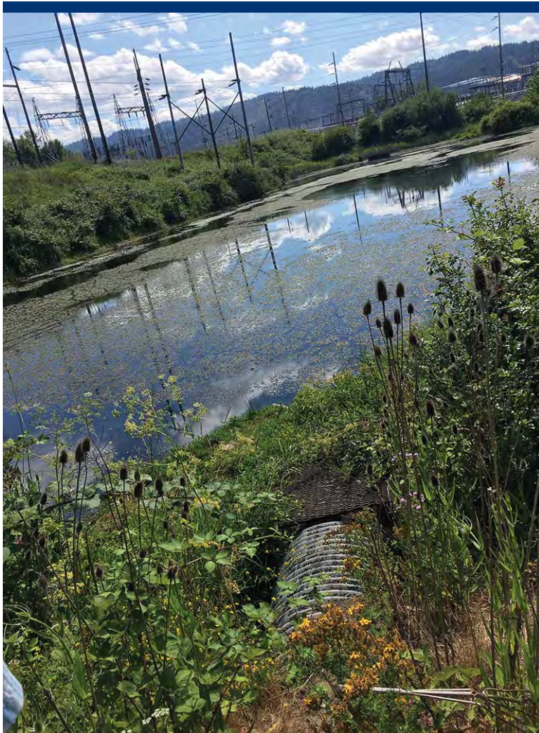
Photo 31 Inlet to culvert draining pond. Inlet approximately 1 to 1.5 feet above current pond level.
