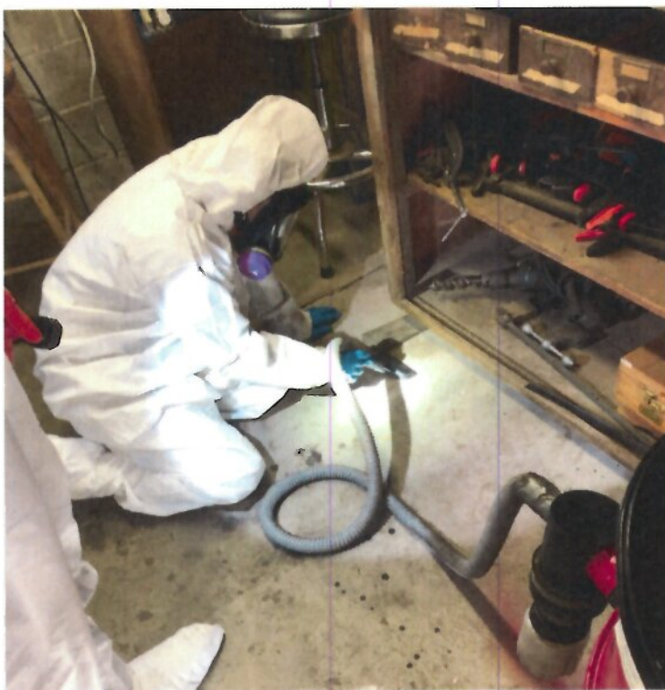
ERRS contractor recovering mercury with a Merc-Vac recovery unit.
