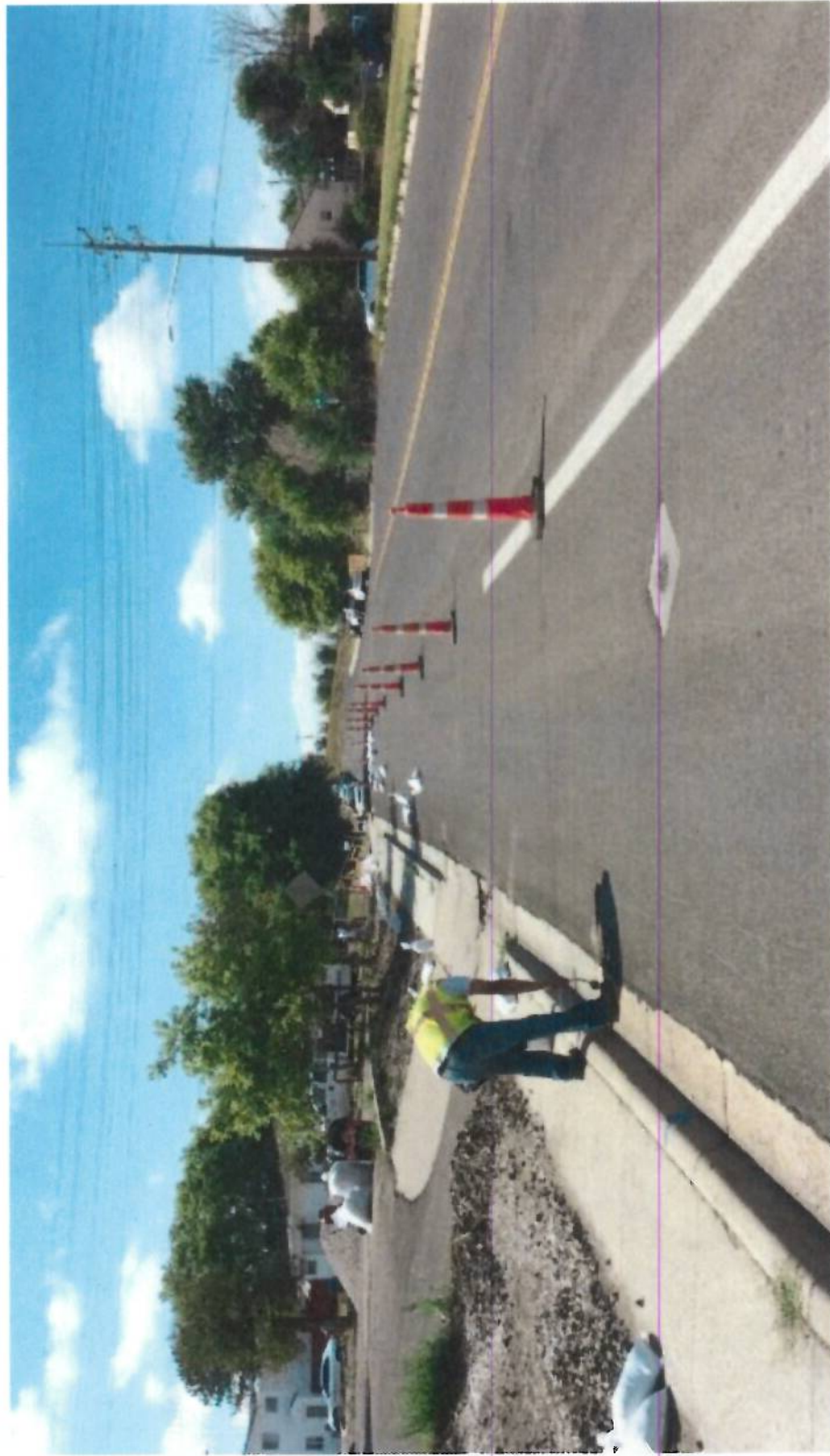
Figure 4. START contractor screening the street for mercury vapors after the removal
