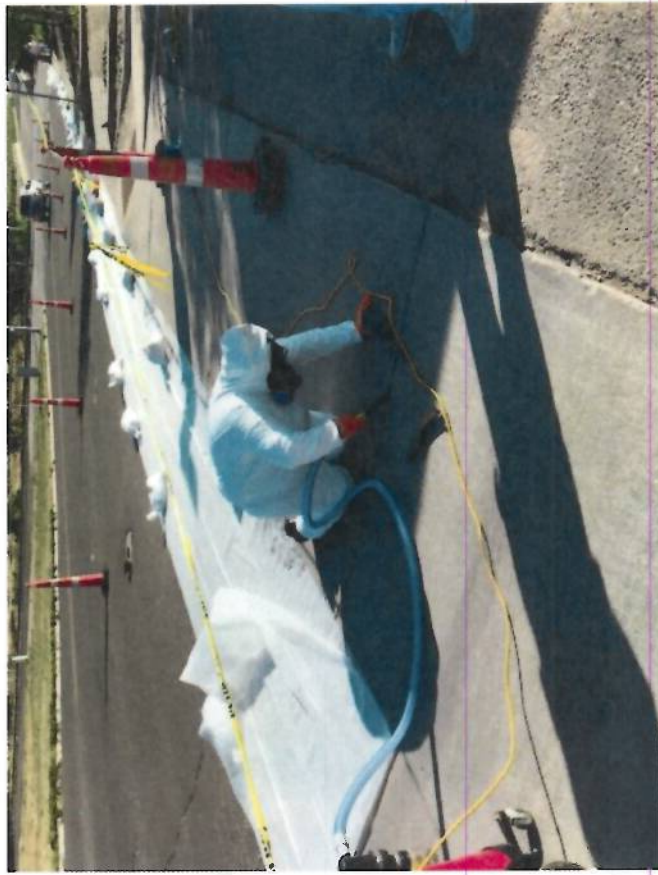
Figure 2. ERRS crew vacuuming visible mercury
