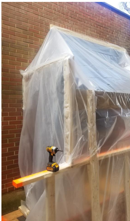
Photograph Description: Containment area to prevent release of asbestos fibers during ACM removal. Photographer: START
