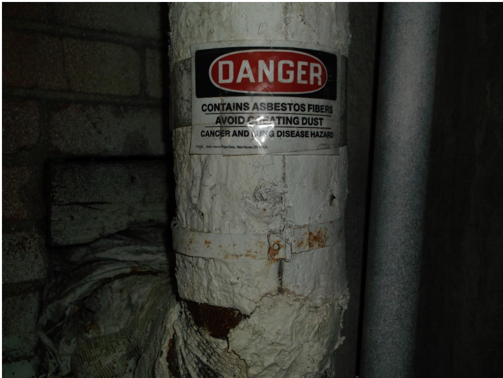
Photograph Description: Damaged pipe wrap labeled with asbestos signage located in the machine room Photographer: START
