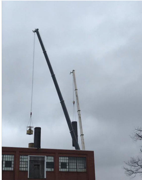
Photograph Description: Dismantling of the metal stack. Photographer: START
