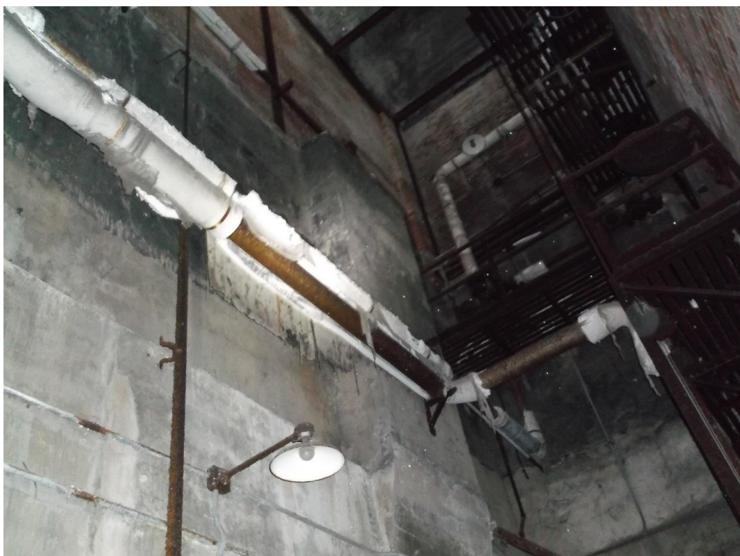
Photograph Description: Damaged pipe wrap located in the lower boiler room Photographer: START
