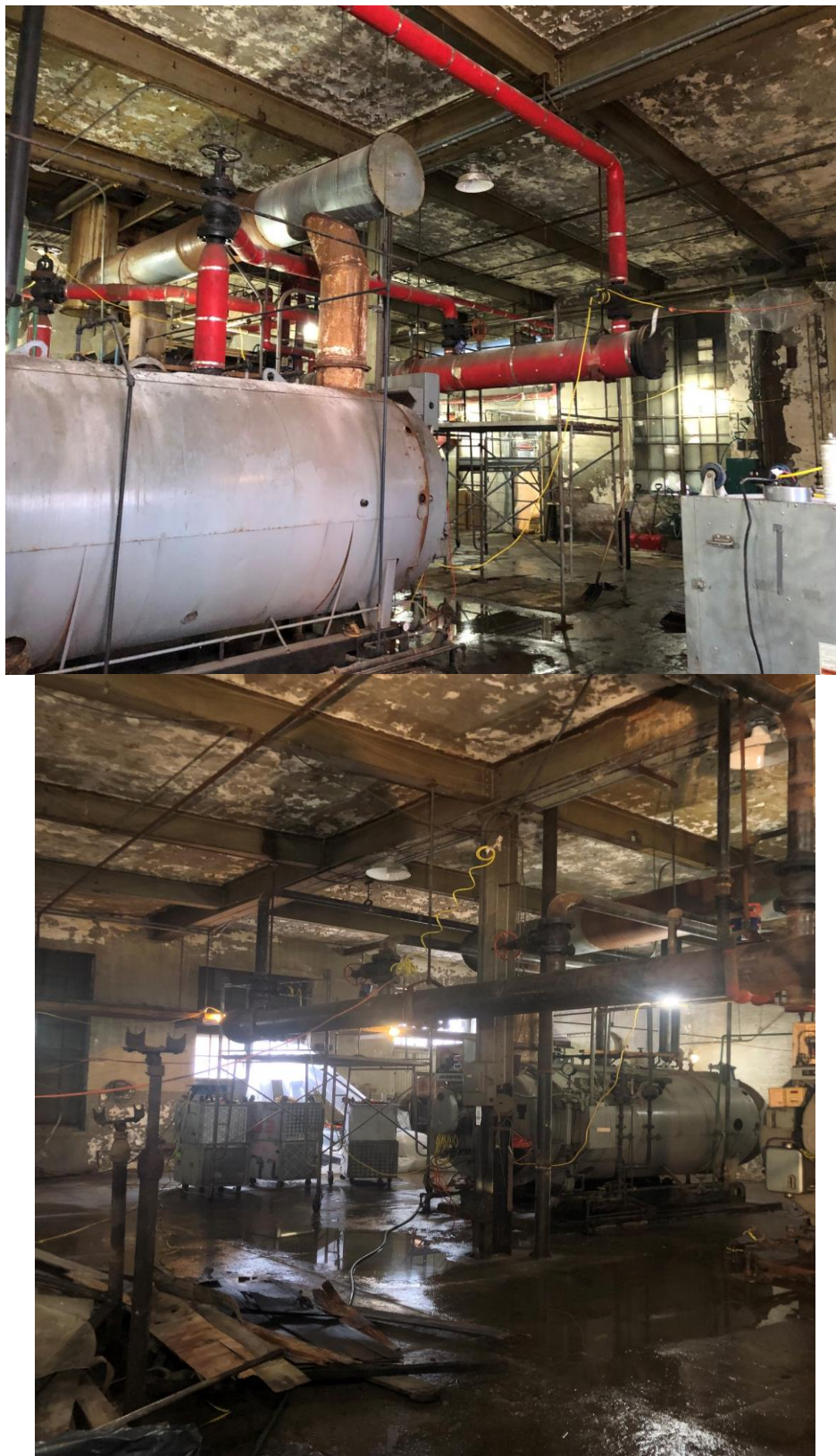
Photograph Description: Before and after ACM removal in the upper boiler room. Photographer: START
