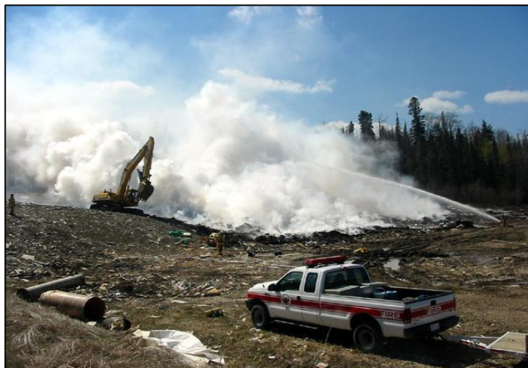
Best Practice: Excavator used to remove burning waste combined with continual water application.
