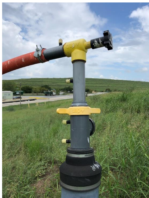
Figure 9. LFG Wellhead
