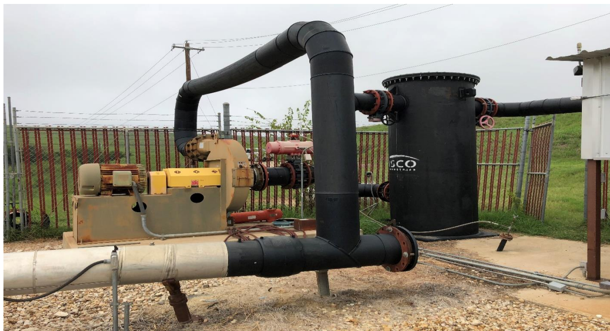
Figure 10. Typical LFG Skid
