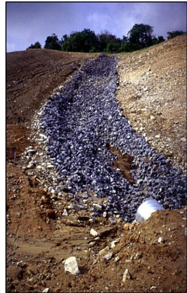
Best Practice: Proper stormwater controls minimize erosion.
