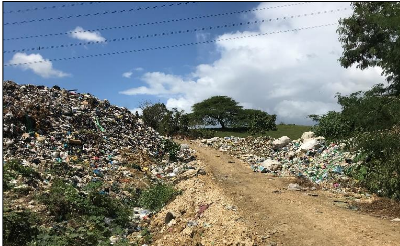
Section of the current access road showing exposed waste and poor drainage.
