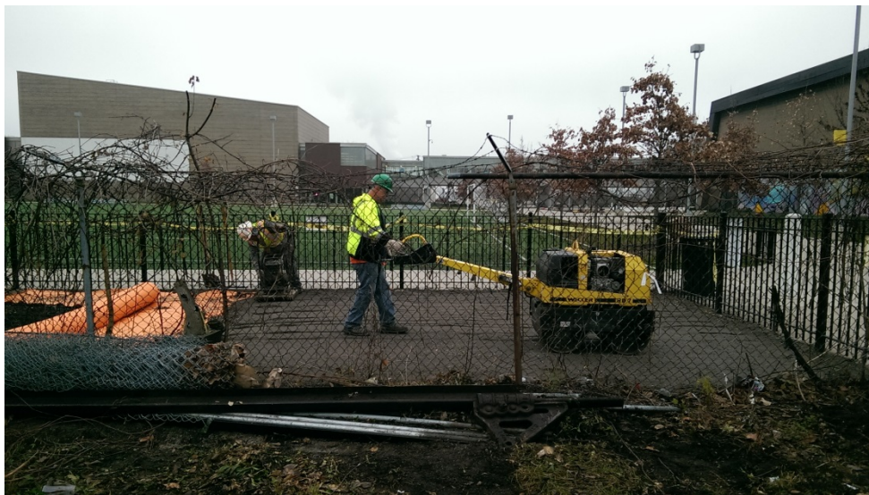
Photo 18 - Installing Geotextile Fabric and Gravel Area 1
