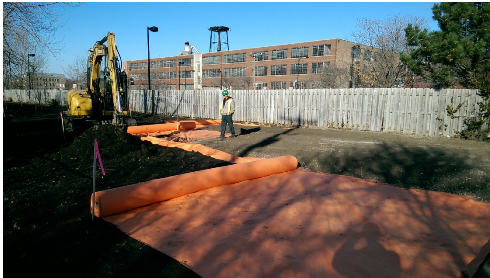
Photo 20 - Installing Geotextile Fabric and Gravel Area 2
