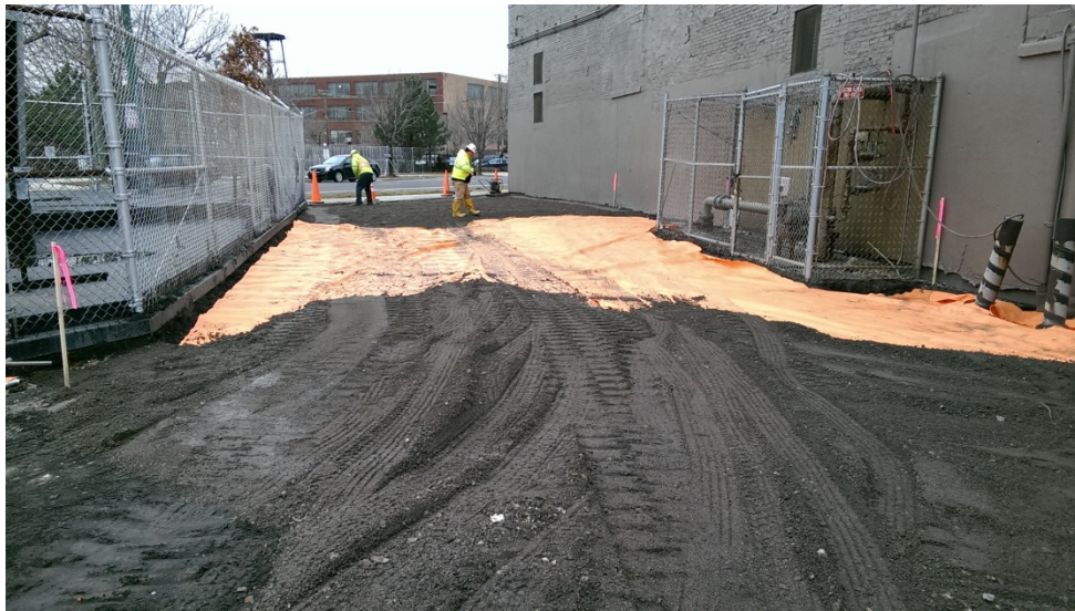
Photo 26 - Installing Geotextile Fabric and Gravel in Area 4
