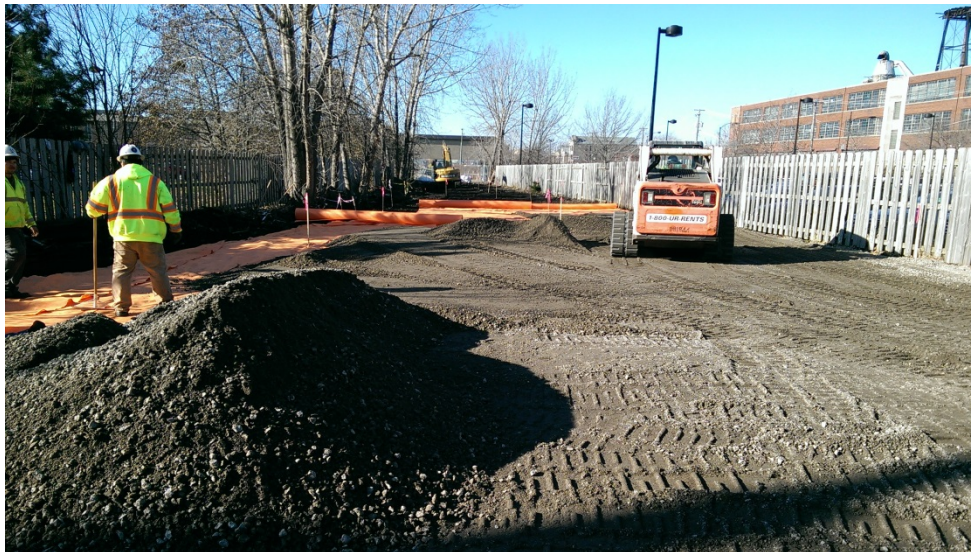
Photo 21 - Installing Geotextile Fabric and Gravel Area 2
