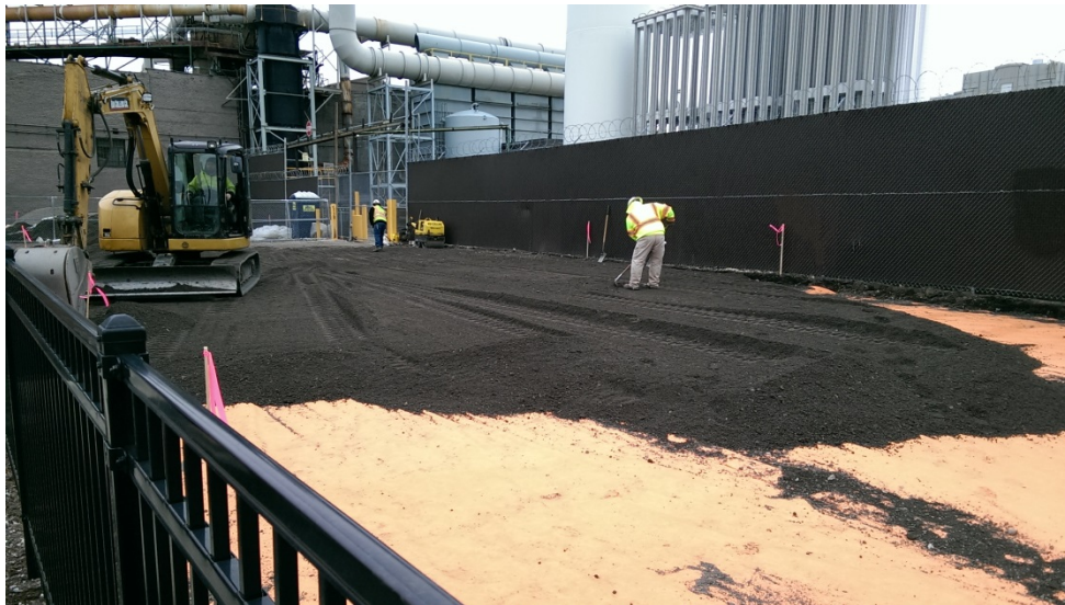
Photo 28 - Installing Geotextile Fabric and Gravel in Areas 6 and 7
