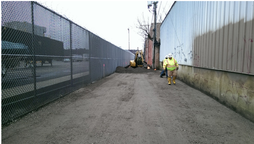
Photo 29 - Installing Geotextile Fabric and Gravel in Areas 8 and 9
