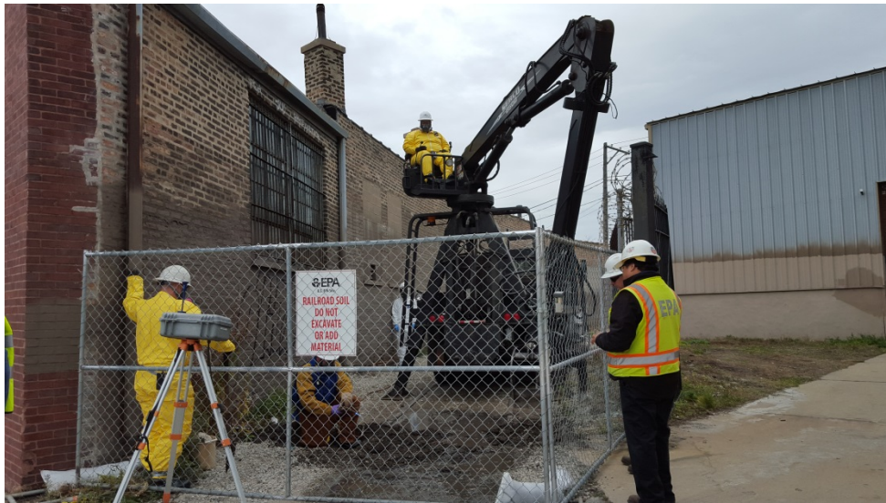
Photo 7 - Rail Removal Area 10 with Perimeter Air Monitor
