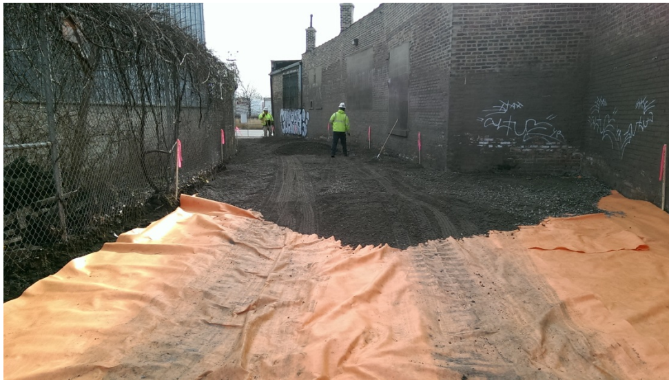
Photo 24 - Installing Geotextile Fabric and Gravel in Area 10
