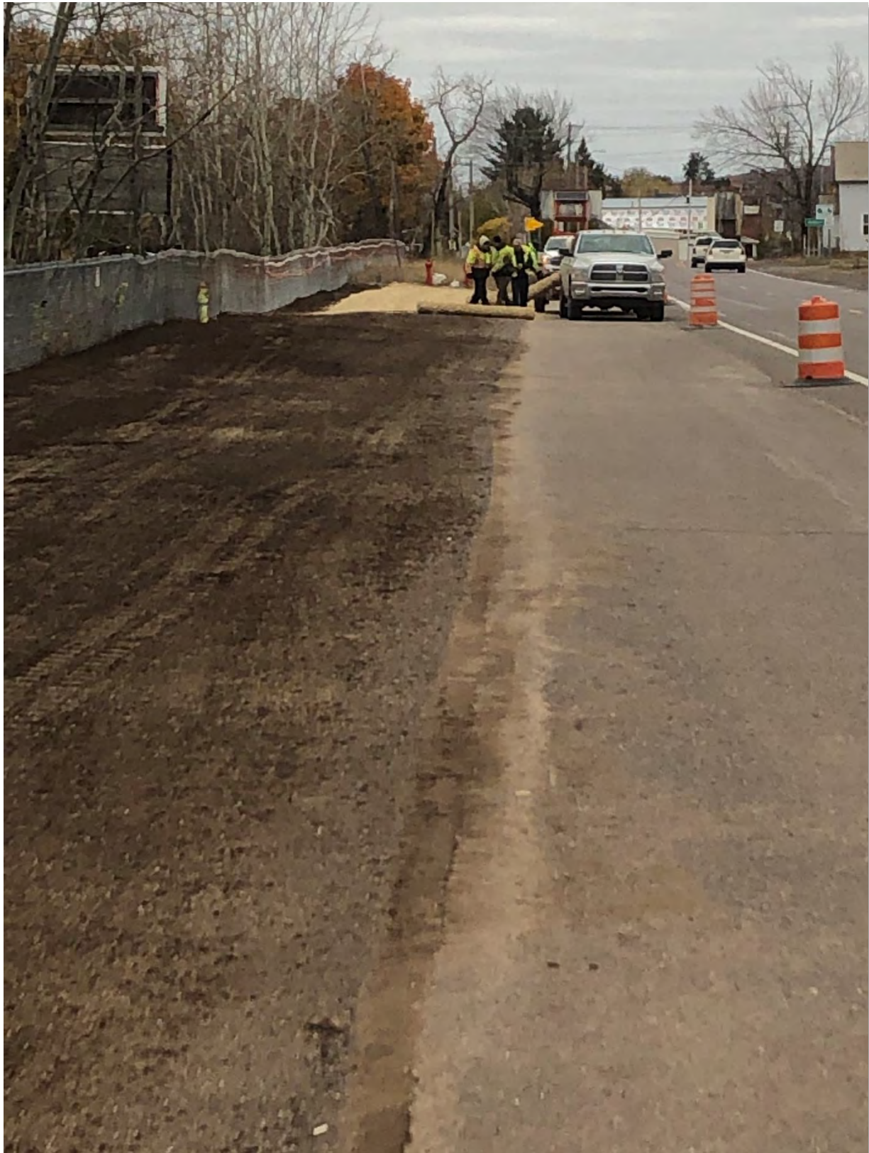
Photo 5: Installation of Mulch Blankets
