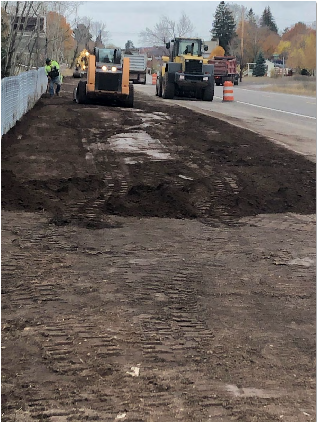
Photo 3: Placement of Topsoil
