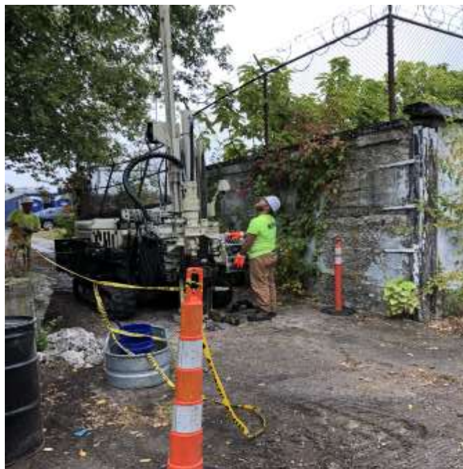
EPA contractors used a Geoprobe machine to install monitoring wells near the site.
