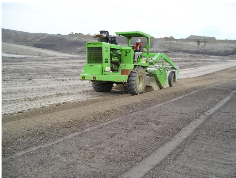
Figure 8: Processing Liner Soil to Control Clod Size
