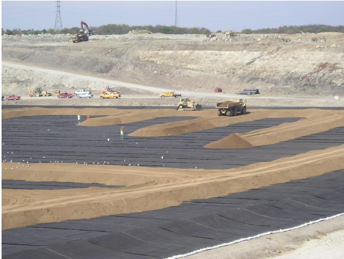
Figure 24: Protective Cover Deployed in Fingers
