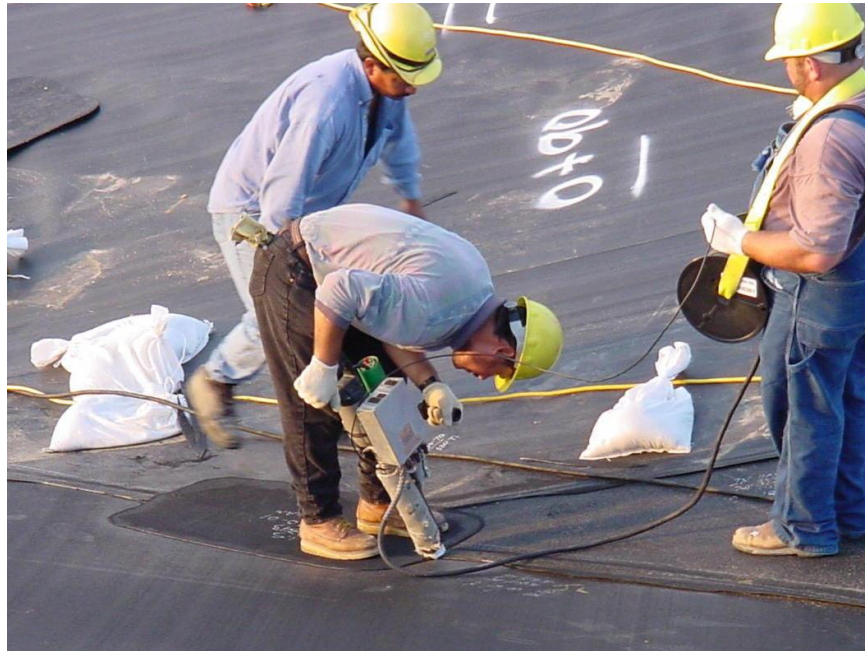
Figure 17: Extrusion Welding Geomembrane
