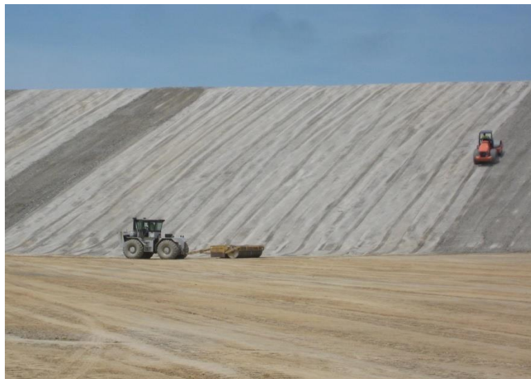
Figure 5: Parallel Lifts on 3:1 Side Slope
