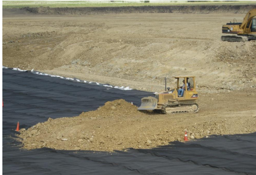
Figure 25: Protective Cover Placement Over Geotextile Using Traffic Cones as Thickness Indicators
