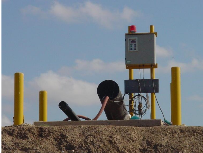
Figure 31: Leachate Riser Pipe and Distribution System
