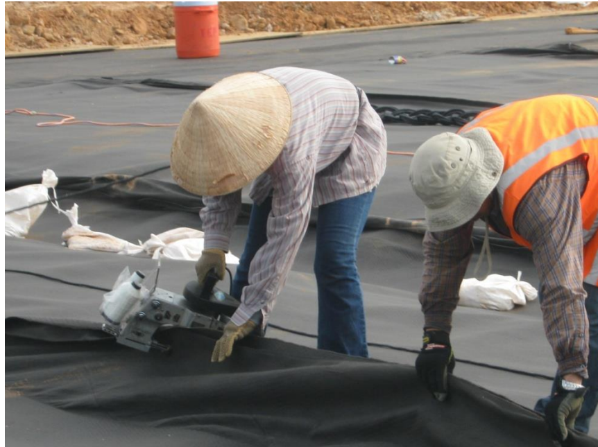
Figure 27: Sewing Geotextile
