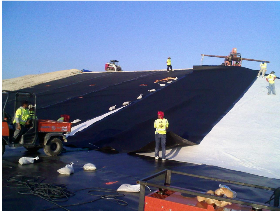
Figure 14: Geomembrane Deployment
