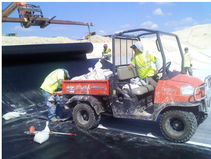
Figure 15: Low Ground Pressure All Terrain Vehicle on Geomembrane
