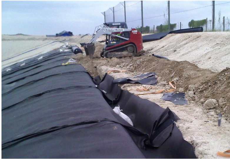
Figure 23: Anchor Trench being Backfilled with Soil
