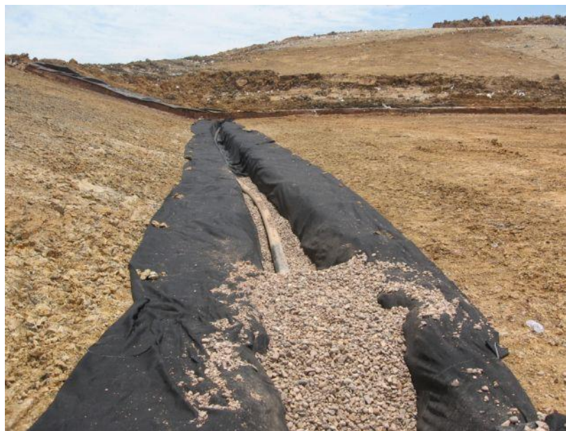
Figure 34: Dewatering Underdrain
