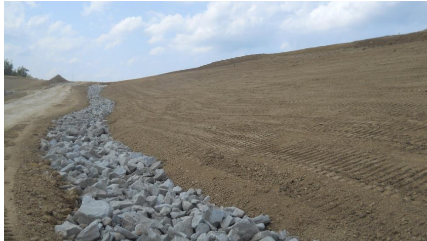
Figure 4: Stormwater Channel Along Perimeter of Landfill
