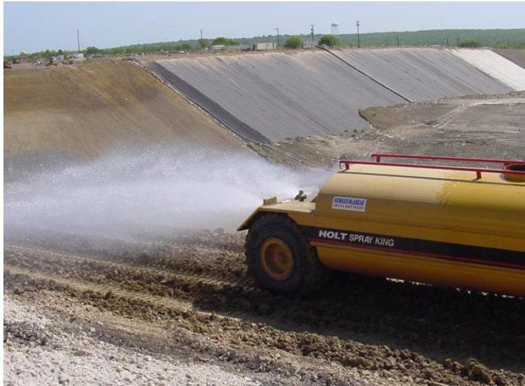
Figure 7: Hydrating Soil Liner
