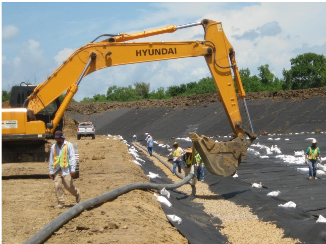
Figure 29: Leachate Collection Pipe Installation
