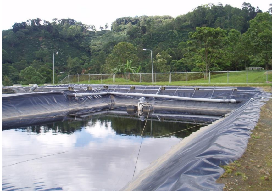
Figure 32: Lined Aerated Lagoon for Leachate Treatment
