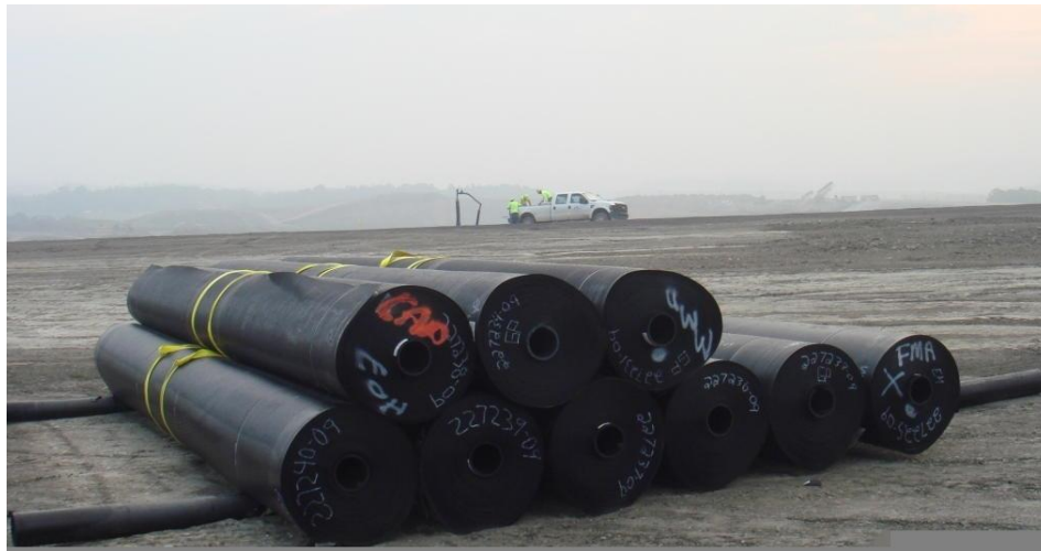
Figure 12: Geosynthetic Rolls of HDPE Liner Stored Properly
