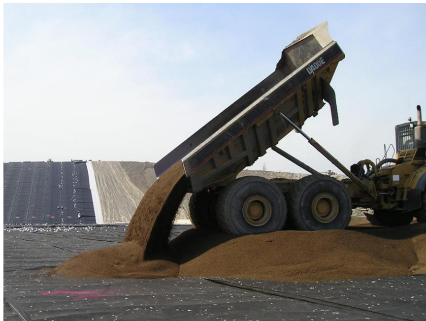
Figure 10: Protective Cover Soil
