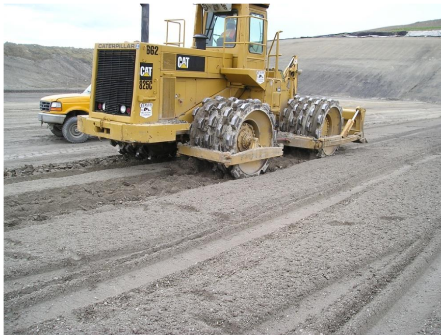
Figure 9: Compacting Soil Liner
