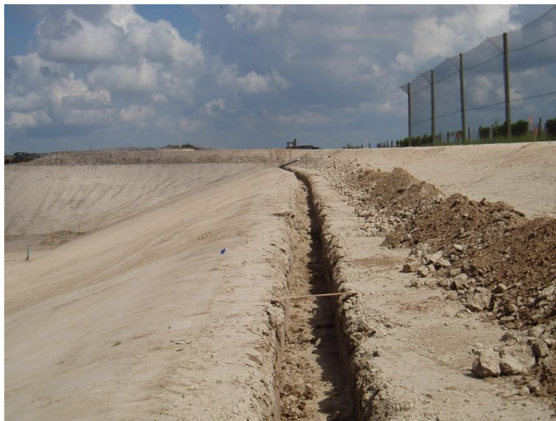
Figure 22: Anchor Trench During Excavation
