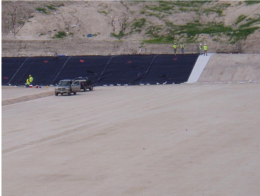
Figure 13: Prepared Subgrade
