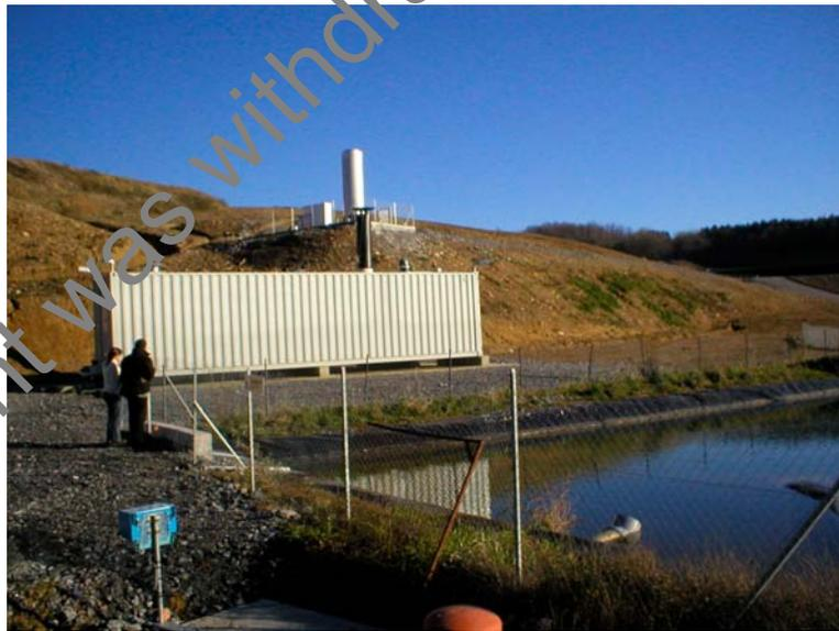
**Plate 2.3:** Typical configuration of a 2-stage RO plant with leachate lagoon, direct permeate discharge and concentrate re-infiltration (72 m<sup>3</sup>/d, landfill CSDU Pays des Graves, district Hautes-Pyrenees, Commune de Lourdes, France, commissioned 2004) (see Wachter 2005)
