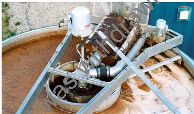
**Plate 2.6. The main DAF treatment tank at Arpley Landfill**
