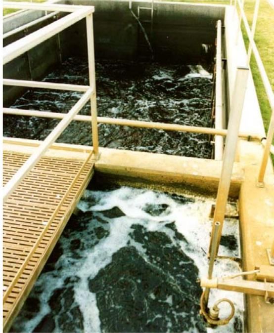
**Plate 2.7:** Typical reactor (35 m<sup>3</sup>) for contact with PAC in treatment of landfill leachate
