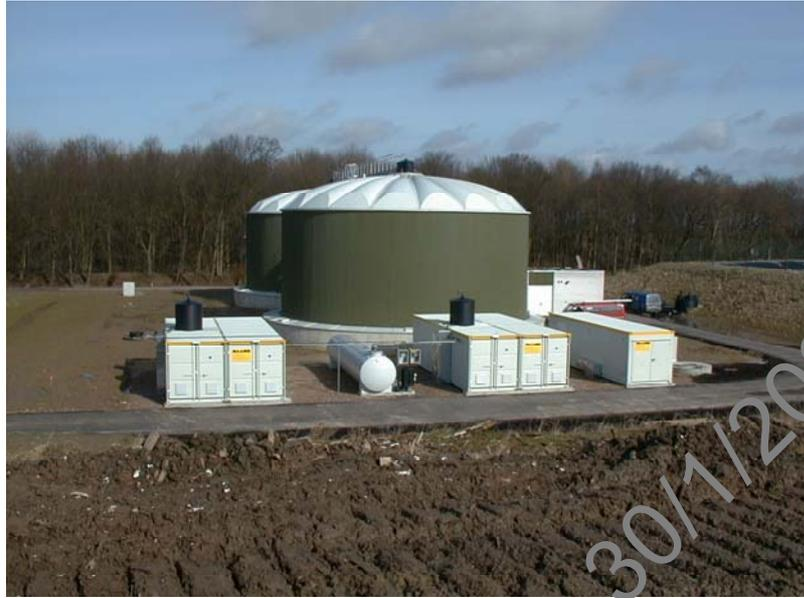
**Plate 2.2:** Typical configuration of two 2-stage RO plant with leachate tanks, direct permeate discharge and concentrate re-infiltration (350 m<sup>3</sup>/d, Niemark landfill, Luebeck Germany, commissioned 1999).
