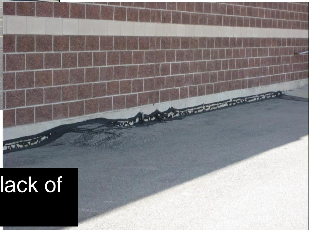
Settlement due to lack of compaction
