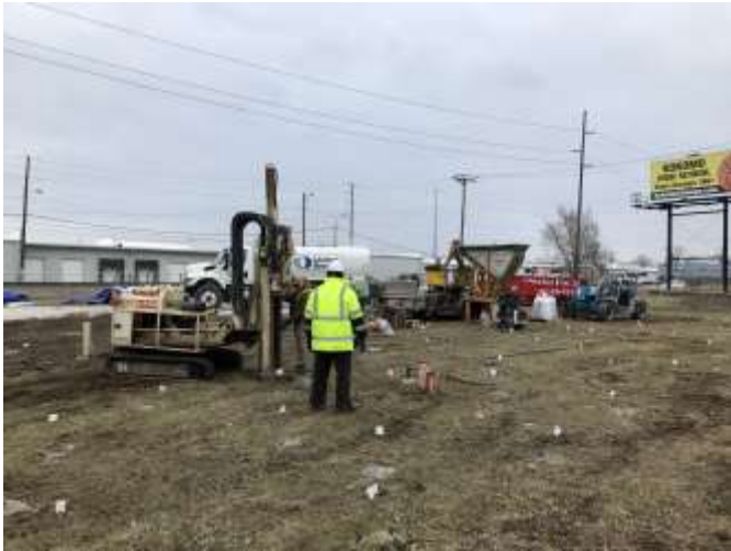
EPA contractors injecting Zero Valent Iron.
