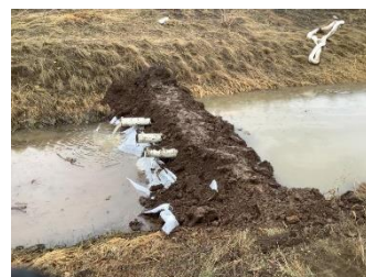
Earthen berm and underflow dam in the ditch that runs west of I-25.
