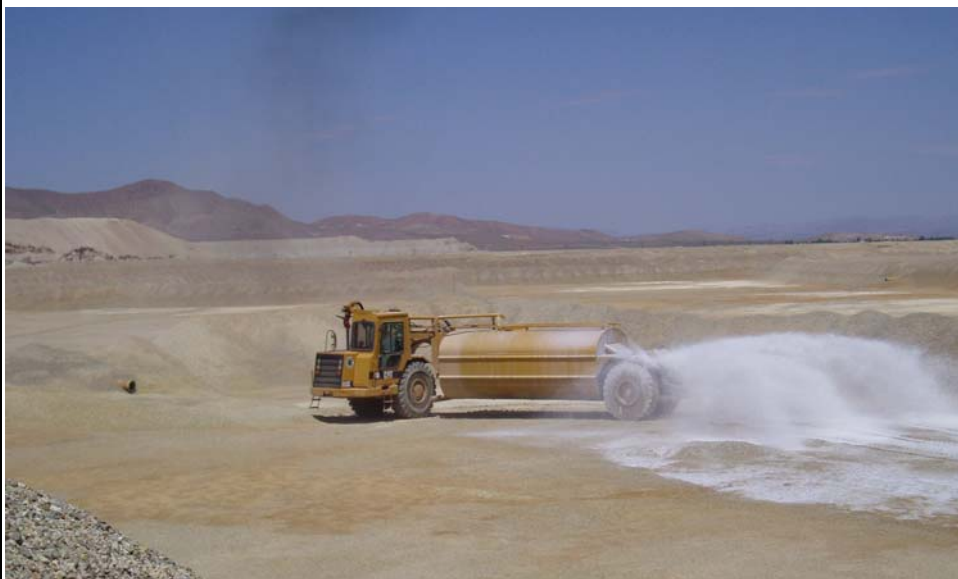
PHOTOGRAPH 7.: Water Truck applying soil sealant in small sulfide basin, Area S4. (Facing West)
