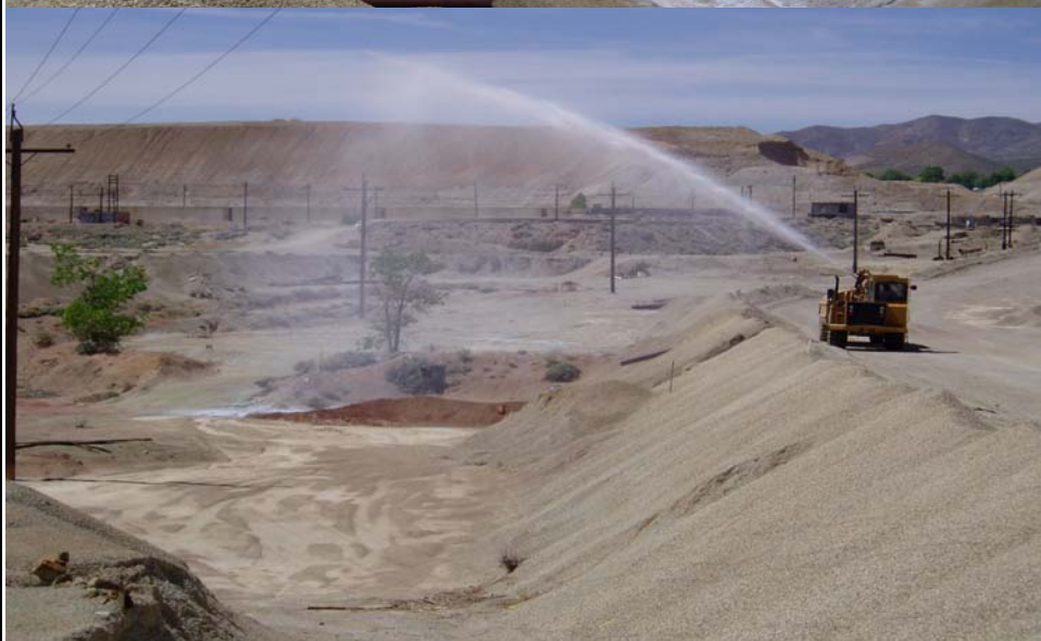
PHOTOGRAPH 20.: Application of soil sealant along east toe of road R12, Area R2. (Facing South)
