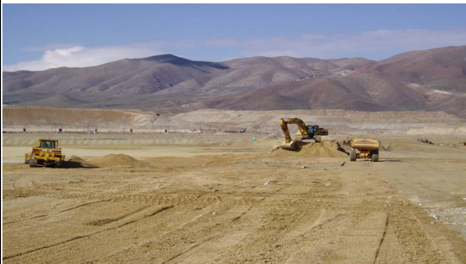
PHOTOGRAPH 1.: Excavator (center), dump truck (right), and bulldozer (left) spreading out VLT material in Area 1 as part of the capping activities. (Facing Southwest)
