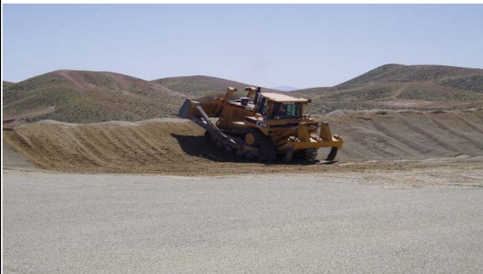
PHOTOGRAPH 4.: Bulldozer reworking loose sand material along the north edge of tailings pile, along interstate 95 ALT. (Facing East)
