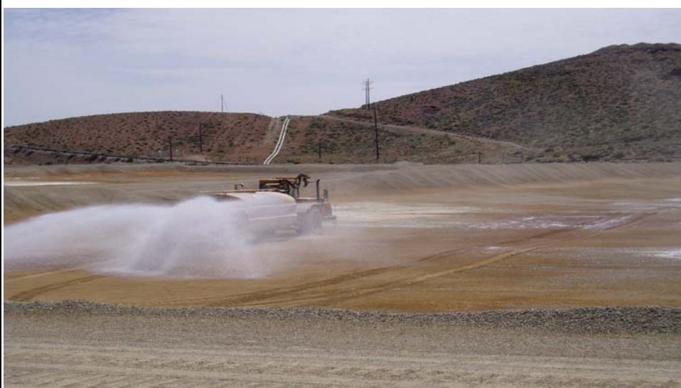
PHOTOGRAPH 6.: Water Truck applying sealant at the northwest corner of Area S3. (Facing Southeast)
