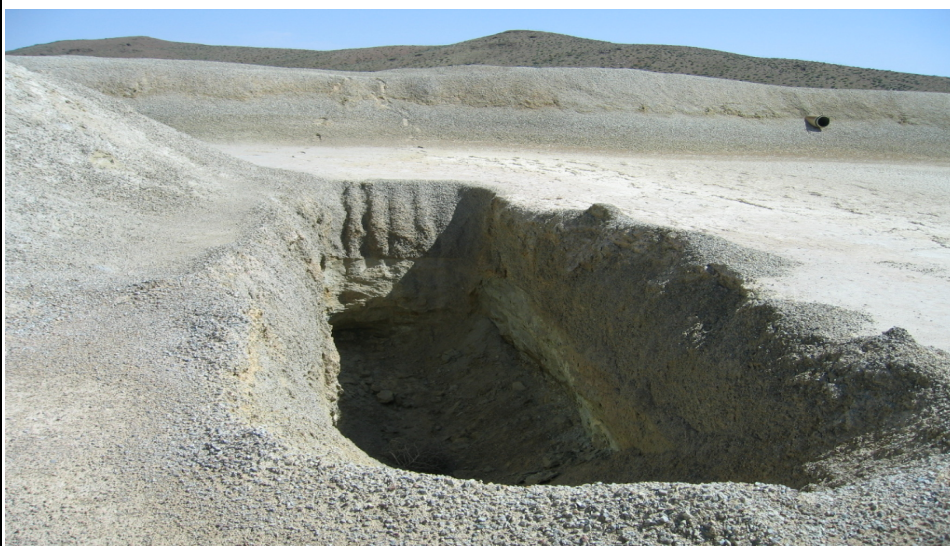
PHOTOGRAPH 5.: Photo taken standing in southernmost pond (Area S3) looking northeast at excavation in northwestern corner. This excavation shows at least 3 feet of VLT material on top of the pre-existing evaporation pond.
