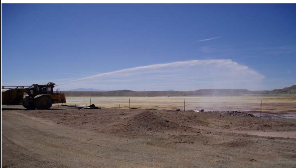
PHOTOGRAPH 15.: Application of soil sealant of north portion of North Evaporation Pond, Area S12. (Facing Northeast)
