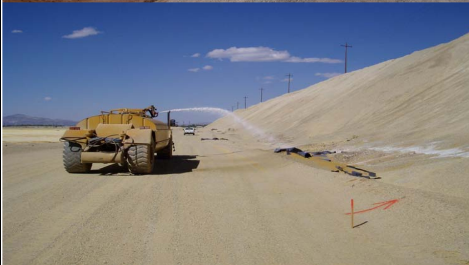
PHOTOGRAPH 17.: Application of Soil Sealant along west toe of Sulfide Tailings, Area S9. (Facing Northeast)
