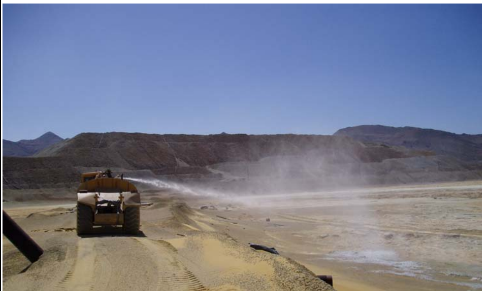
PHOTOGRAPH 13.: Application of soil sealant along west portion of Area S7. (Facing Northwest)
