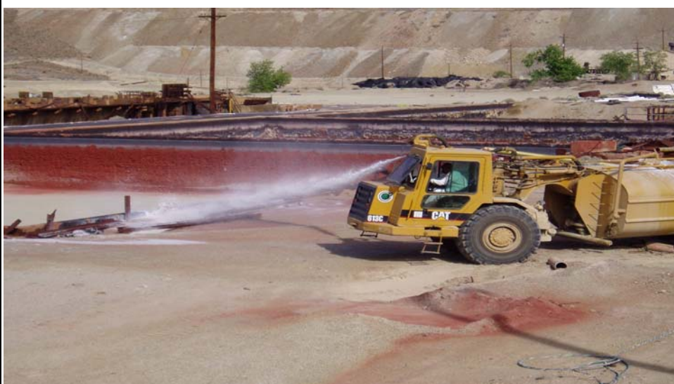
PHOTOGRAPH 12.: Application of Soil Sealant in Process Area S5. (Facing East)
