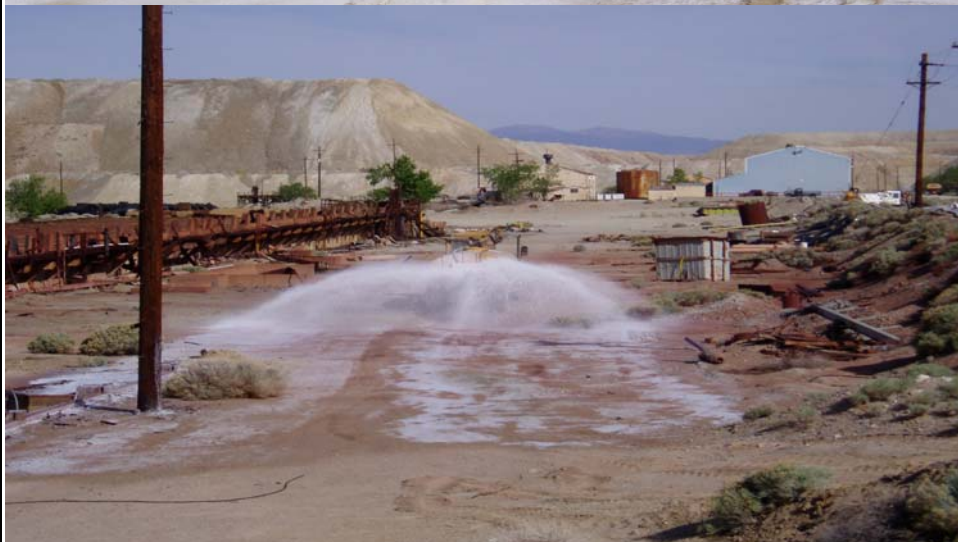
PHOTOGRAPH 11.: Application of Soil Sealant in Process Area S5. (Facing Southeast)
