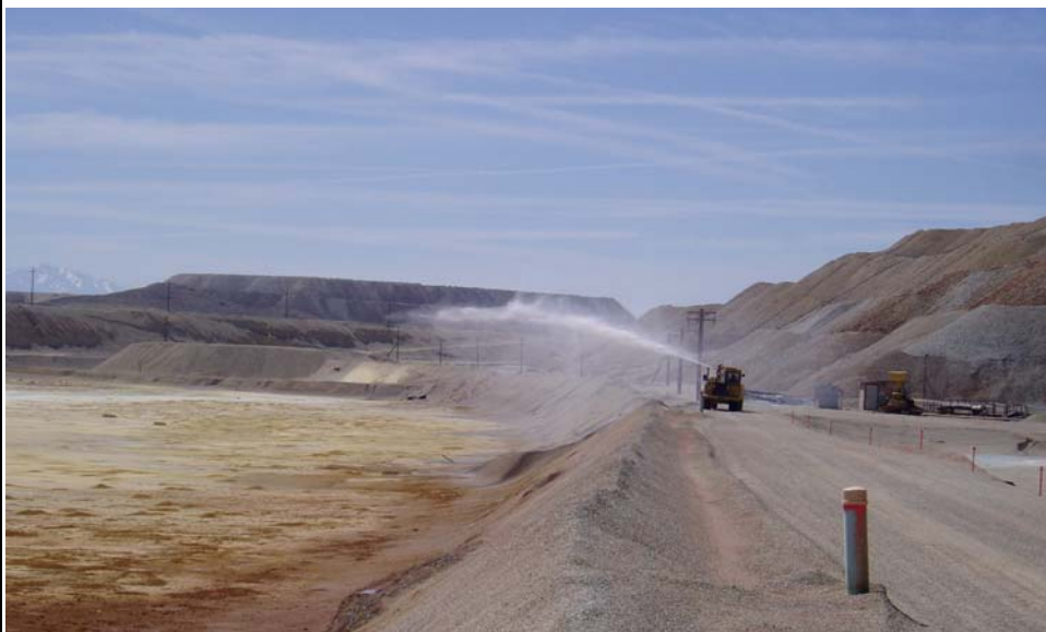
PHOTOGRAPH 16.: Application of soil sealant along west edge of North Evaporation Pond, covering dark reddish material, Area S13. (Facing South-southeast)
