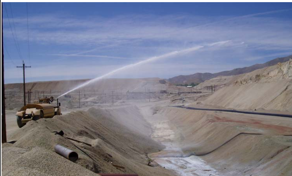
PHOTOGRAPH 19.: Application of soil sealant along west toe of road R12, Area R2. (Facing South)
