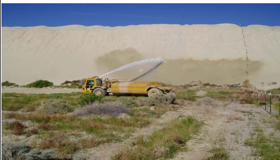
PHOTOGRAPH 18.: Application of soil sealant along the northern face of the Sulfide Tailings, Area S11. (Facing West)
