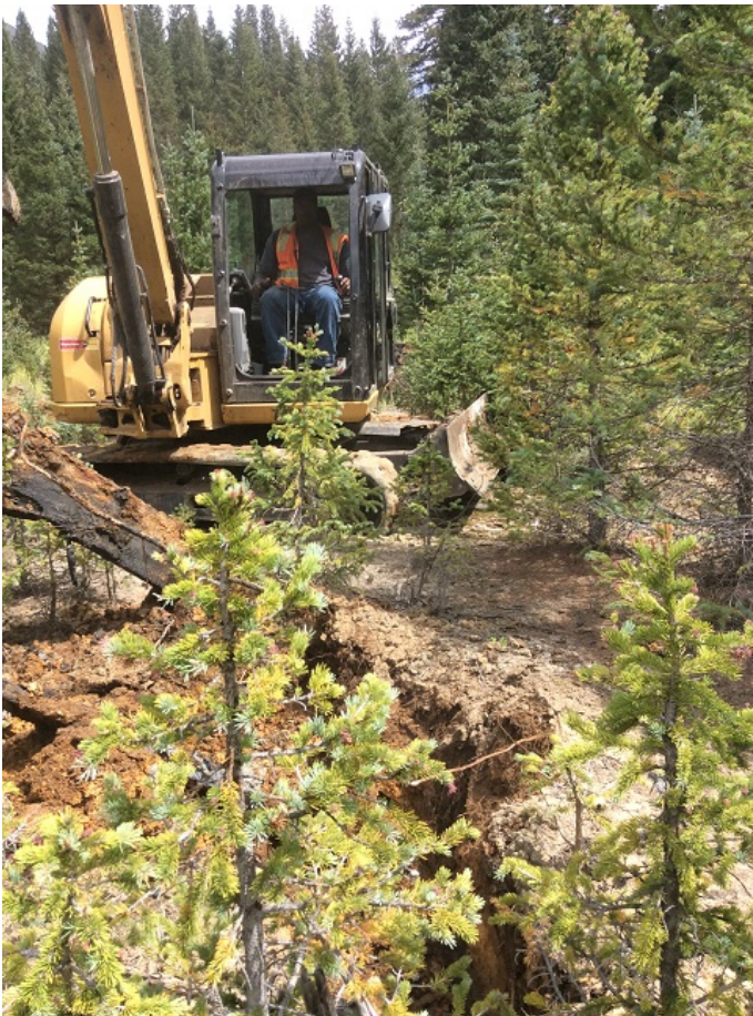
Excavation up to 6 ft down to the water table in tailings.
