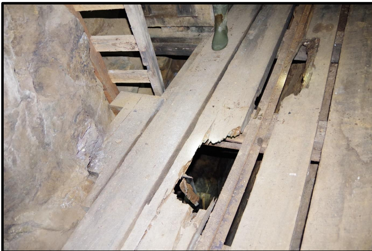
Photo 17: Daylight Winze with rotten wood cover
