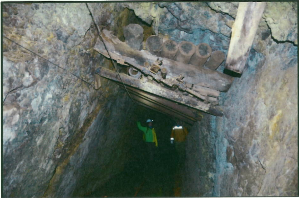
Photo 39: Steel pipe stulls near 32+20; Note pipe cribbing
