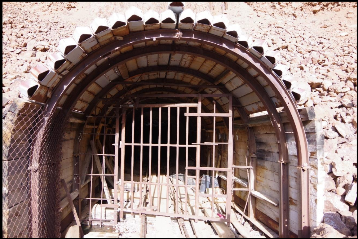
Photo 5: Portal Gate to be replaced
