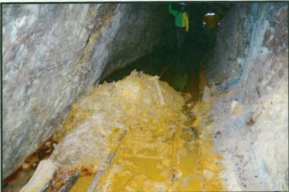
Photo 38: Debris from actively raveling raise near 32+00; Note water backed up behind
