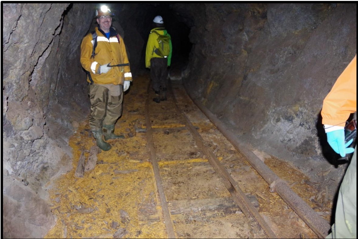
Photo 32: Decayed rail ties near 25+00; Note staining from water
