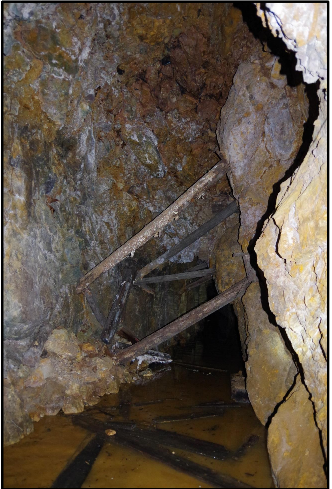
Photo 44: Large loose slabs in hanging wall near 38+10; View is outby
