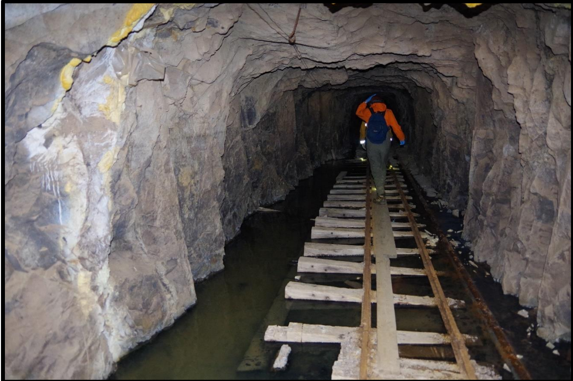
Photo 7: Floating rail ties and poor drainage near 1+00
