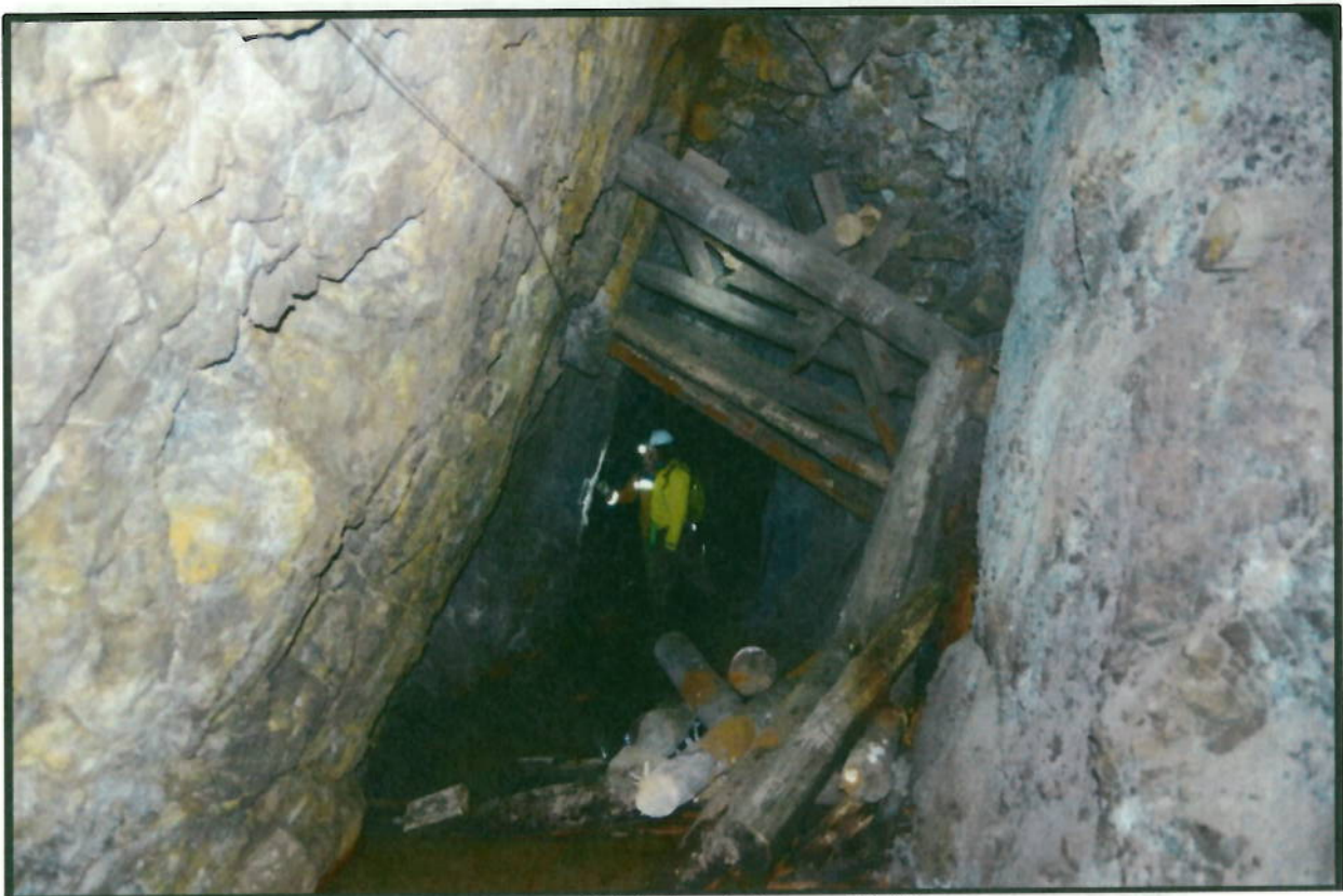
Photo 40: Failed timber stulls near 32+80
