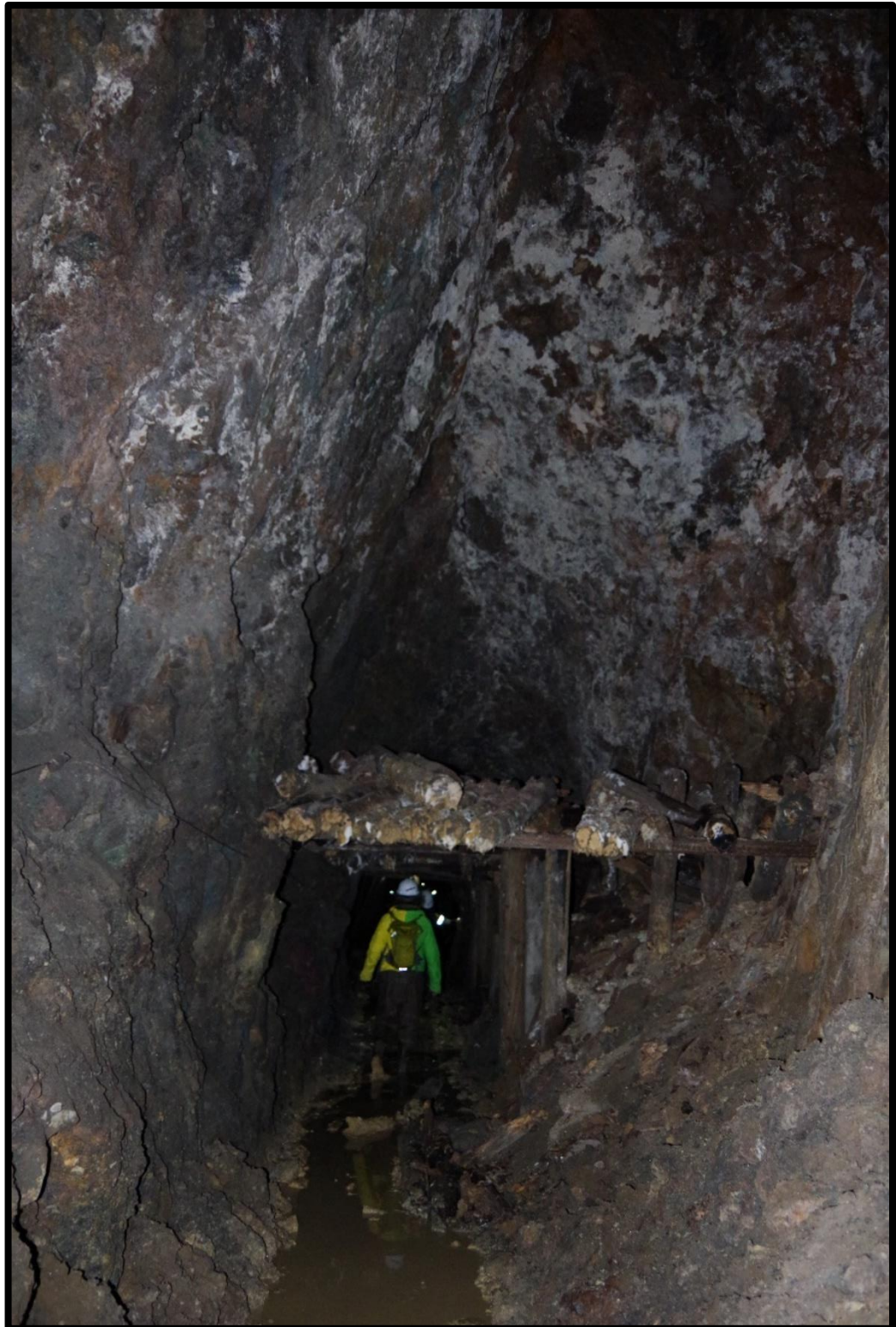
Photo 50: Cathedral near 43+50; Note loose muck in right rib and rotten timber lagging
