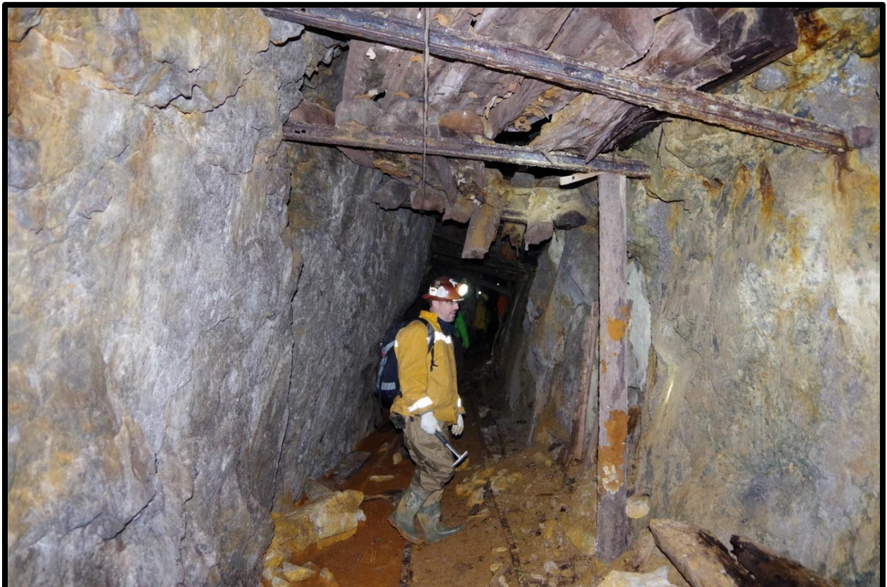
Photo 36: Steel rail stulls with rotten timber lagging 30+50
