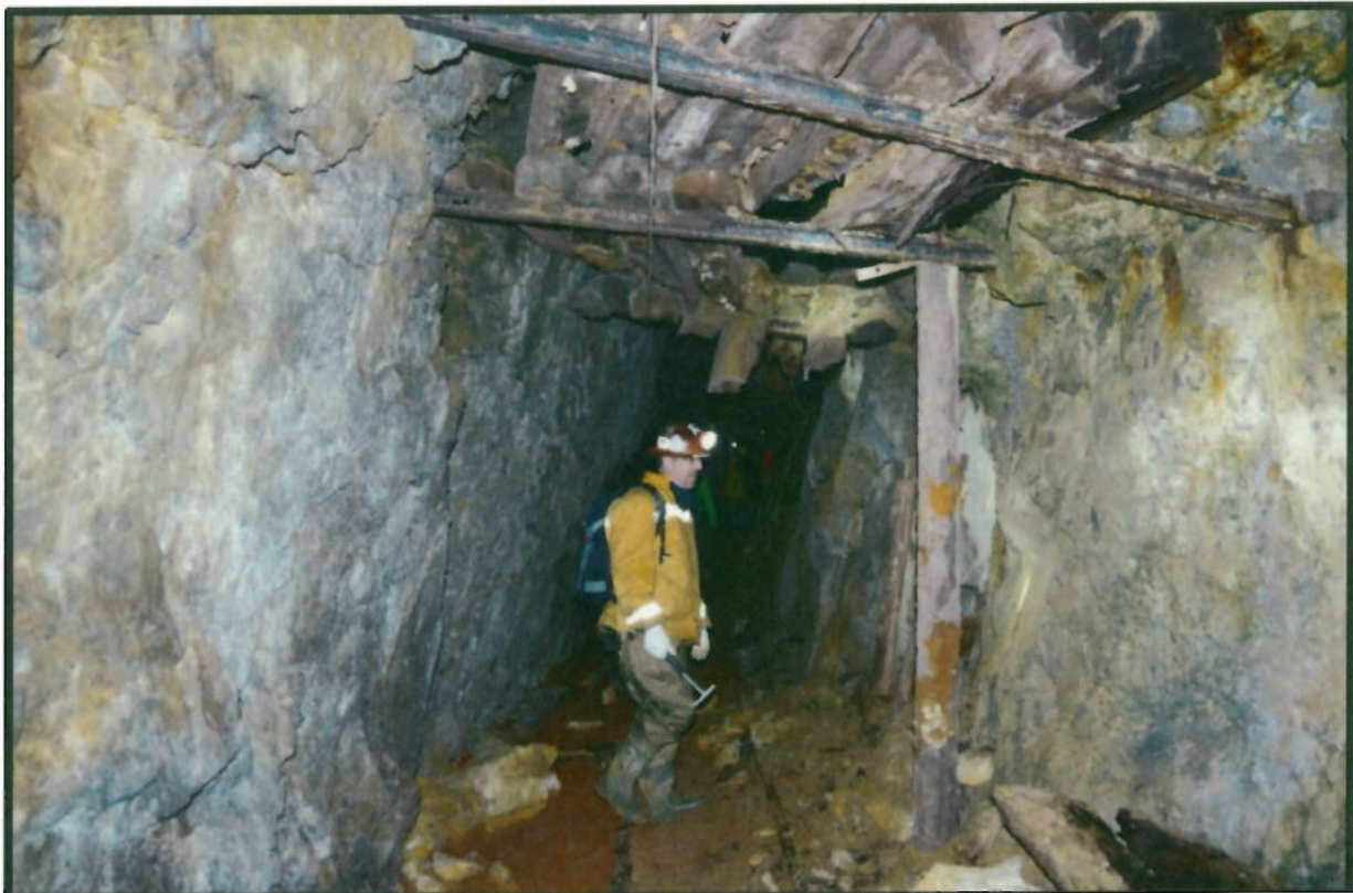
Photo 36: Steel rail stulls with rotten timber lagging 30+50
