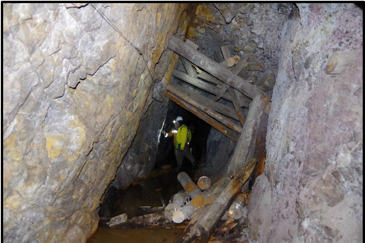
Photo 40: Failed timber stulls near 32+80
