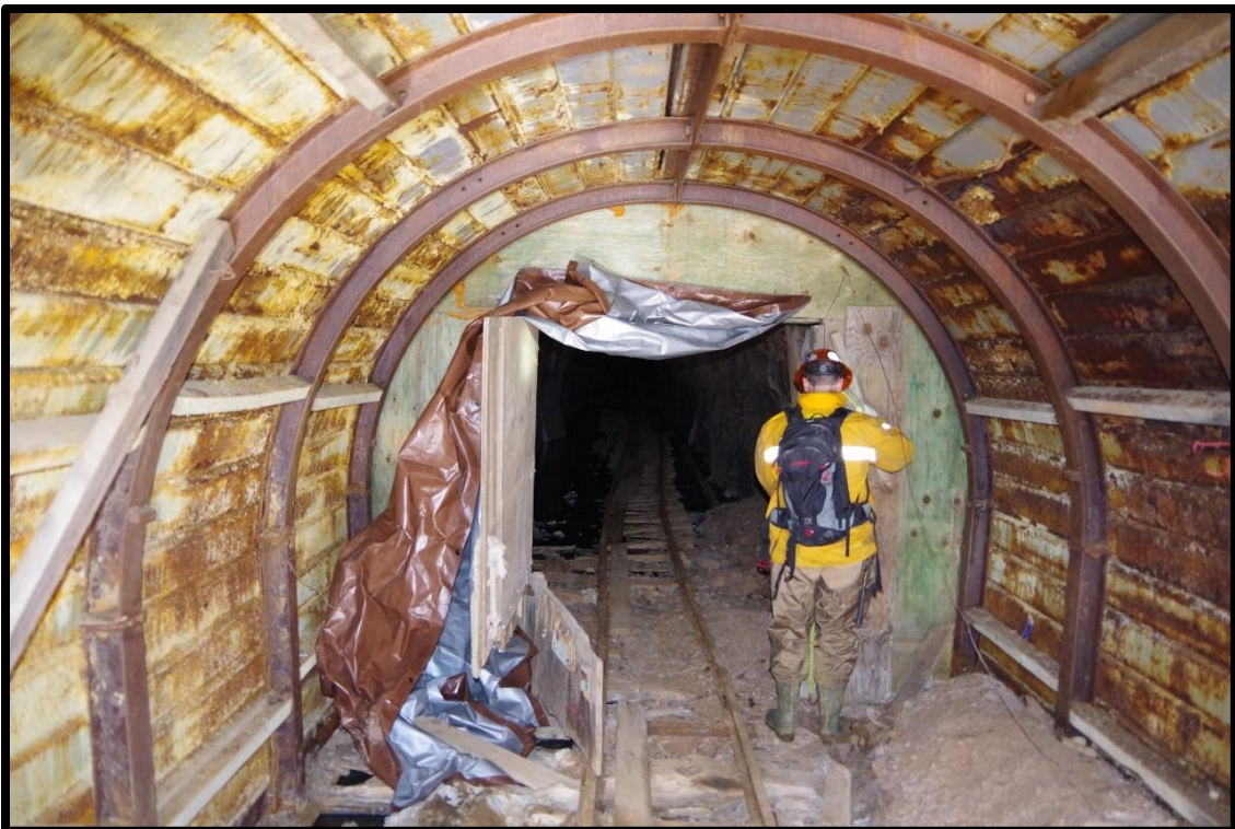
Photo 6: First Air Door to be replaced
