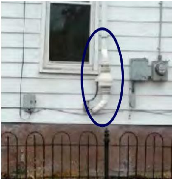
Vapor mitigation system installed on the outside of a house.
