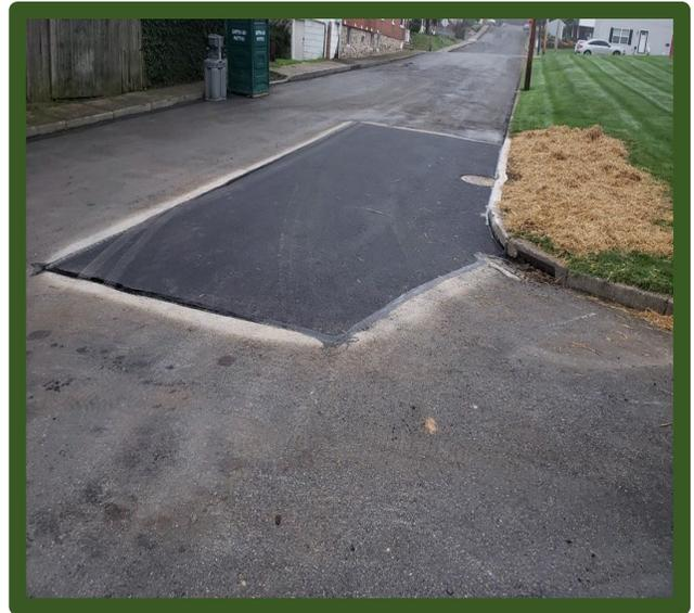
*These photos show the final asphalt, top soil, curb repair after installation. The manhole cover for the oil/water separator can also be seen in these photos.*
