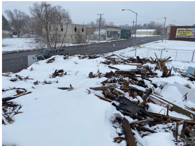
PHOTO 5- Roofing debris contains asbestos
