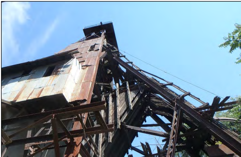
Structure 01: Wood frame contained within steel frame; facing 40 degrees; (Frame P7210149; 07/21/2020)
