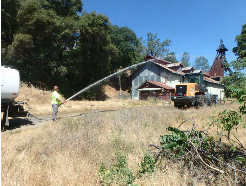
Water application to the staging area prior to grubbing. Facing 290 degrees (Frame P6020003; 06/02/2021)
