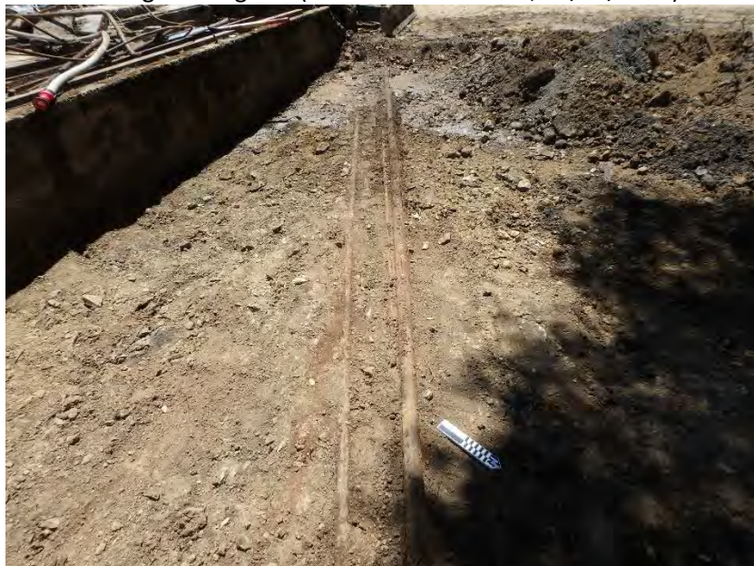
Feature 57: Set of two two-inch metal pipes and two one-inch metal pipes; facing 154 degrees (Photo No. P6140243; 06/14/2021)
