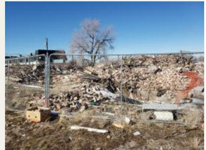
Description: Debris pile of the former Broadway Hotel. Temporary fencing has been placed to deter trespassing but has been inadequate. Debris and friable asbestos containing materials are open to the air and environment. Facing north to showcase extent of debris pile and proximity to public walkways.
