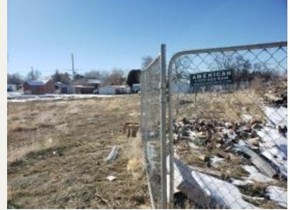
Description: Debris pile of the former Broadway Hotel. Temporary fencing has been placed to deter trespassing but has been inadequate. Debris and friable asbestos containing materials are open to the air and environment. Facing south to showcase extent of debris pile.
