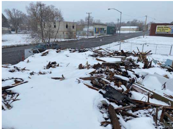
PHOTO 5- Roofing debris contains asbestos
