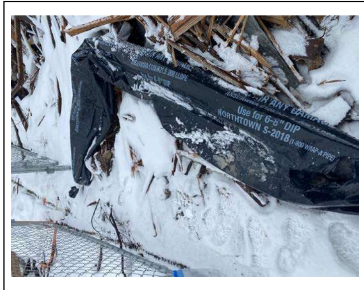
PHOTO 4- Thermal System Insulation "Aircell" debris contains asbestos (wrapped in plastic sheeting)
