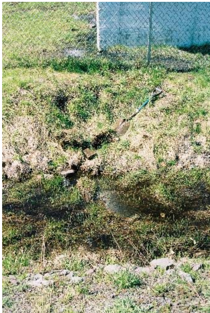
Photograph 14: 5/17/06 Looking northerly at the ditch and base for the southwestern above ground gas storage tank from Franklin Street. Note the discolored surface around the tank base, ponded water, and erosion channels toward the ditch. The base of the shovel is near the test hole in photographs 12 and 13. Photo by J. Chrestensen
