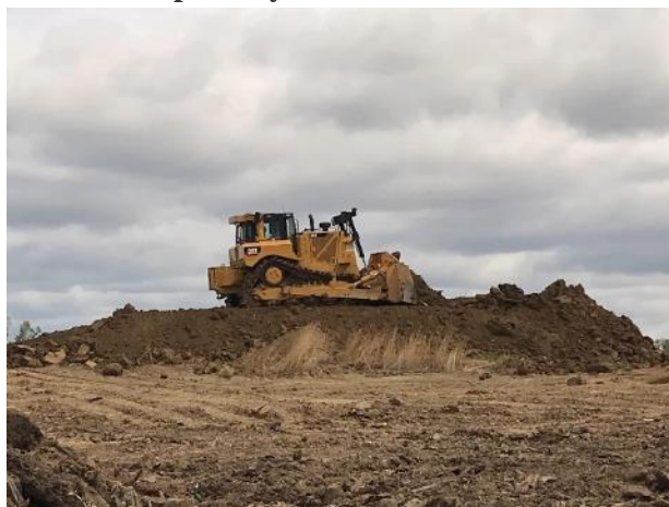
Stockpiling of Back-fill Material
