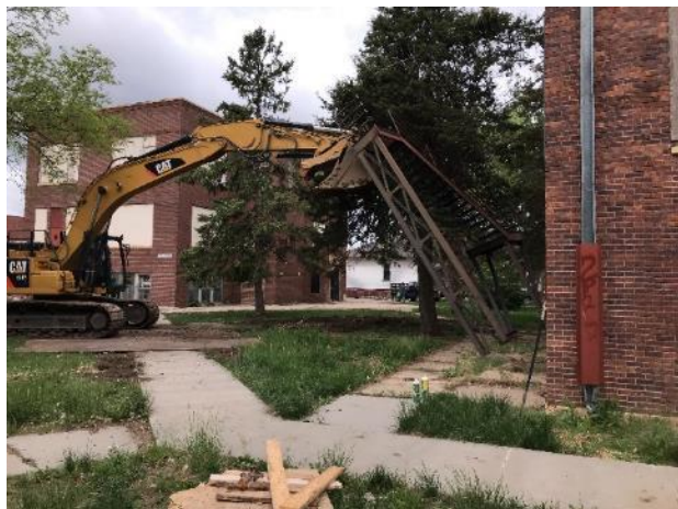
Removal of Exterior Stairs on St. Joseph
