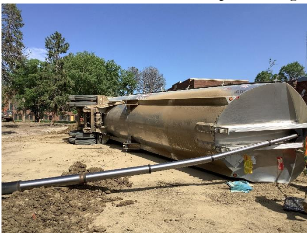
Truck is tipped over due to concrete giving way
