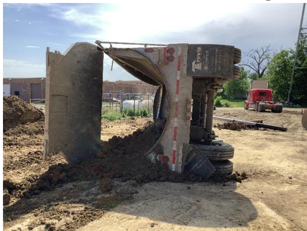
Truck tipped over while unloading backfill
